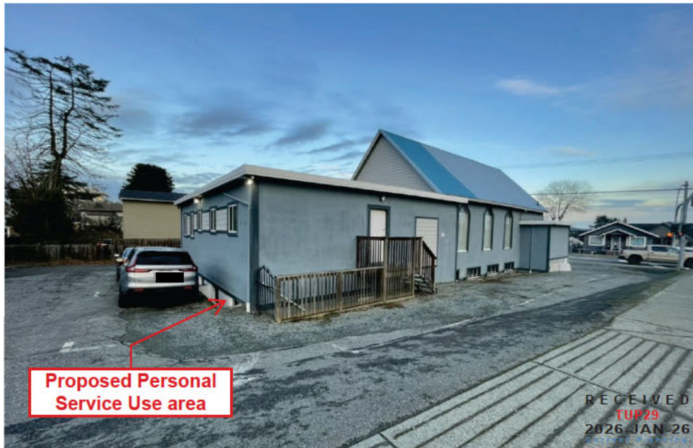
View from Milton Street looking towards Victoria Road
