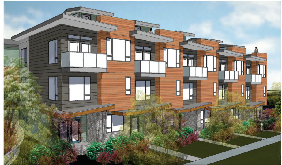
BUILDING 4 FROM DEPARTURE BAY ROAD
