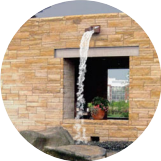
Wall scupper: water discharges from stormwater detention/retention chamber under parking through scupper in retaining wall to ringarden below.
