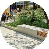
Concrete seawall: seawalls are integrated into the concrete planters at the entrance ramp and stairs to the building.
