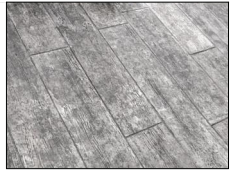
① STAMPED CONCRETE, PAVILION WALKWAY
