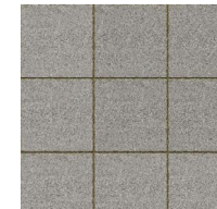
Courtyard Walkway 0.6m x 0.6m Concrete Pavers
