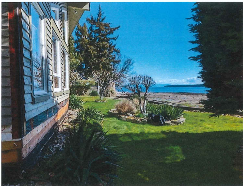
Photograph 1. April 9, 2024. View south – north along the east (oceanfront) side of the house.
