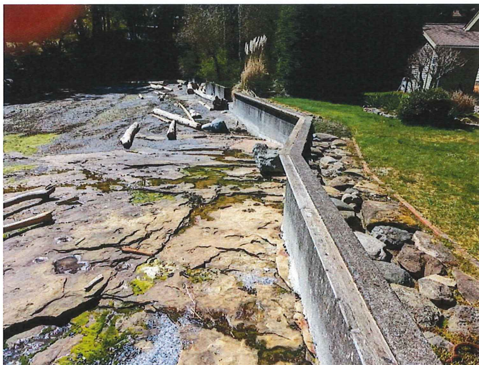
Photograph 4. View north – south along seawall forming natural boundary.
