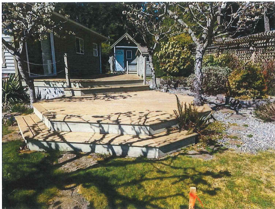
Photograph 5. View of wood deck, ornamental cherry trees and landscaping along the north side of the house.
