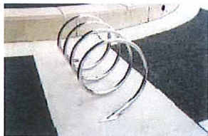
COBRA BGA TO BNG RACK, SURFACE MOUNT PER MANUFACTURER'S SPECS
