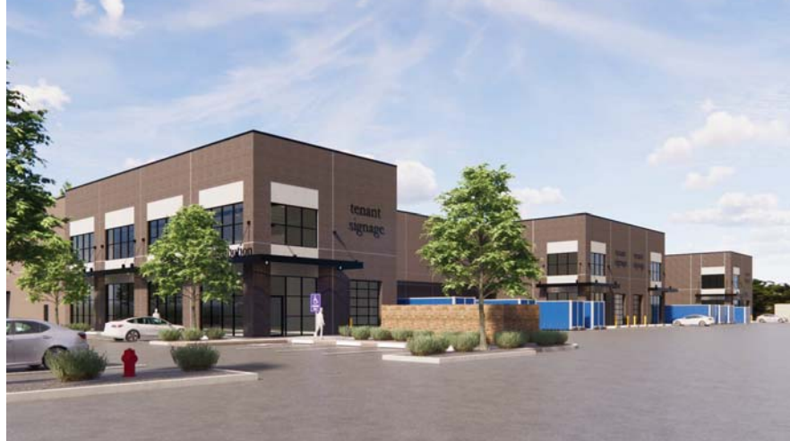
BUILDING 3 - NORTHWEST ELEVATION
