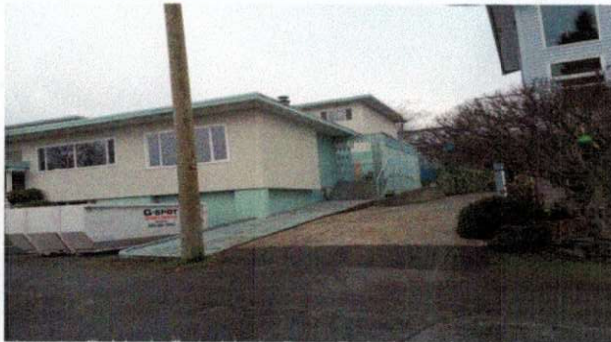
NORTH SIDE PRIOR TO BUILDING PERMIT
