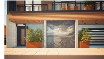
Robson Street - Detail View (Gas Meter Screen)
