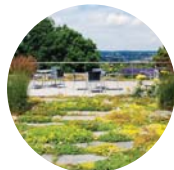
15 Greenroof with roof deck patio
