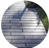
09 Arbour walk permeable concrete unit pavers
