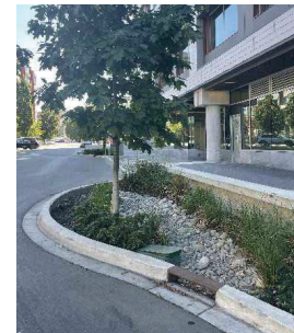
2. Street surface runoff collection into rain garden.
