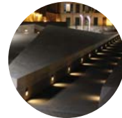
06 Recessed wall lighting
