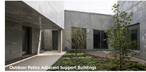
Outdoor Patios Adjacent Support Buildings
