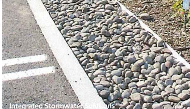
Integrated Stormwater Berms
