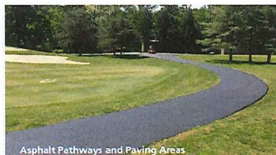
Asphalt Pathways and Paving Areas
