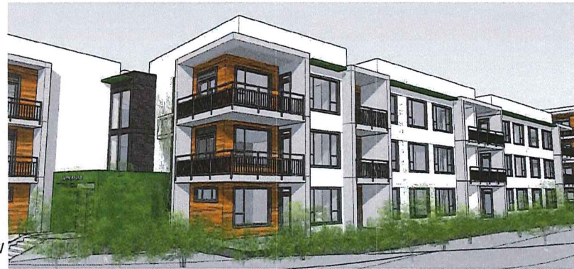
3 SOUTH-WEST CORNER VIEW
