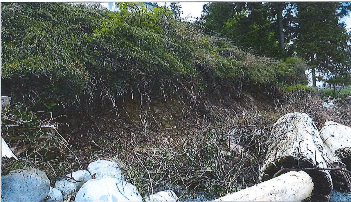
Photo 6. Showing the embankment slope facing north towards the neighbouring property (3500 Chinook Road). Erosion evident at the toe of the slope.
