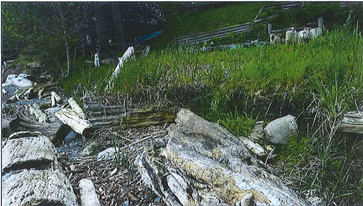
Photo 3. Showing the embankment slope down to the beach vegetated with dune grass. Slope erosion areas evident. The rock rip rap will cover the erosion areas.
