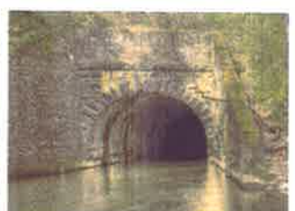
WEST END OF STONE BRIDGE UNDER RAILWAY
