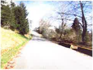
CALEDONIA AVE. LOOKING NORTH
