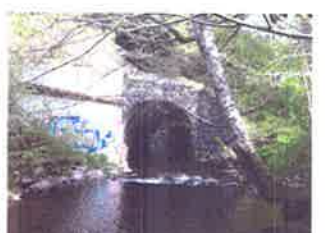
WEST END OF STONE BRIDGE UNDER RAILWAY
