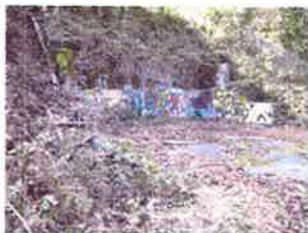
WEST POWER HOUSE EXISTING FOUNDATIONS (STAVE PIPE TO RIGHT)
