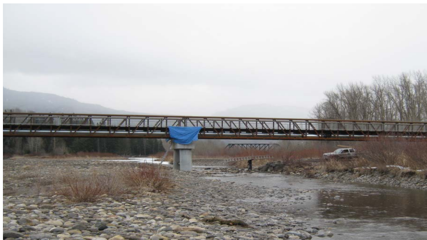
Figure 4.3 – Example of a Steel Truss Bridge with Integral Guardrails (Elk River Crossing near Sparwood)
