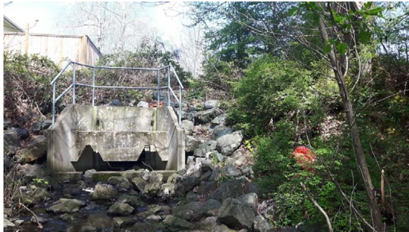
Figure 3.5 – Storm Sewer Headwall looking north
