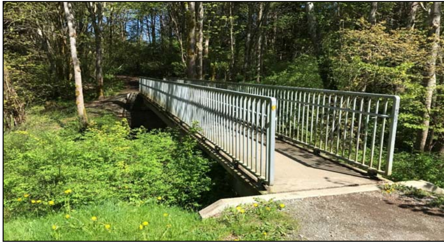
Figure 4.1 – Example of Concrete Box Girders and Galvanized Railing (Cat Stream Crossing near Park Avenue in Nanaimo)
