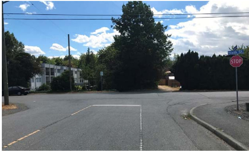
Figure 3.2 – Sixth Street/Georgia Avenue intersection looking south towards 10m wide road ROW
