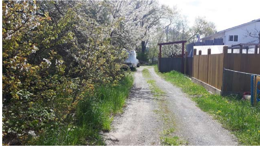
Figure 3.3 – 10m wide road allowance looking south
