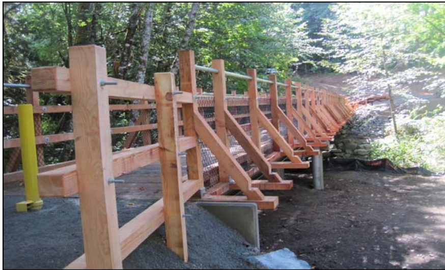
Figure 4.2 – Example of Steel Girders and Timber Guardrails (Bings Creek Crossing near Duncan)
