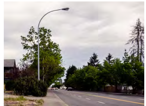
Typical cobra head light standard on Terminal Nicol.
