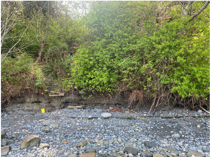
Photo 3.29 Undercutting with a low erosion scarp along shoreline.
