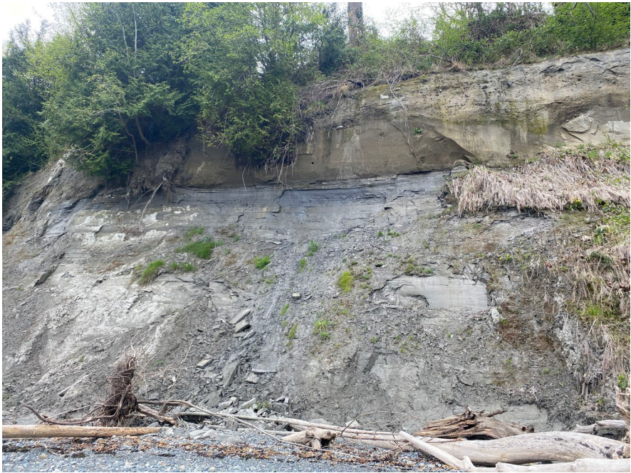
Photo 3.6 Bluff scarp with evidence of recently deposited sediment at the toe of the bluff.
