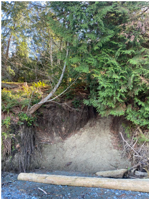
Photo 3.7 Small slope failure resulting in additional erodible sediment at the toe of the bluff.
