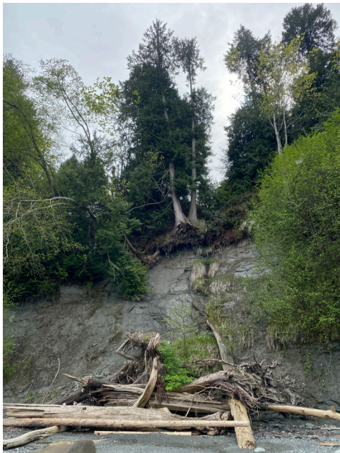
Photo 3.10 Location of slope failure along bluff.
