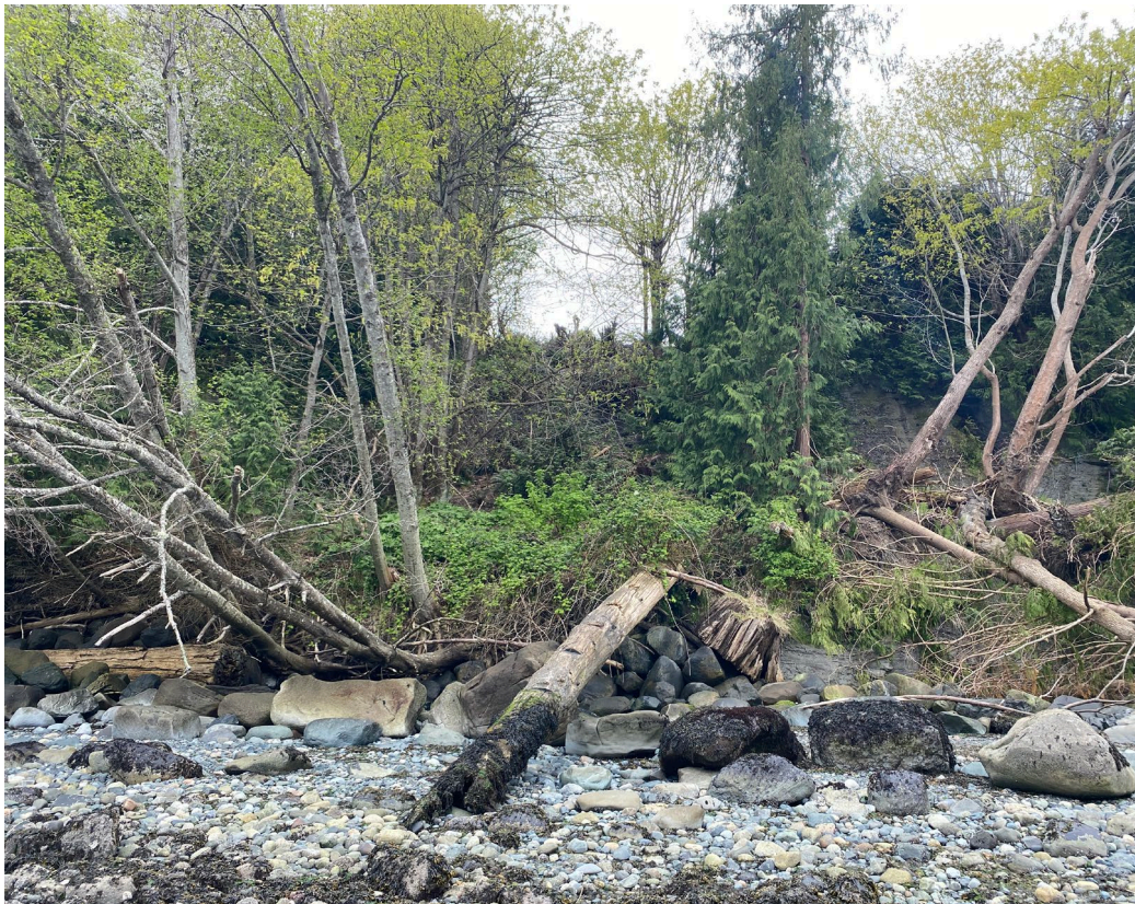
Photo 3.13 Location of slope failure along bluff.
