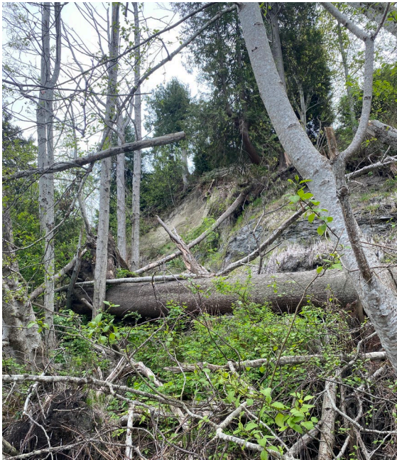
Photo 3.11 Location of slope failure along bluff.
