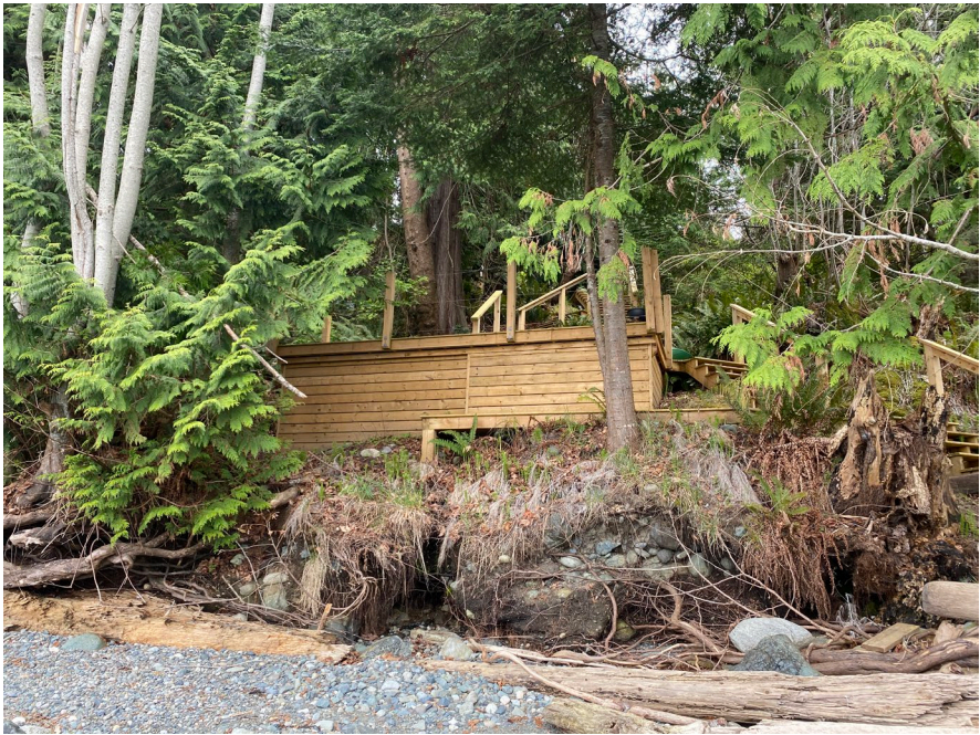
Photo 3.3 Undercutting and exposed tree roots along shoreline.
