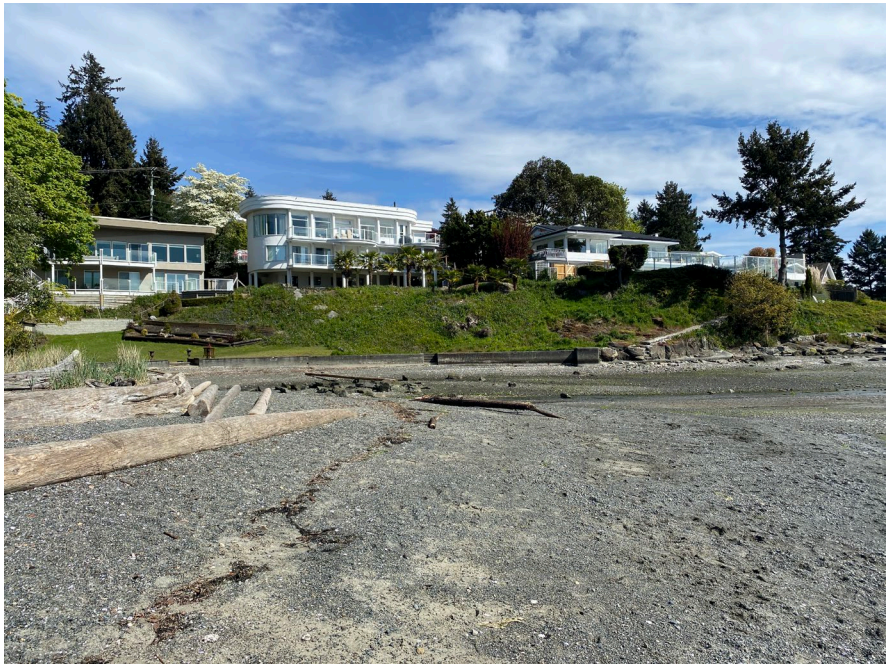
Photo 3.16 Departure Bay bluff next to Departure Creek. The toe of the bluff is protected by a low seawall (left) and bedrock outcrops (right).
