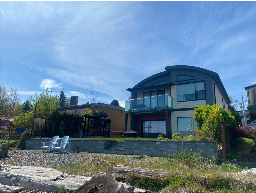
Photo 3.39 Example of low walls as shoreline protection along Randle Road.
