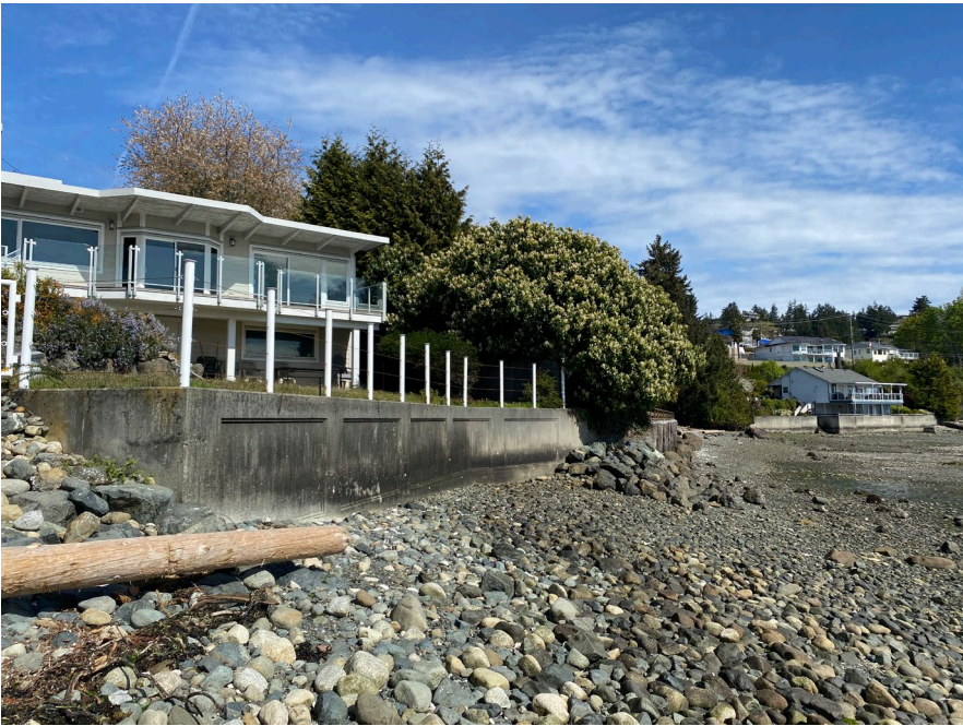
Photo 3.23 Examples of shoreline protection along the lower lying west end of the Departure Bay focus area.
