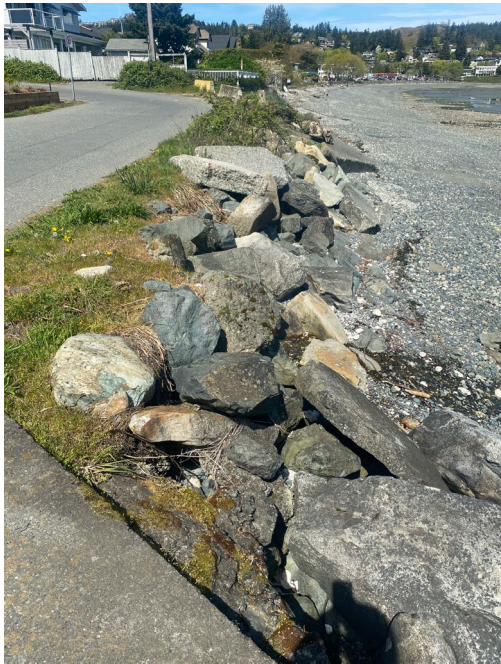
Photo 3.41 Riprap along Battersea Road.
