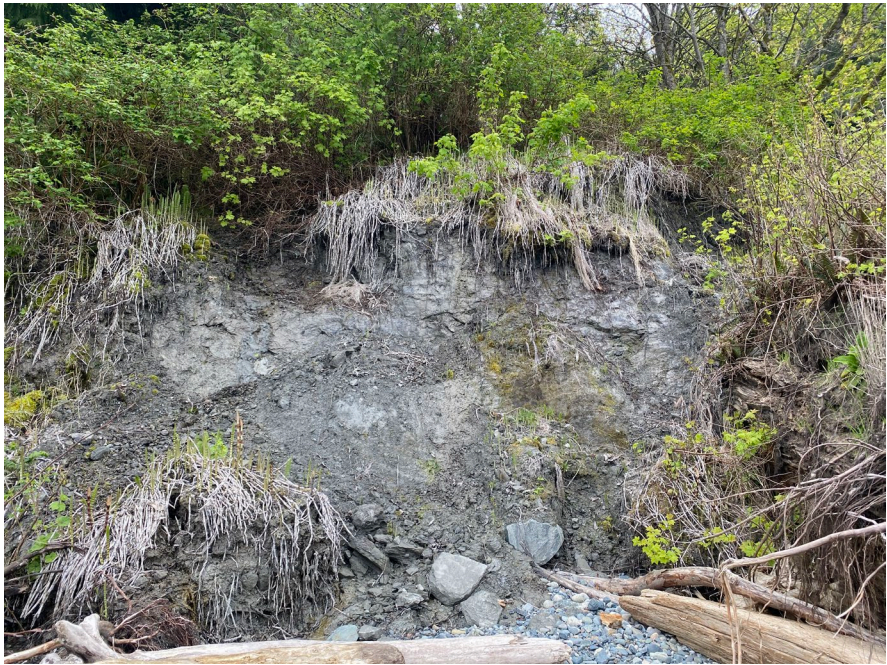
Photo 3.4 Erosion scarp along shoreline.
