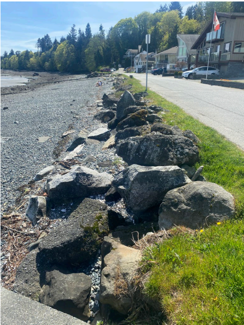
Photo 3.42 Riprap along Battersea Road.
