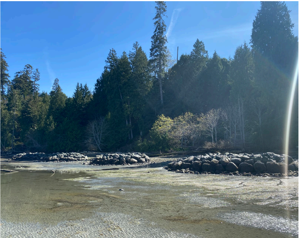
Photo 3.15 RDN interceptor protection east of Oar Road.
