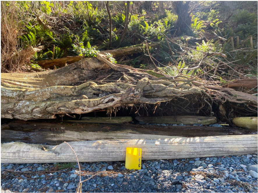
Photo 3.2 Undercutting and exposed tree roots along shoreline.
