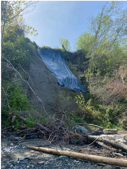
Photo 3.32 Exposed bluff scarp with evidence of slope failure at toe of the bluff.
