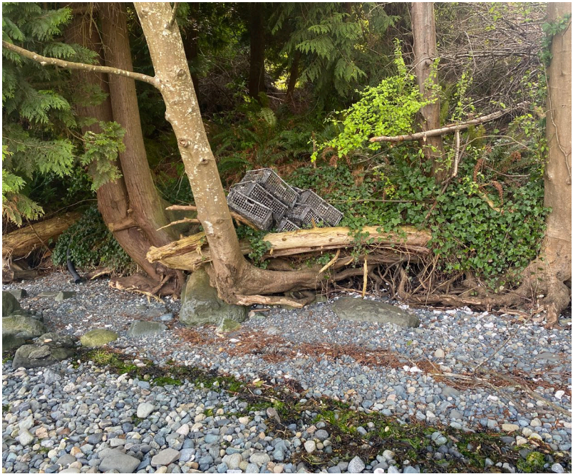
Photo 3.28 Undercutting and exposed tree roots along shoreline.
