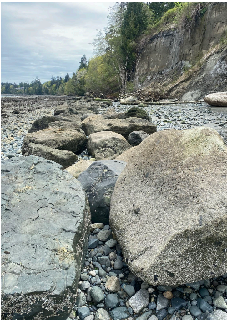
Photo 3.14 Suspected remnants of old riprap placement. Bluff has receded behind line of boulders.
