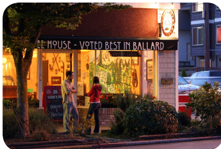
Well designed exterior lighting improves the streetscape.
