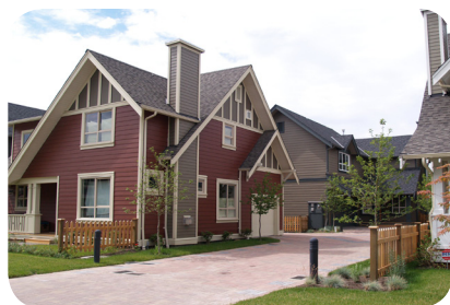
Shared driveways with permeable surfaces.
