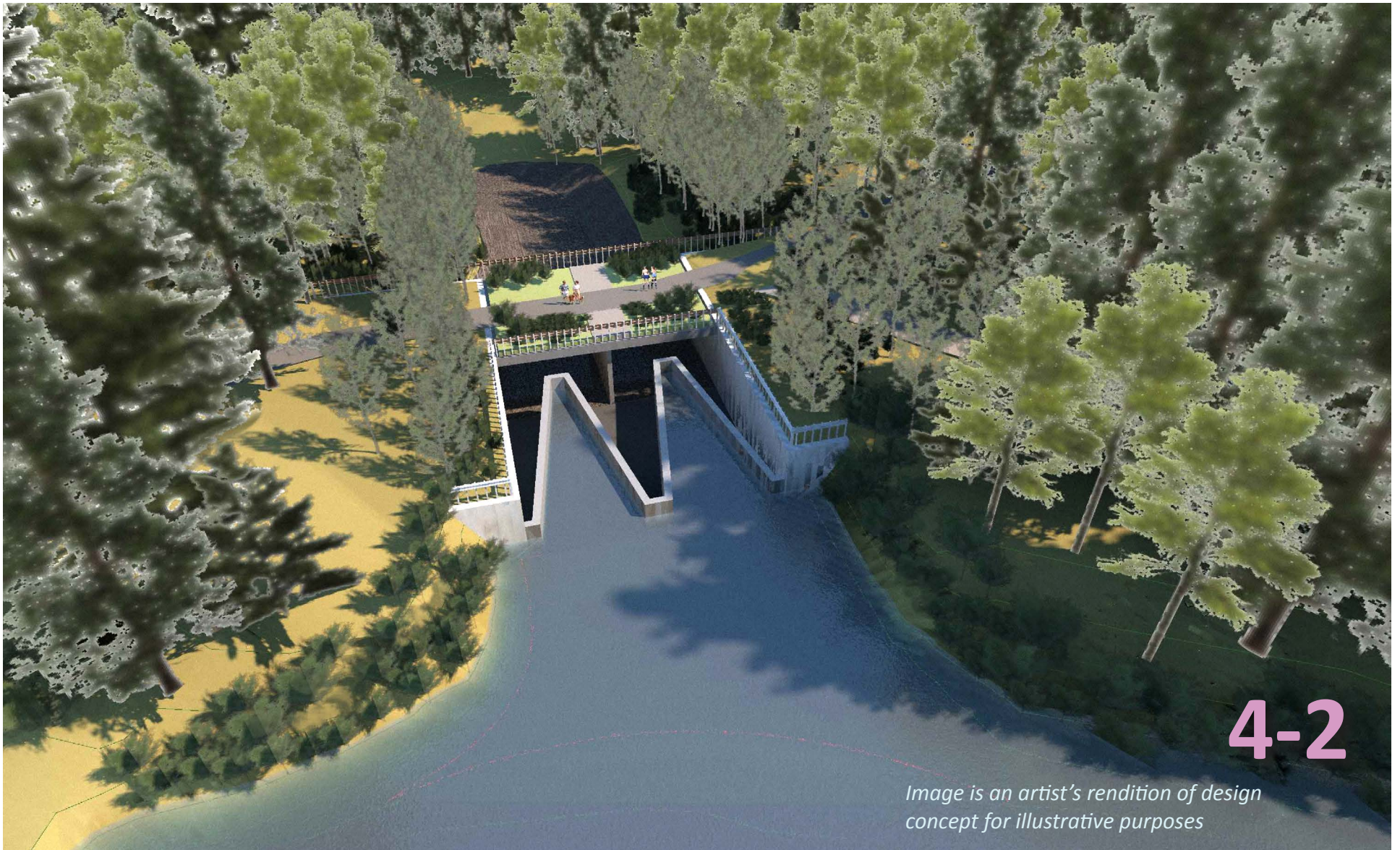
Auxiliary Spillway to Harewood Creek - Labyrinth /Box Culvert Open Channel Option 2 Aerial view from the north
