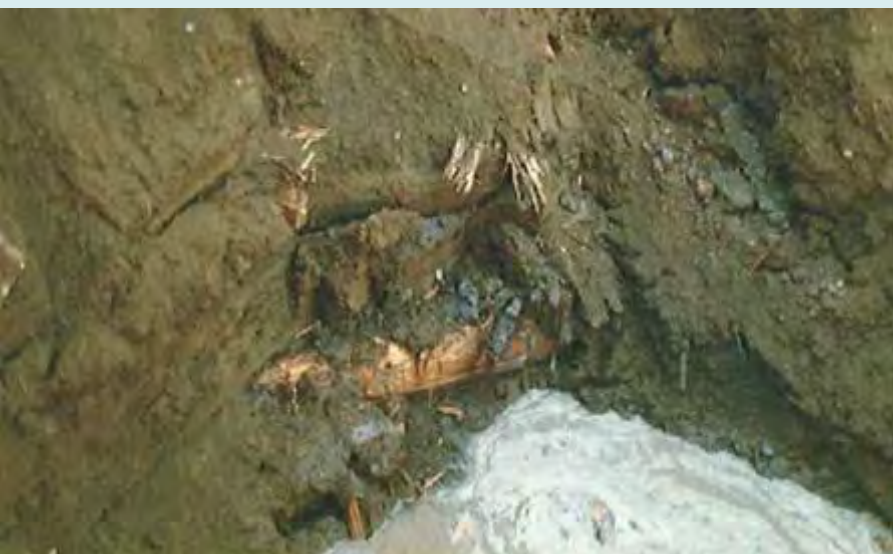
Original log crib exposed – logs were still intact
