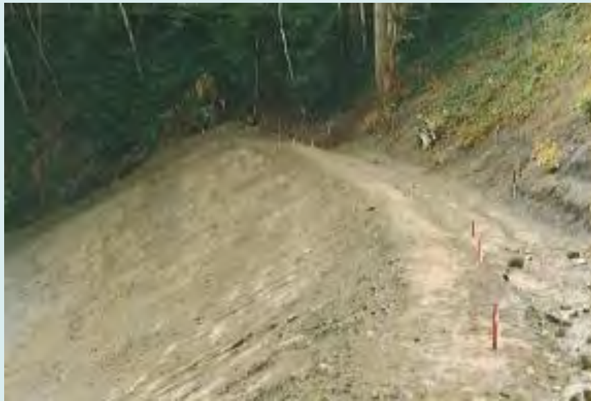
Stabilizing berm viewed from left abutment
