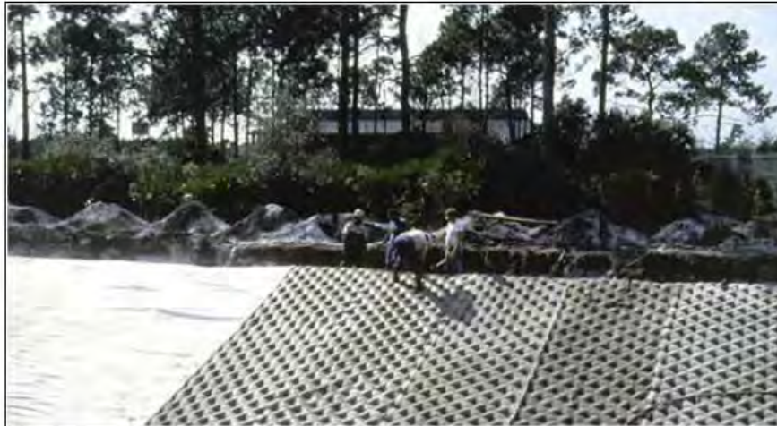
Figure 7.—Fabric forms being filled with fine aggregate concrete. (Courtesy of Donnelly Fabricators.)
