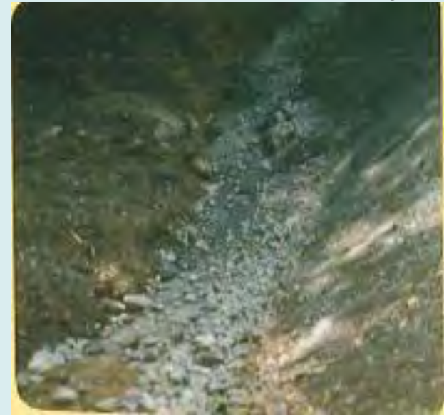
Drain rock toe drain used to pick up embankment seepage
