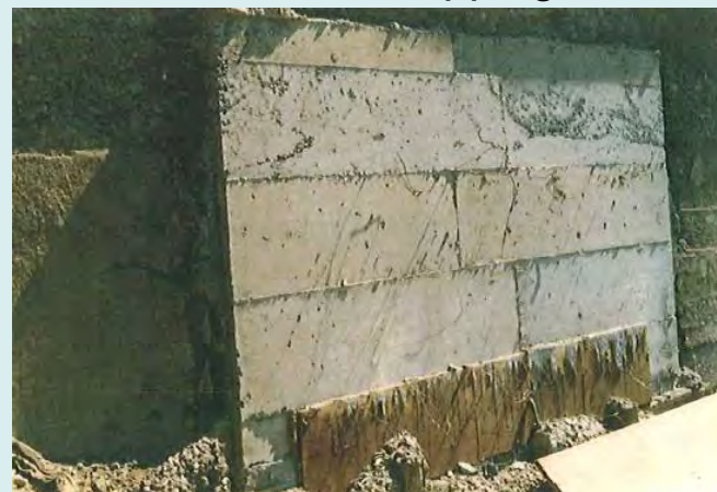
Concrete plug from upstream face after stripping
