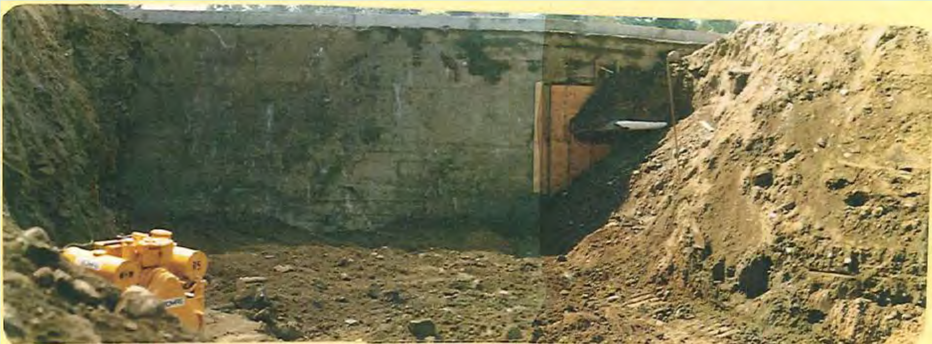
Beginning of fill replacement – note vibratory compaction in left foreground of photograph
