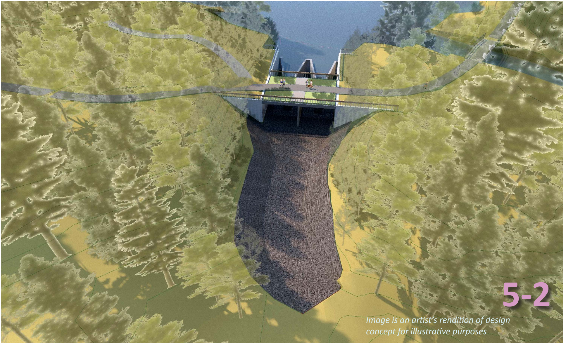
Auxiliary Spillway to Harewood Creek - Labyrinth /Box Culvert Open Channel Option 2 Aerial view from the south
