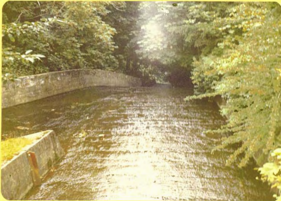
Spillway chute downstream of bridge.
