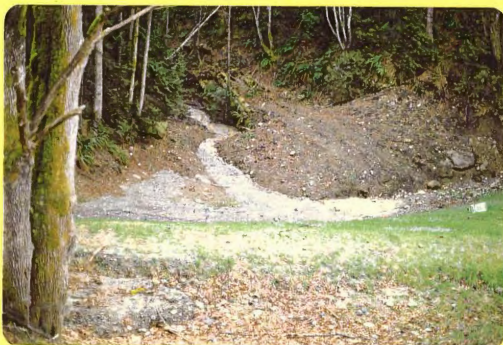
Infilling of toe drain from left abutment sluff.
