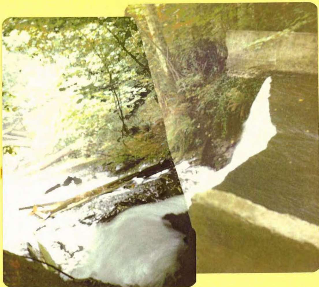
End of spillway chute showing concrete erosion water falls on sound rock.
