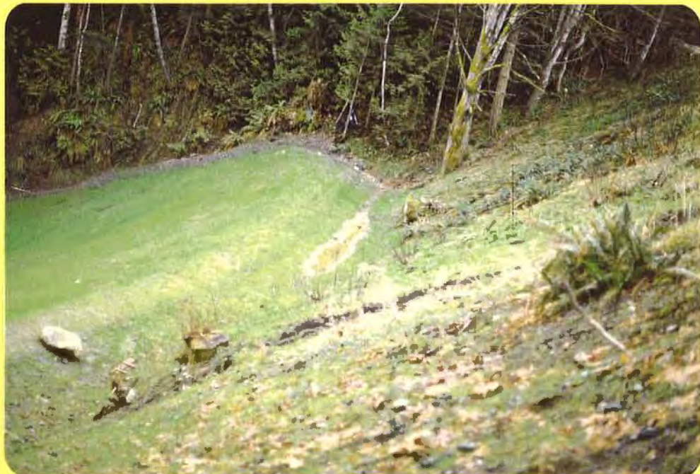
Run-off pooling on filter blanket.
