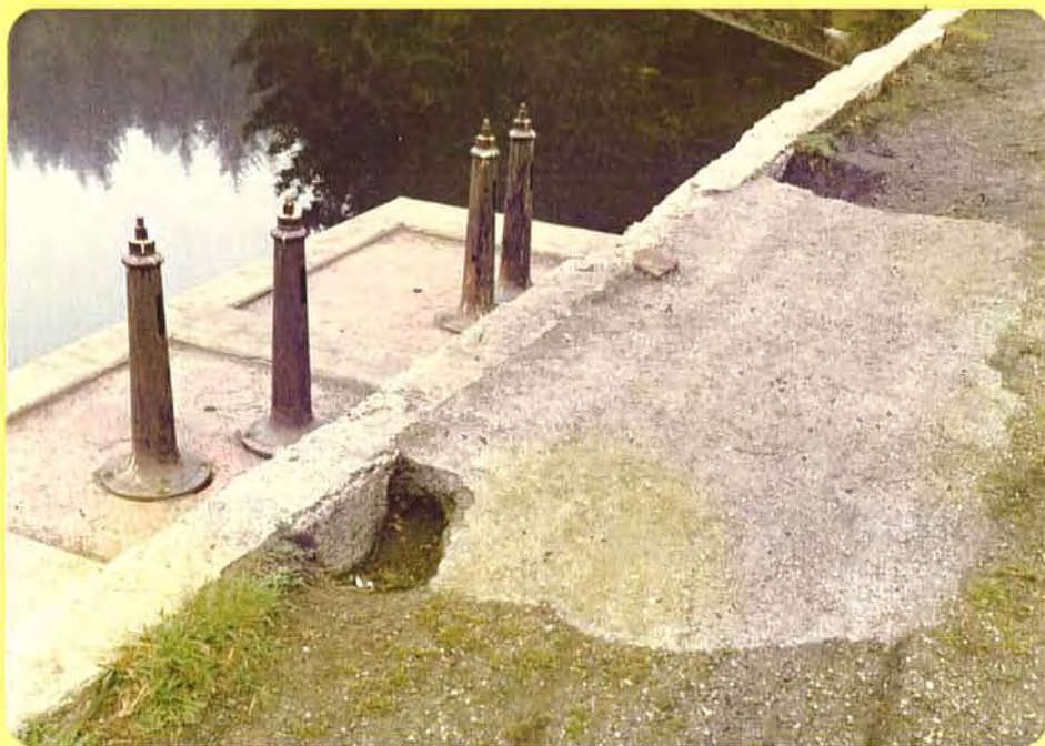
Sluice gates and area where dam crest fill has eroded away.
