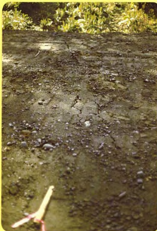
Cracking in berm observed from dam toe.
