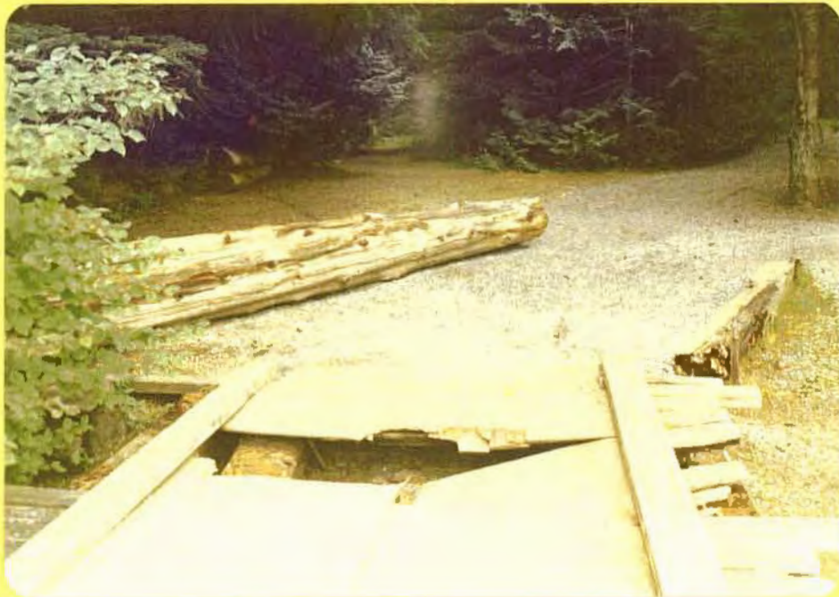
Spillway bridge. Note repairs needed.
