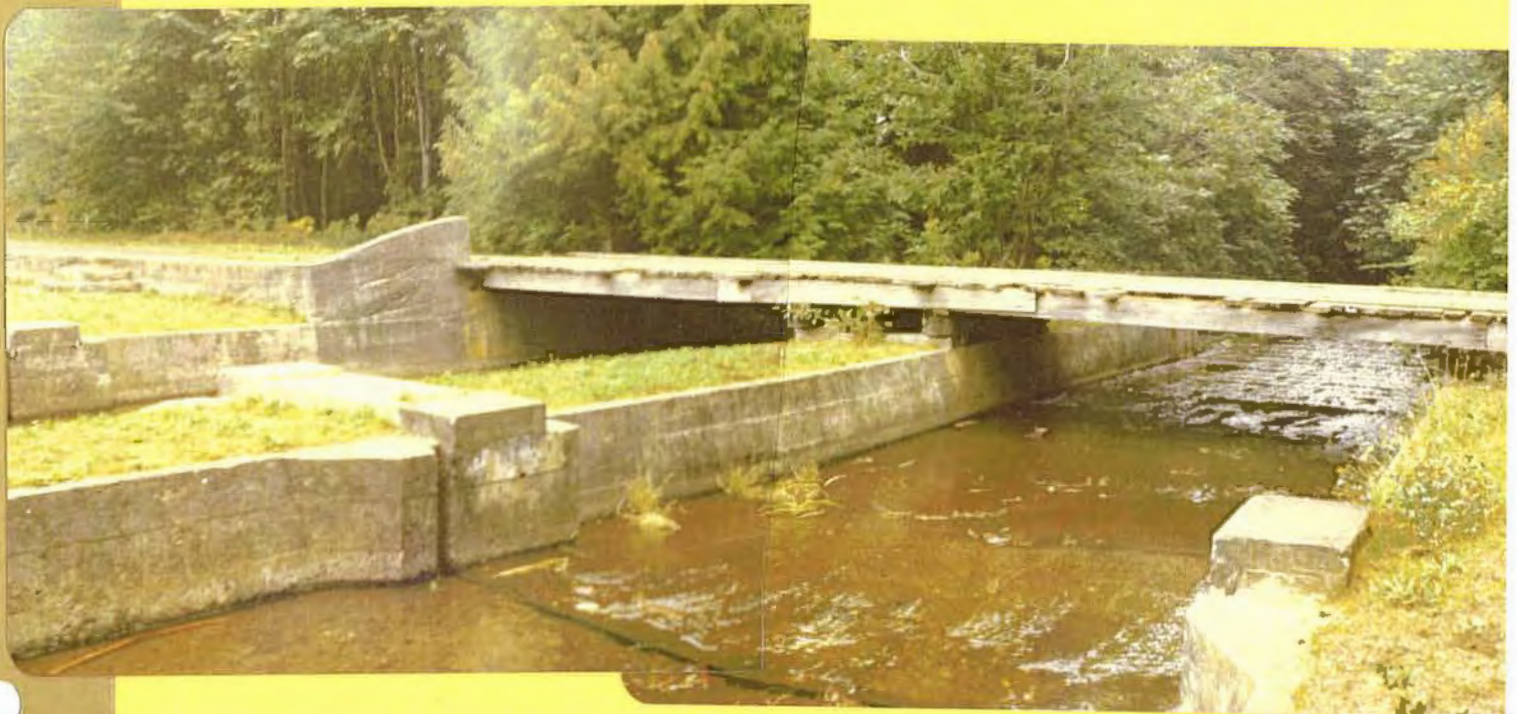
Spillway bridge on Dam centreline.
