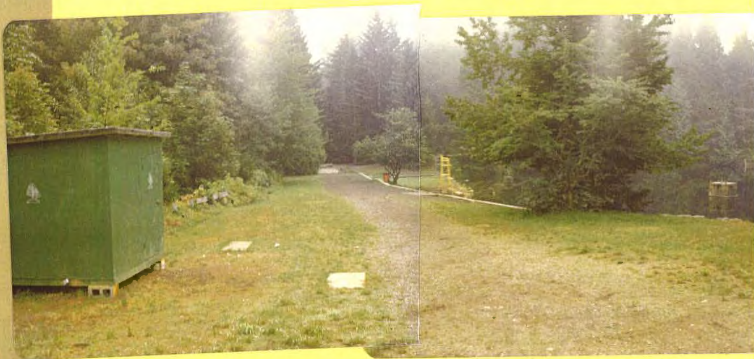
#137 Crest of dam and reservoir. Note heavy growth on downstream face of dam.
