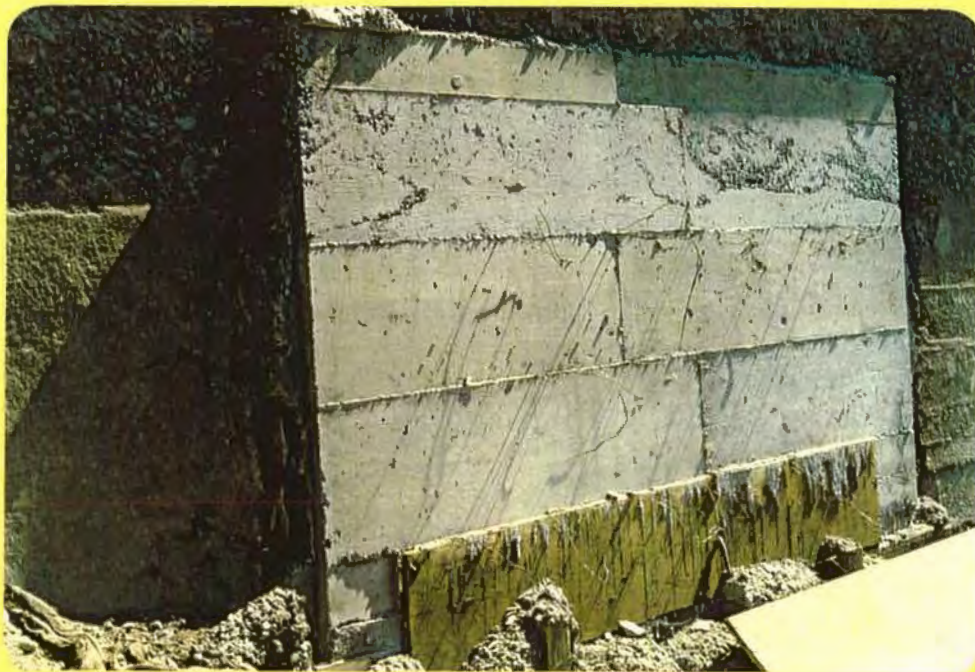
Concrete plug from upstream face after stripping.
