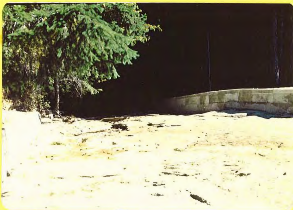
Spillway channel from crest of dam.
