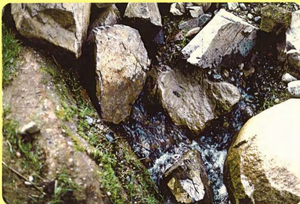
Seepage at downstream toe.
