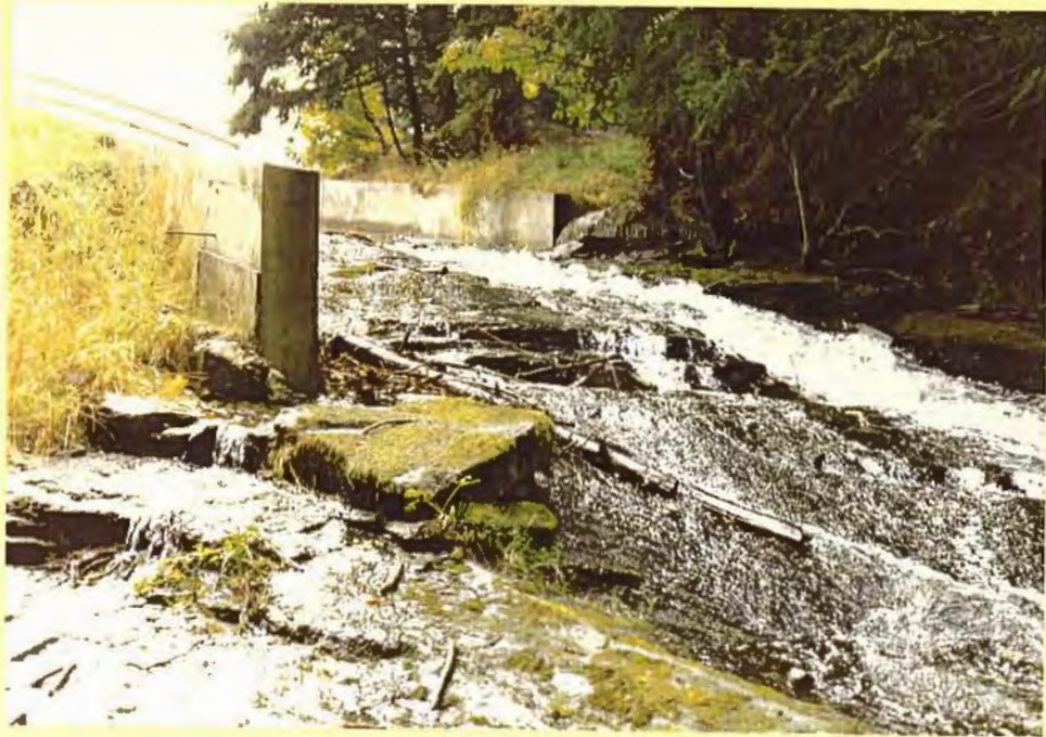
Spillway flowing at right of photo into monitoring weir.
