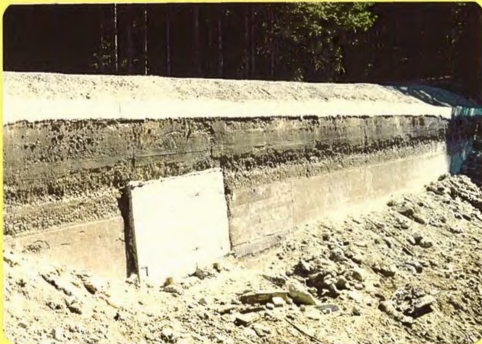
Upstream face of dam showing one foot high concrete wall addition and concrete plug at old outlet area. Note also deterioration of existing concrete.
