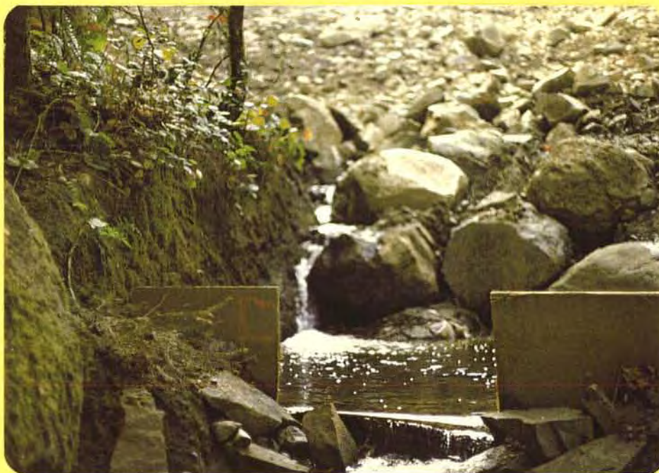
Upstream face of completed renovations. Note concrete plug repairing hole through concrete face.
