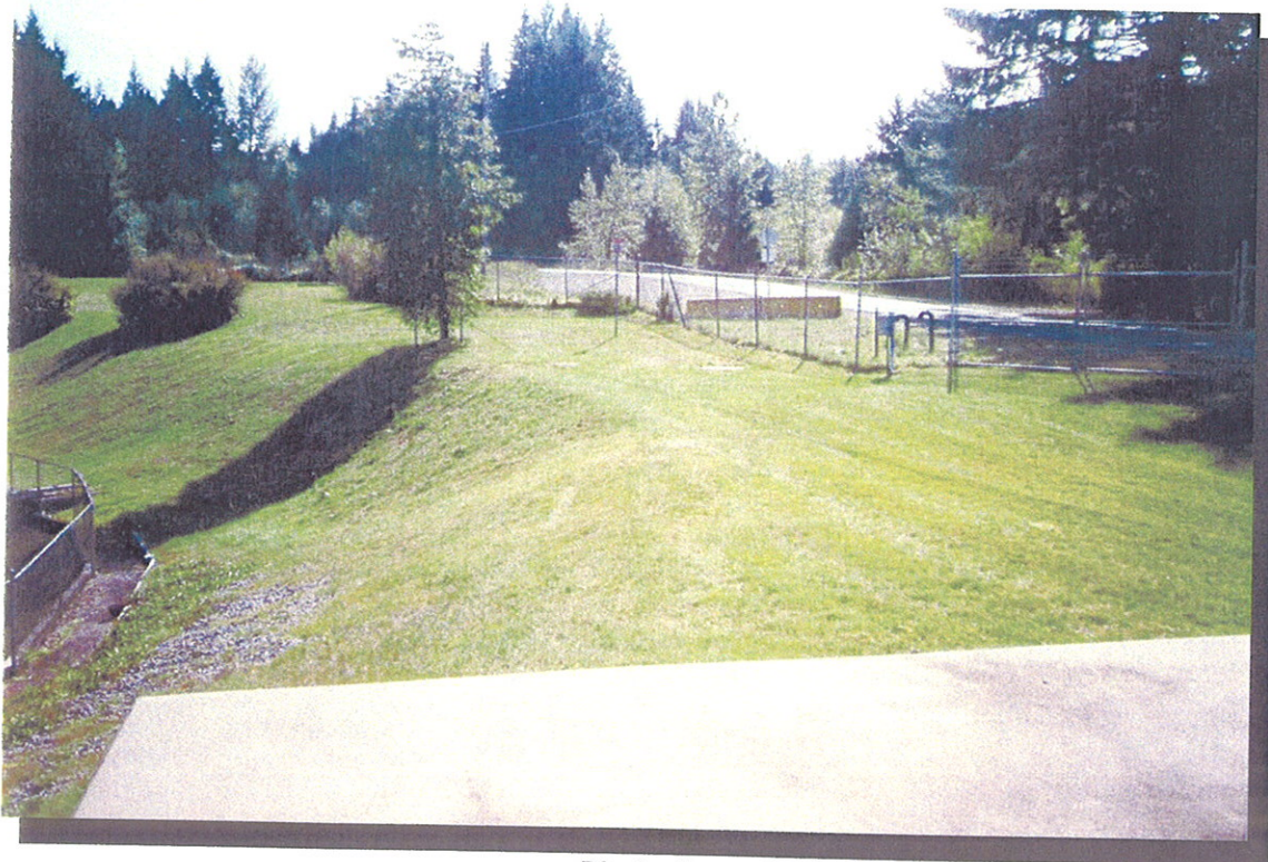
Photo 6 Downstream slope of Upper Chase River Dam, facing south. Structure in foreground is a concrete banker founded on bedrock at approximate location of bedrock ridge encountered in 1998. Edge of Reservoir No. 1 at bottom left corner of photo.
