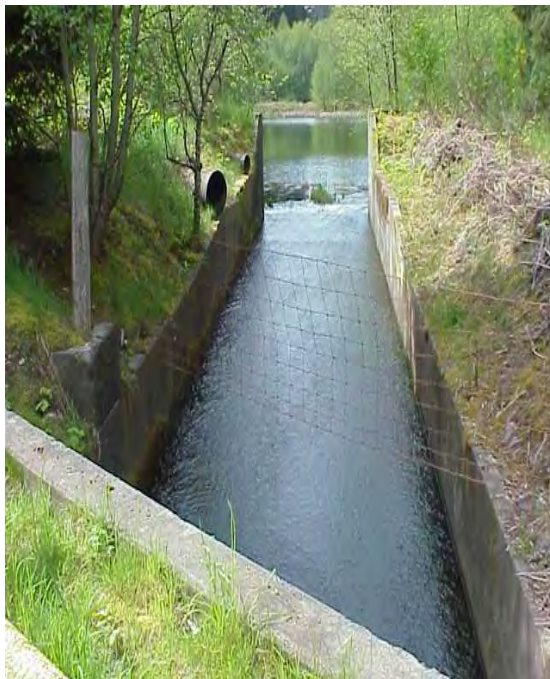
Upper Chase River Dam Spillway
