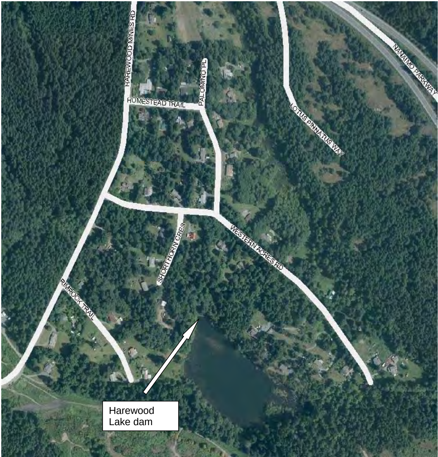
Harewood Lake Dam
