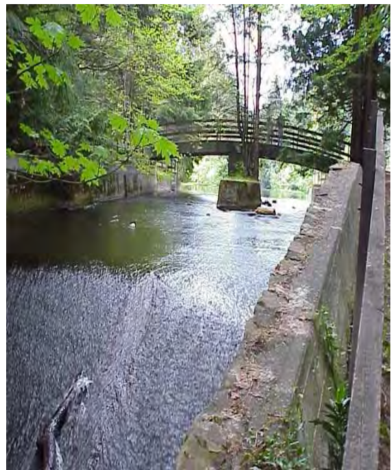
Lower Chase River Dam Spillway
