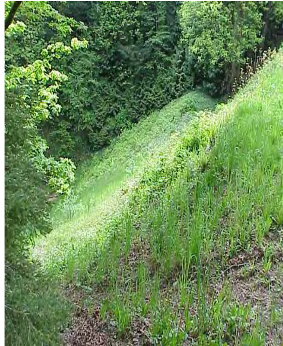
Lower Chase River Dam downstream
