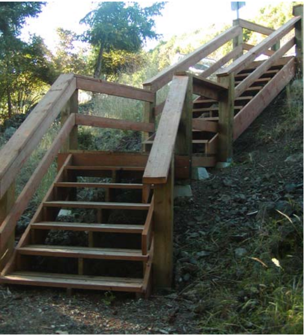
Fillinger Waterfront Park Beach Access stairs.
