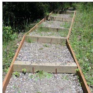
Dirt filled and timber steps like those above have become maintenance concerns and are no longer a park standard.
