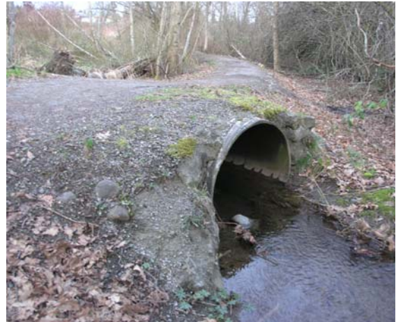
Culvert and headwall at Buttertubs Marsh.
