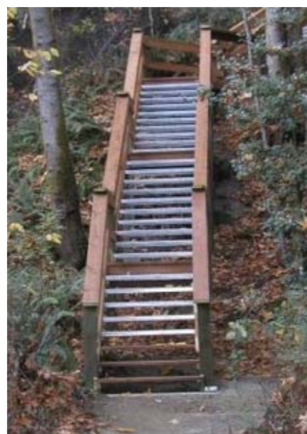
Stairs near Bradley Street. Treads are metal and have great traction.
