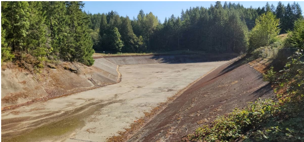
R01 1: Dewatered Reservoir Looking Upstream from the Dam
