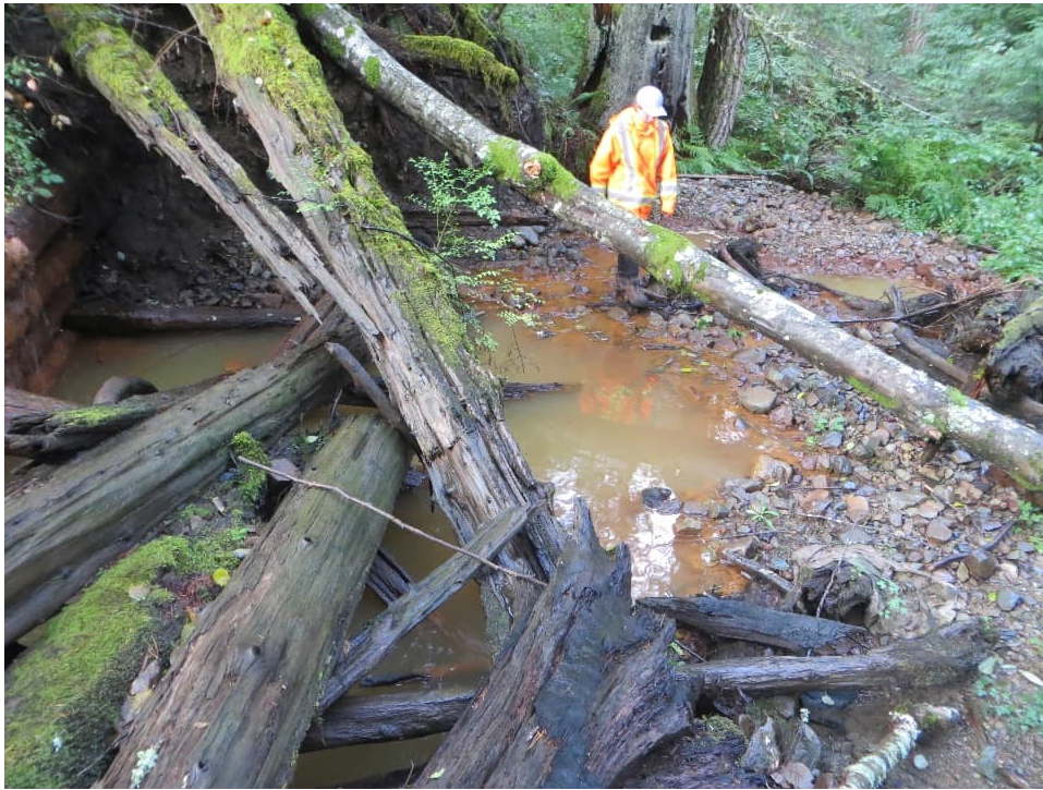
WCL 2: Left Abutment Looking Downstream
