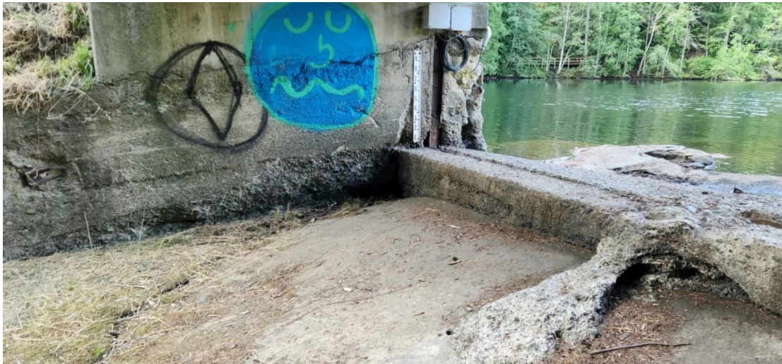
MCR 3: Right Spillway Pier
