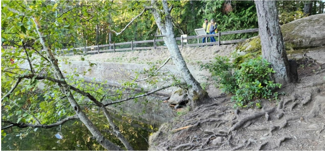
MCR 17: Upstream of Dam Looking Left Abutment
