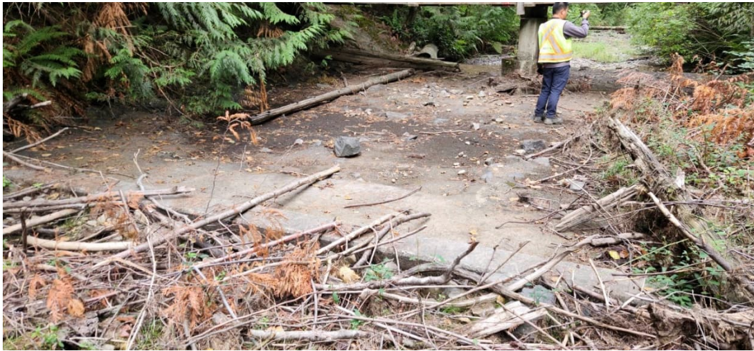
WWL 15: Westwood Lake Outlet Concrete Sill (Outlet Channel)
