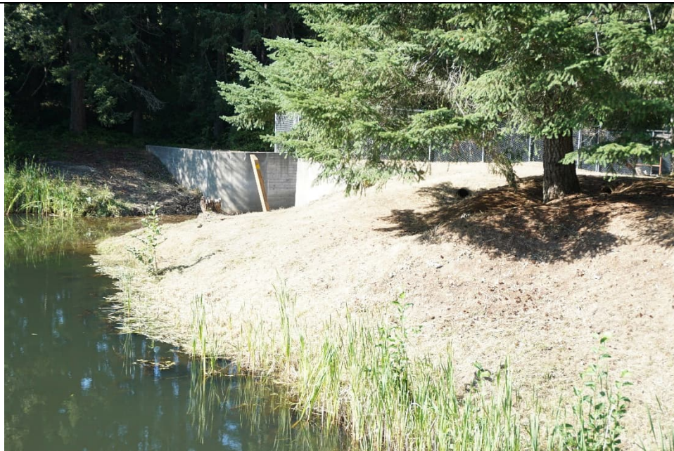
UCR 9: Embankment Dam and Vegetated Shoreline
