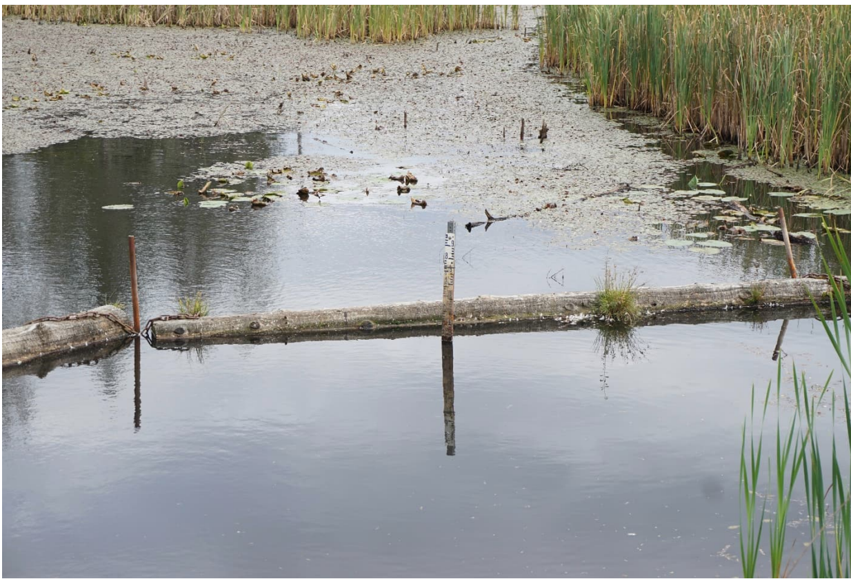
MGC 2: Staff Gauge and Boom Upstream of the Dam
