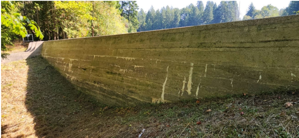
HAW 7: Downstream Side of the Dam
