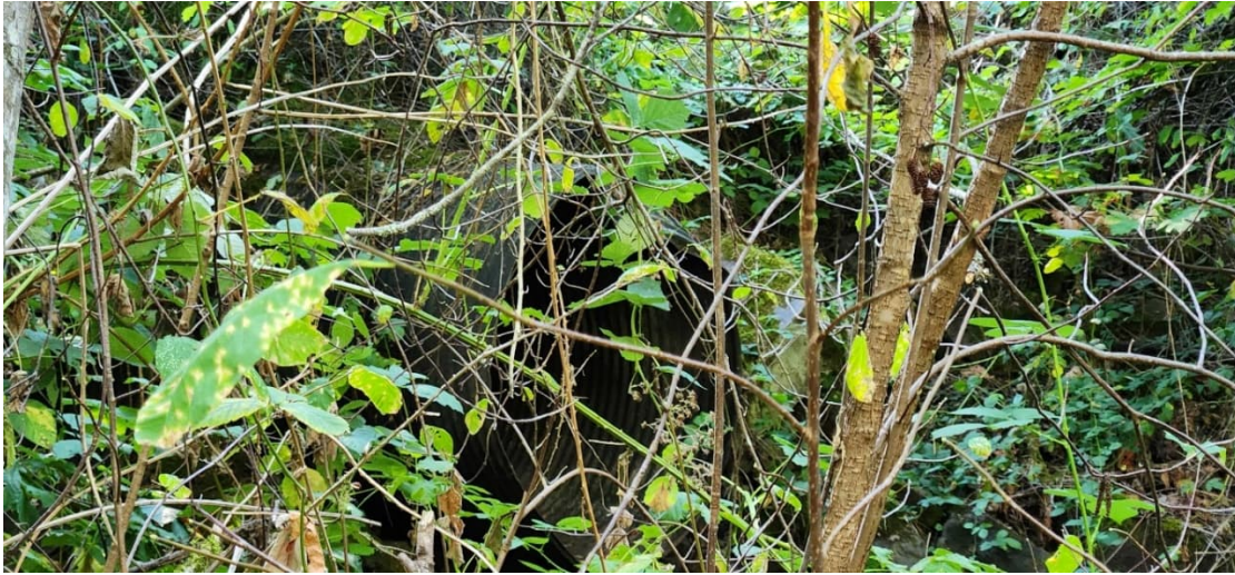
UCR 16: Damage to Left Culvert at Downstream End
