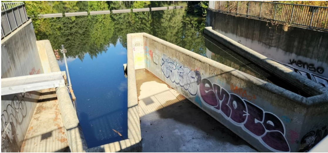
LCR 16: Upstream Side of Auxiliary Spillway Structure and Log Boom Beyond
