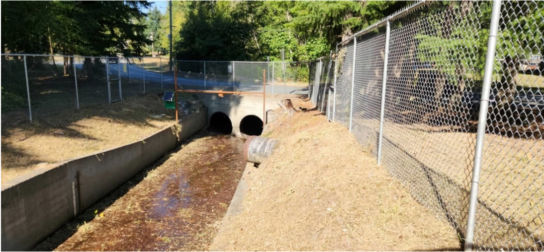
UCR 4: Spillway Structure and FlowDar System (looking Downstream)
