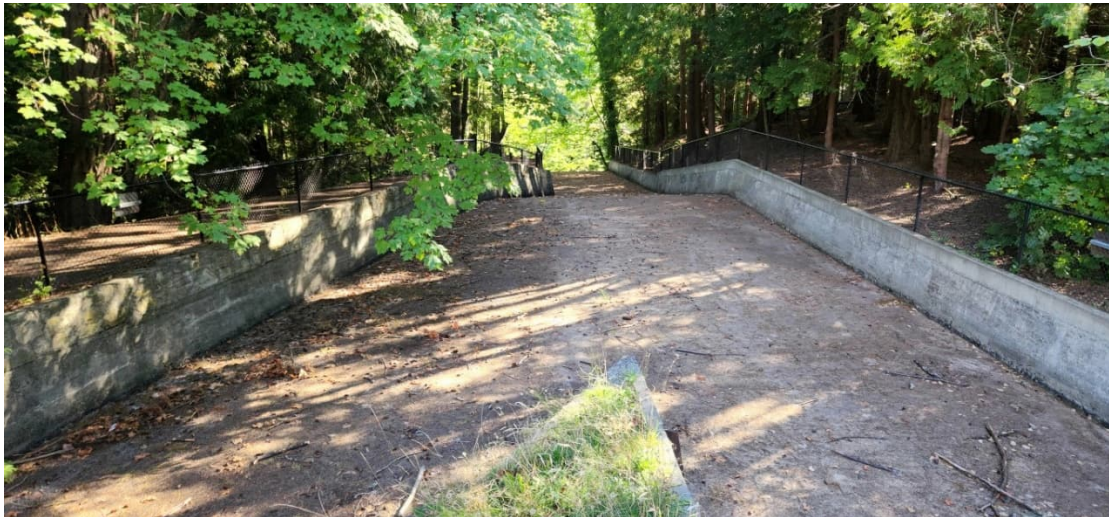
LCR 3: Spillway Structure (Downstream Side of Bridge)
