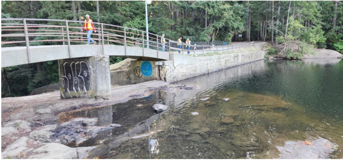
MCR 2: Upstream Wall of the Dam and Spillway
