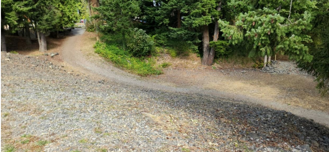
WWL 8: Downstream Face of Main Dam
