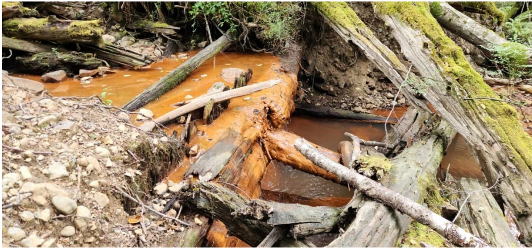
WCL 4: Right Abutment of Dam
