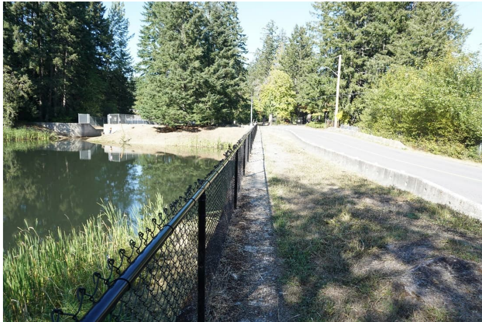
UCR 14: Fencing Along Buttress Dam
