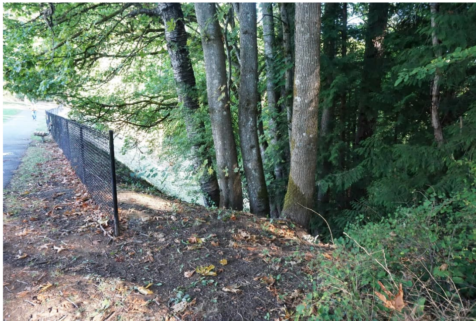
LCR 17: Large Trees at Right Abutment (Downstream)
