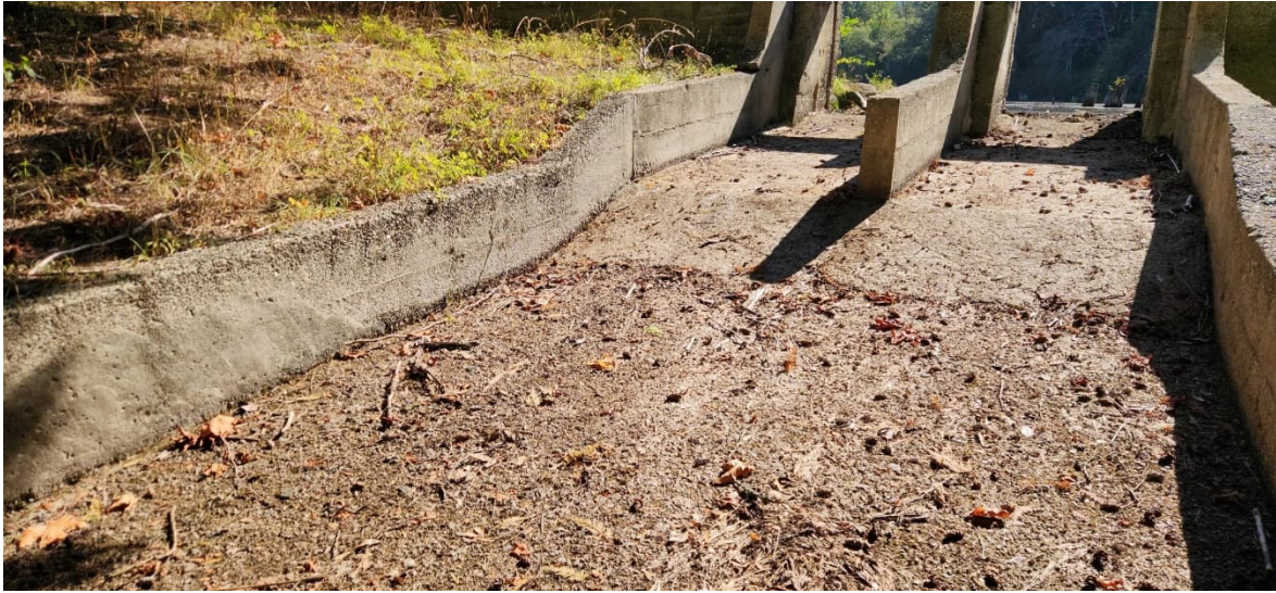
HAW 5: Spillway Chute looking Upstream
