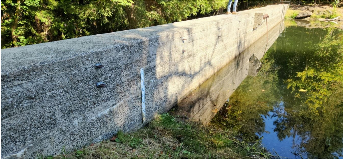
HAW 1: Dam Crest from the Left Abutment
