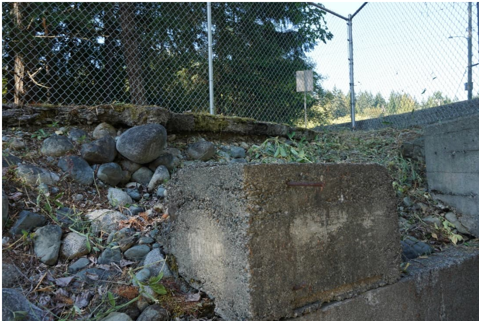
UCR 11: Spillway Wingwalls from Left Abutment
