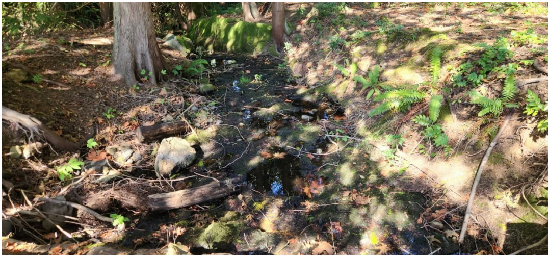
HAW 11: Channel Downstream of Spillway with Minimal Riprap Protection
