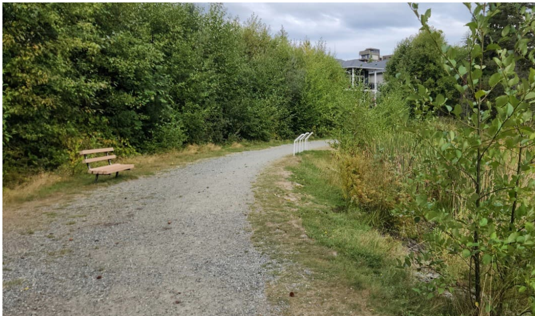
MGC 1: Dam Crest (from Right Abutment of Spillway Bridge)
