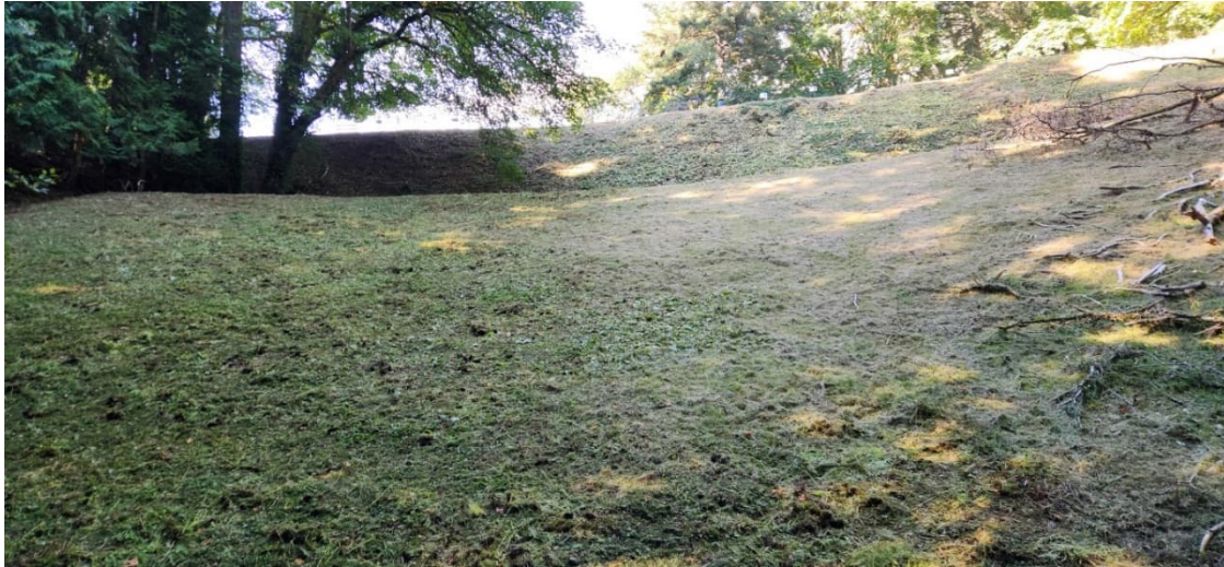
LCR 18: Large Trees at Left Abutment (Downstream)
