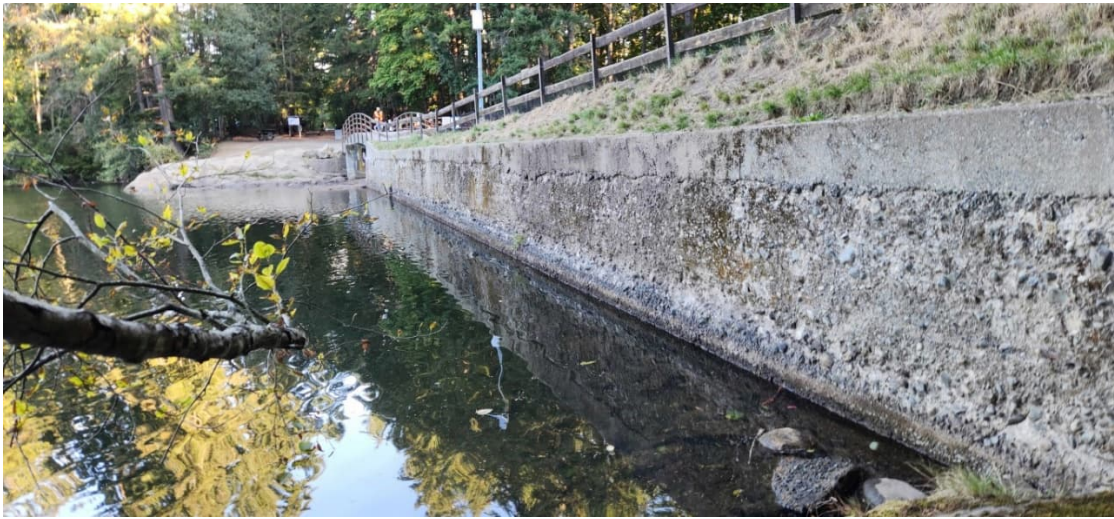
MCR 1: Upstream Wall of the Dam (from Right Abutment)
