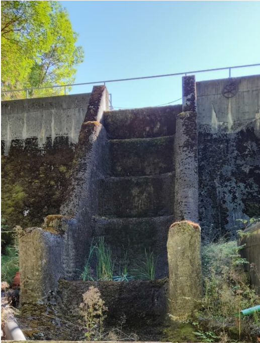
R01 3: Downstream Face and Spillway of the Dam
