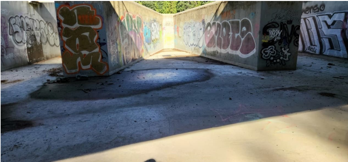
LCR 14: Downstream Face of Auxiliary Spillway Structure
