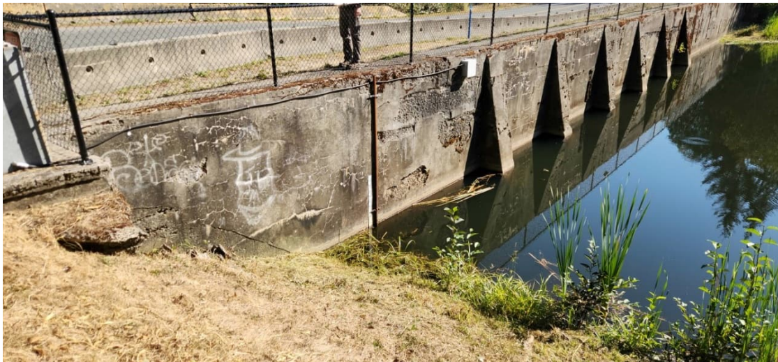
UCR 15: Camera Pole Foundation at Left Abutment
