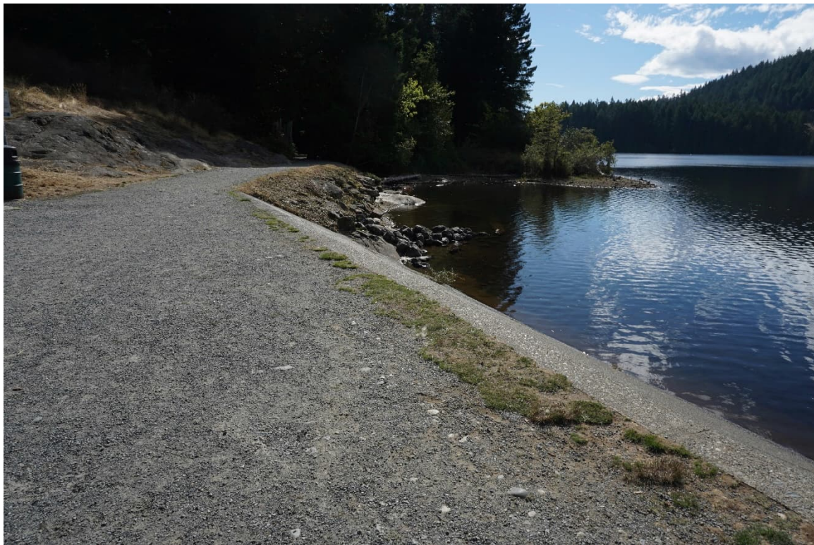
WWL 6: Dam Crest of Main Dam (Looking towards the Right Abutment)
