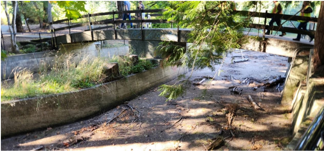
LCR 4: Spillway Chute Structure (Looking Upstream)
