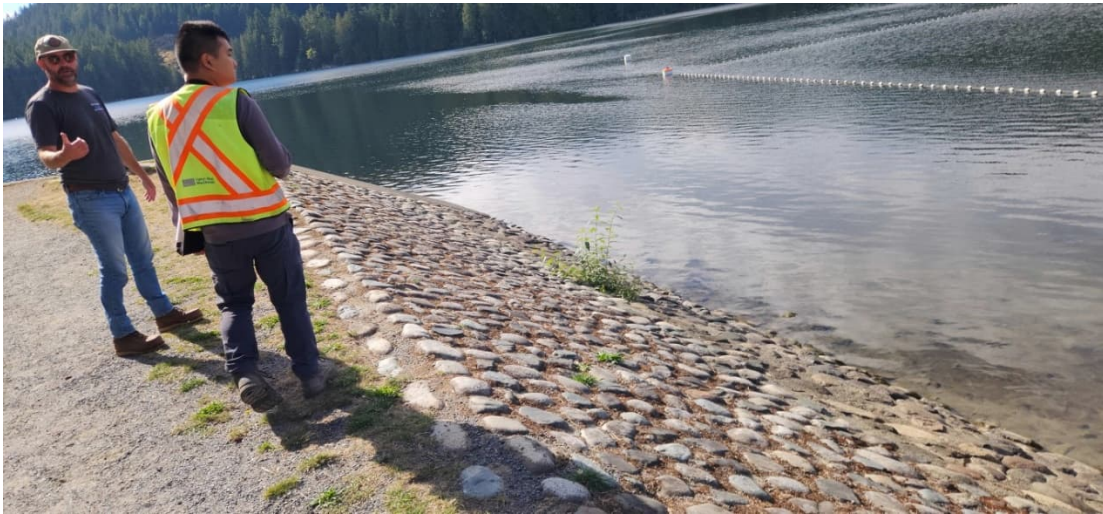
WWL 5: Upstream Stone Face of Main Dam
