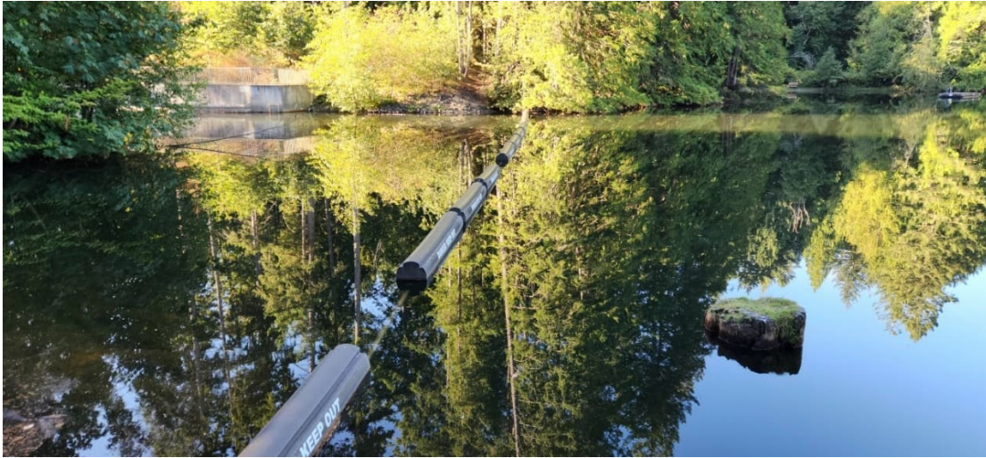
LCR 2: Safety Boom Upstream Side of Auxiliary Spillway
