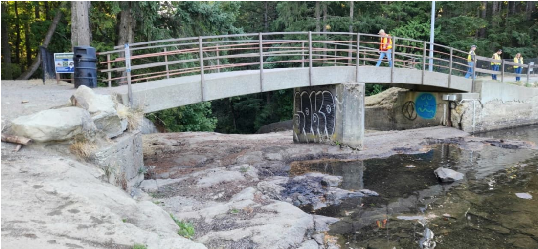
MCR 8: Spillway Chute Structure
