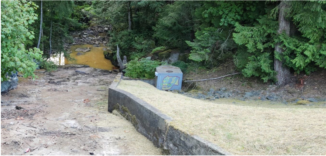
MCR 13: 'V' Notch Weir Housing at Downstream Toe
