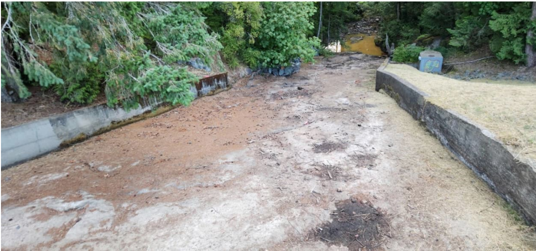
MCR 6: Spillway Chute Slab (Looking Downstream)
