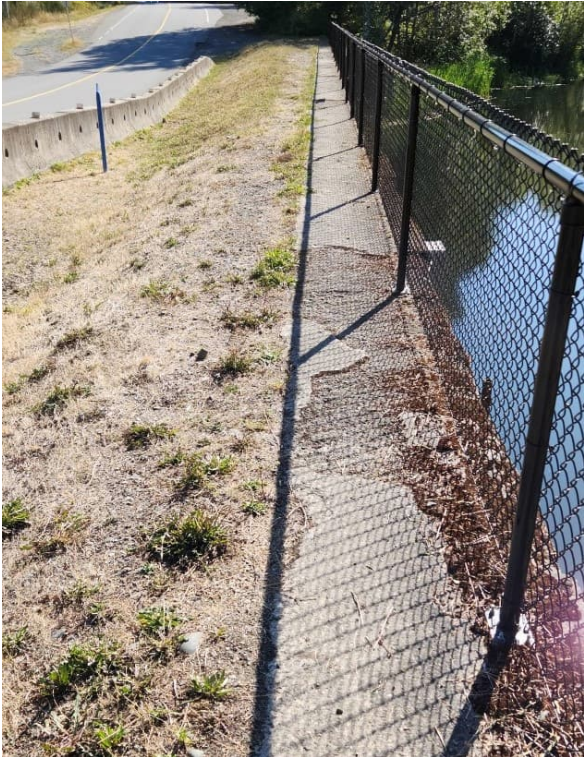
UCR 2: Crest from Right Abutment of Concrete Face of Dam
