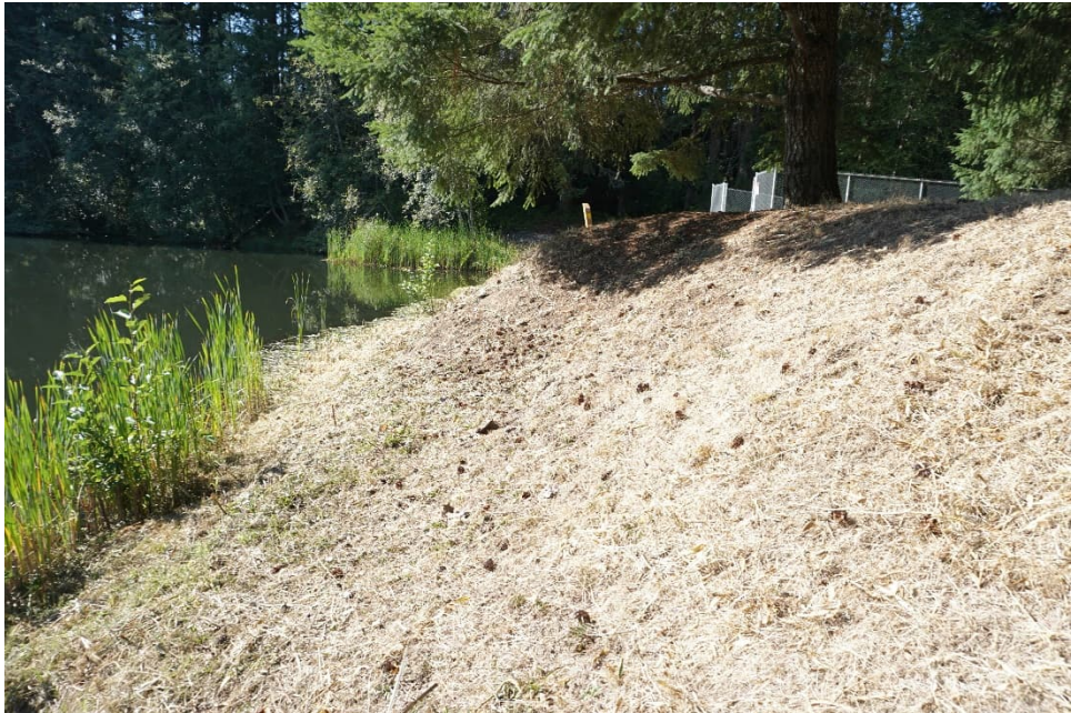
UCR 5: Embankment Dam and Vegetated Shoreline, Looking from Buttress Dam Towards Spillway
