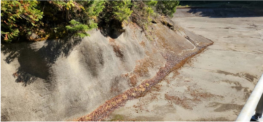
R01 2: Dewatered Reservoir Looking Upstream from the Dam
