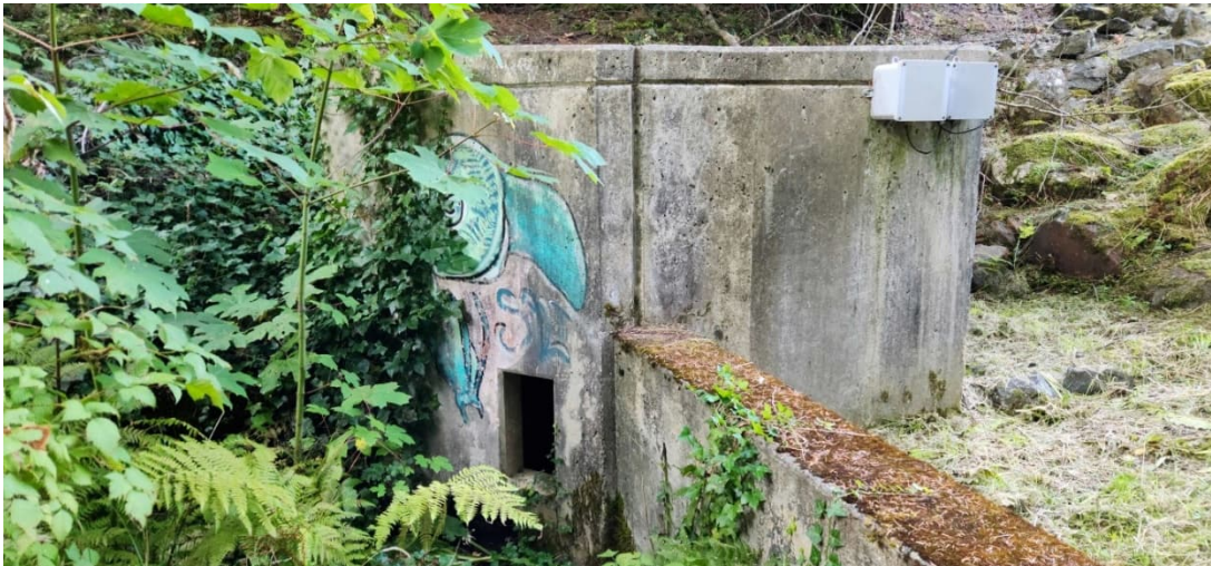
MCR 14: 'V' Notch Weir Concrete Housing (Weir Not Visible)
