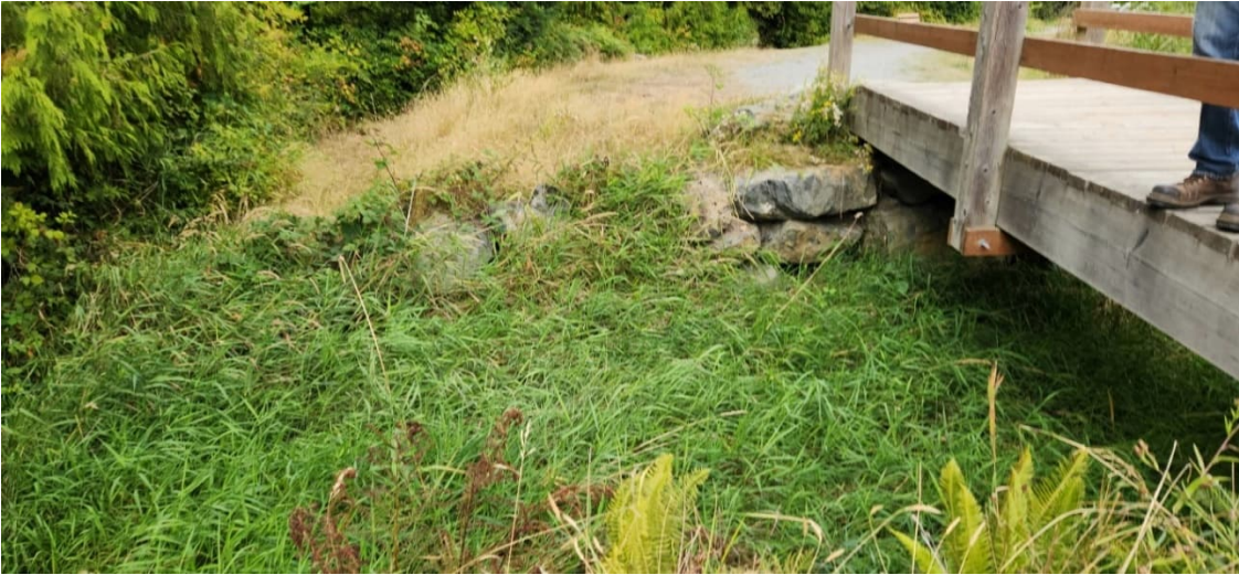
MGC 6: Downstream of Spillway
