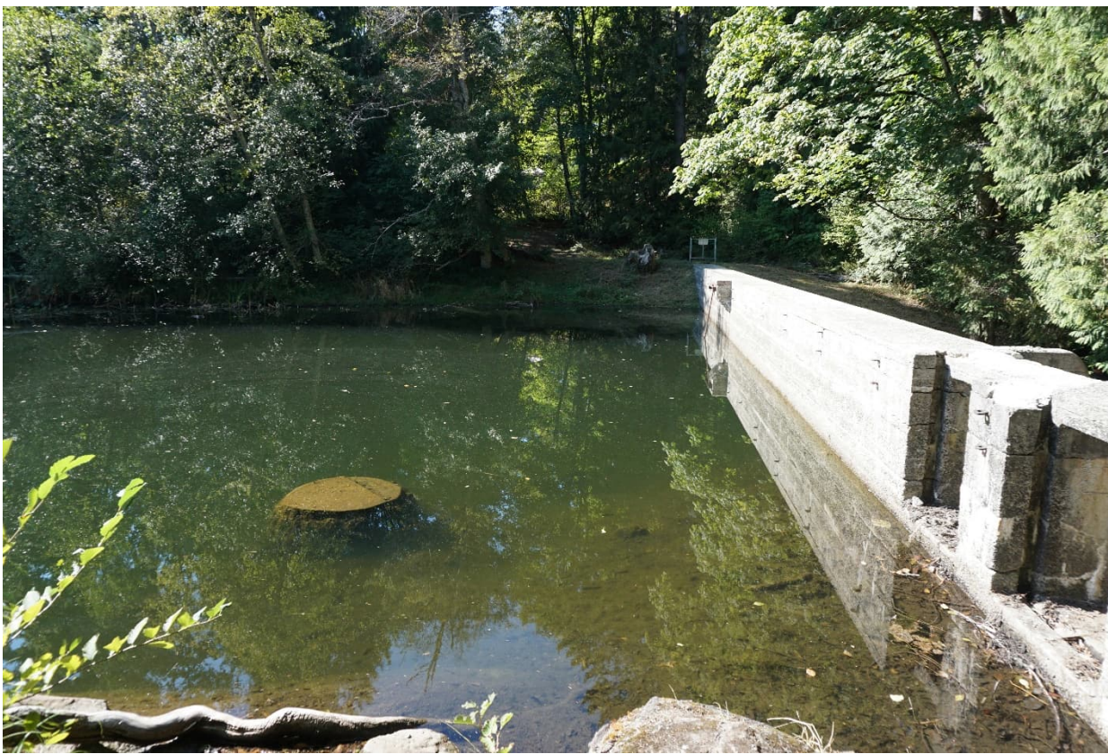
HAW 3: Upstream Face of the Dam and Spillway from Right Abutment
