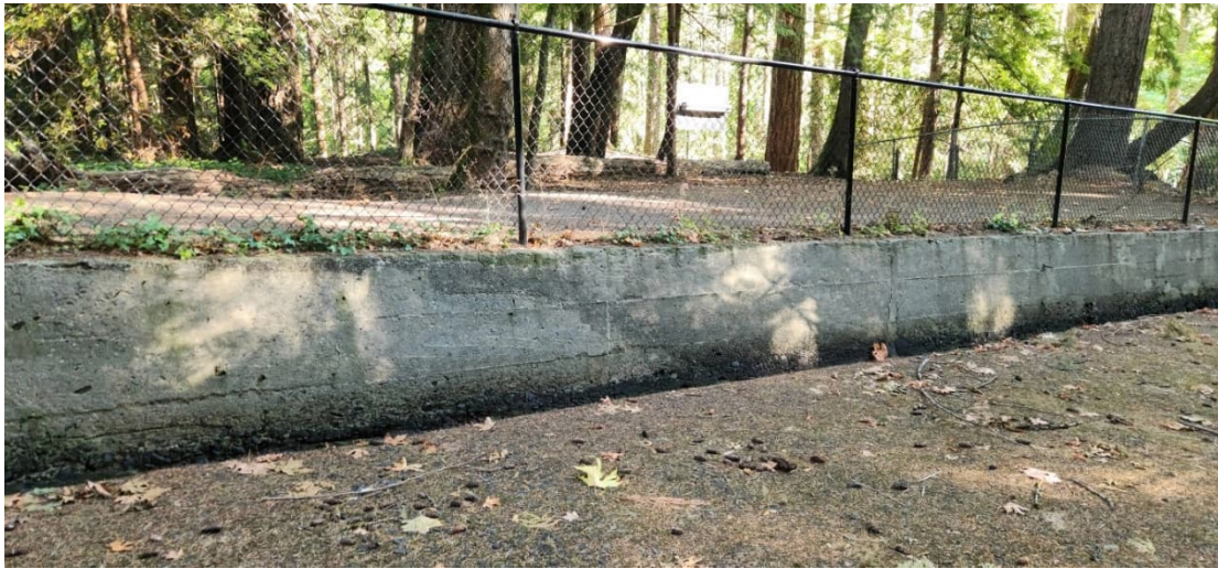
LCR 10: Repair at the Base of Spillway Chute Left Wall
