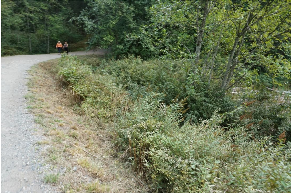
WWL 13: Upstream Face of Saddle Dam
