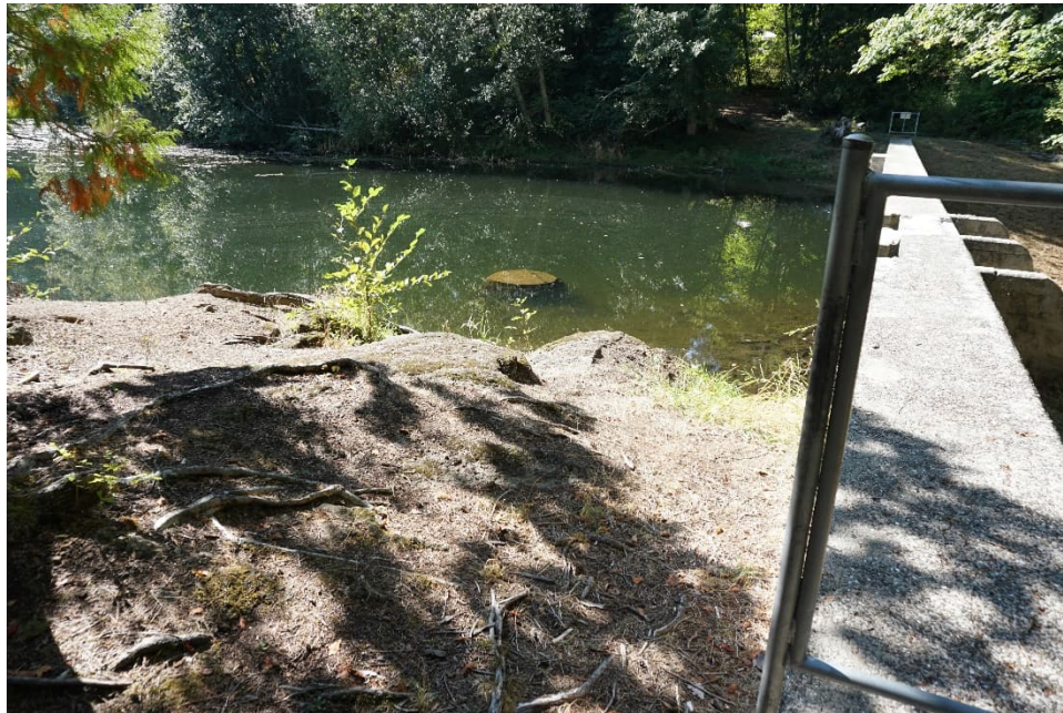
HAW 2: Dam Crest from the Right Abutment
