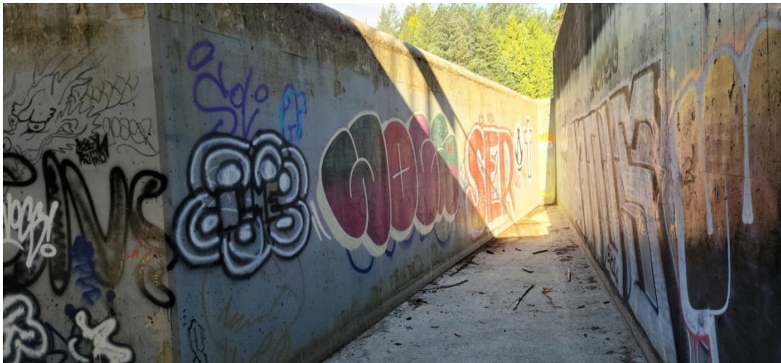
LCR 15: Downstream Face of Auxiliary Spillway (Wet Area at Corner)
