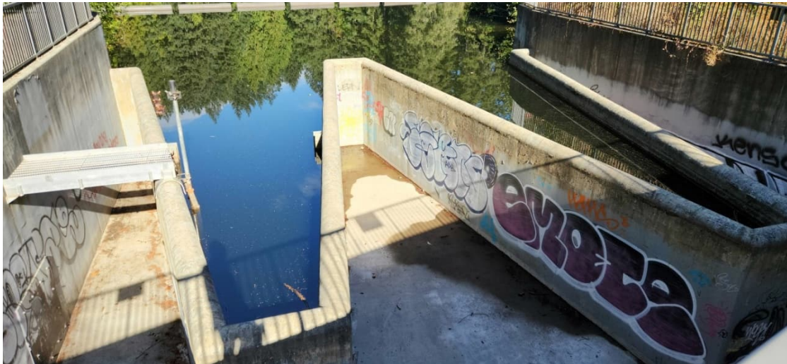
LCR 13: Auxiliary Spillway Structure Looking Upstream with Safety Boom Beyond
