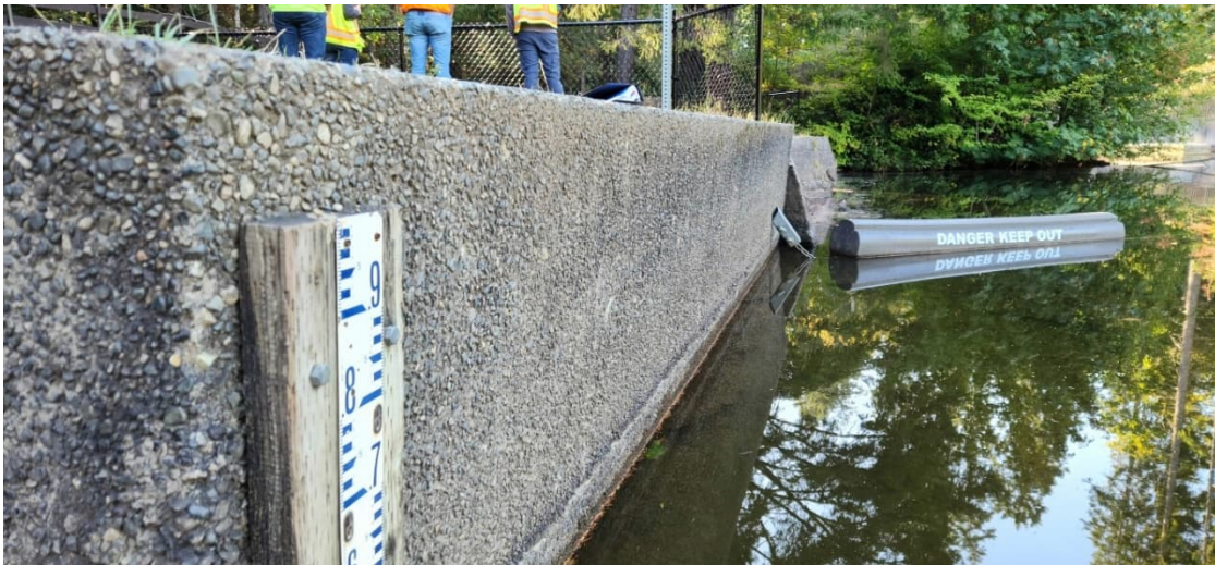
LCR 1: Upstream Face of the Dam with Reservoir (from Left Abutment)
