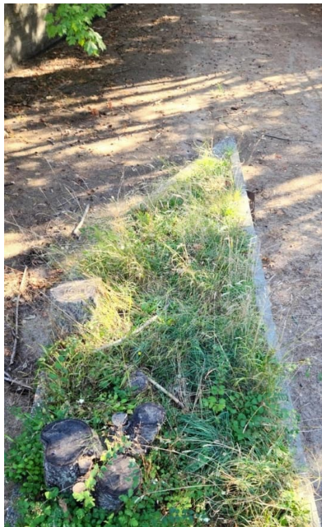
LCR 11: Spillway Chute Structure (looking Downstream)
