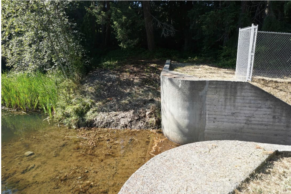
UCR 10: Spillway Wingwalls
