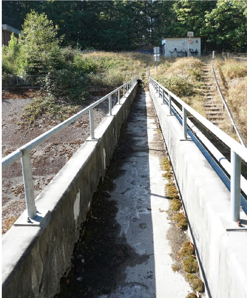
R01 6: Dam Crest and Left Abutment Slope and Wooden Access Stair and Handrail Downstream of Dam
