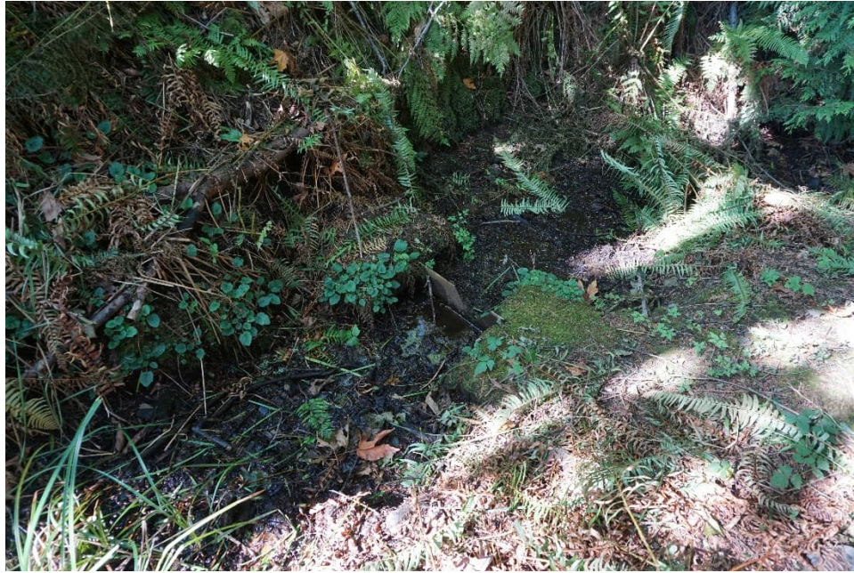
HAW 9: 'V' Notch Weir (Looking Downstream)
