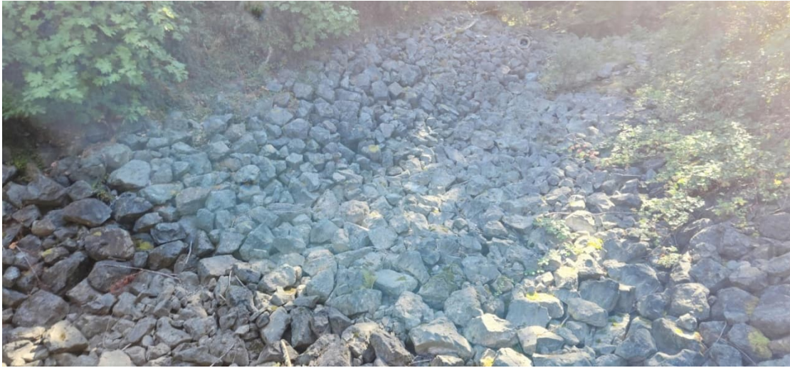
LCR 20: Well-Interlocked Riprap Downstream of Auxiliary Spillway Looking Downstream
