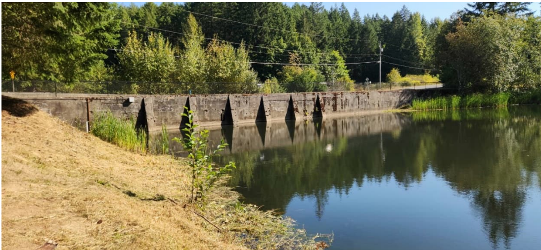
UCR 1: Buttressed Retaining Wall at Upstream Face of the Dam
