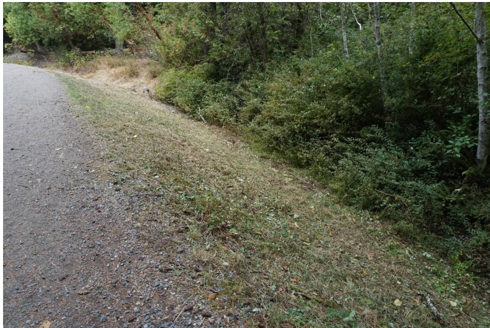
WWL 12: Downstream Face of Saddle Dam
