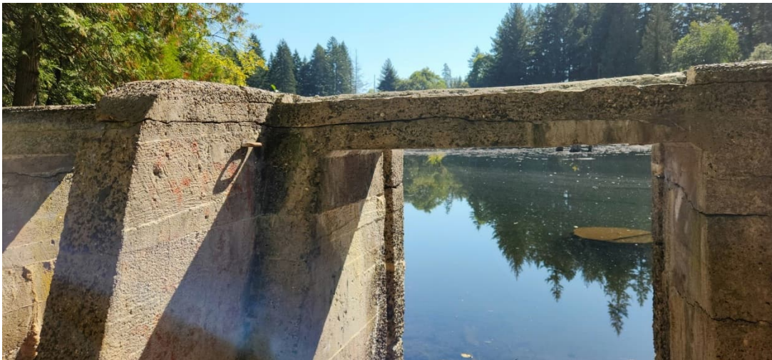
HAW 10: Left Spillway Bay Looking Upstream
