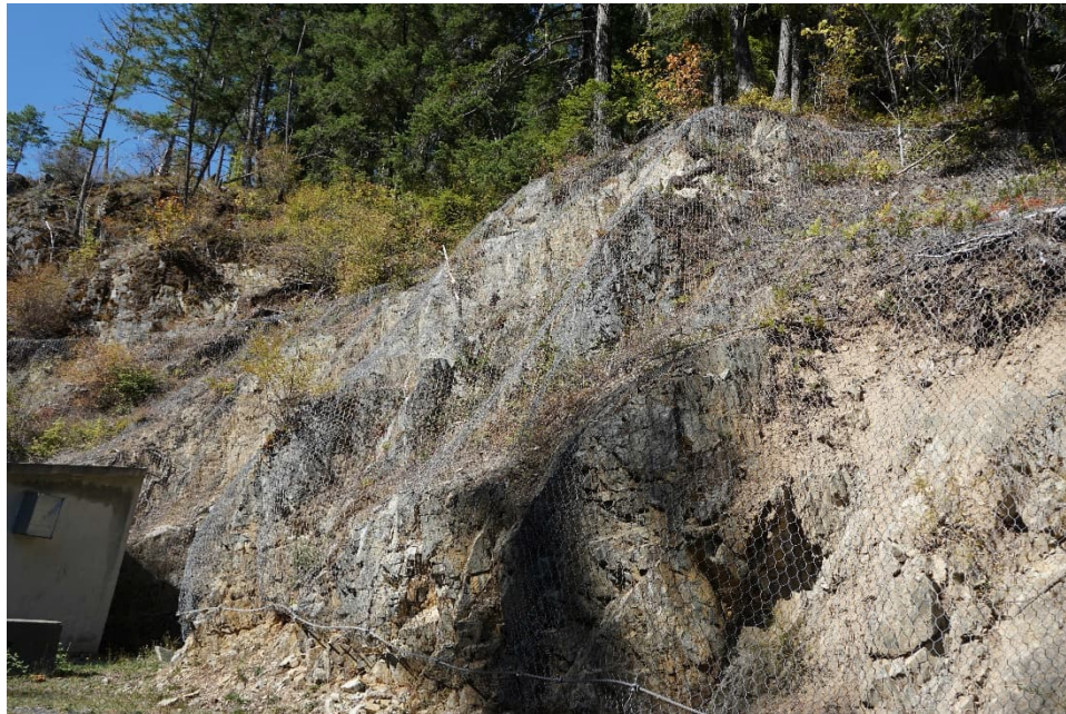
SFK 12: Rock Slope with Rock Bolts and Mesh Installed Behind Building
