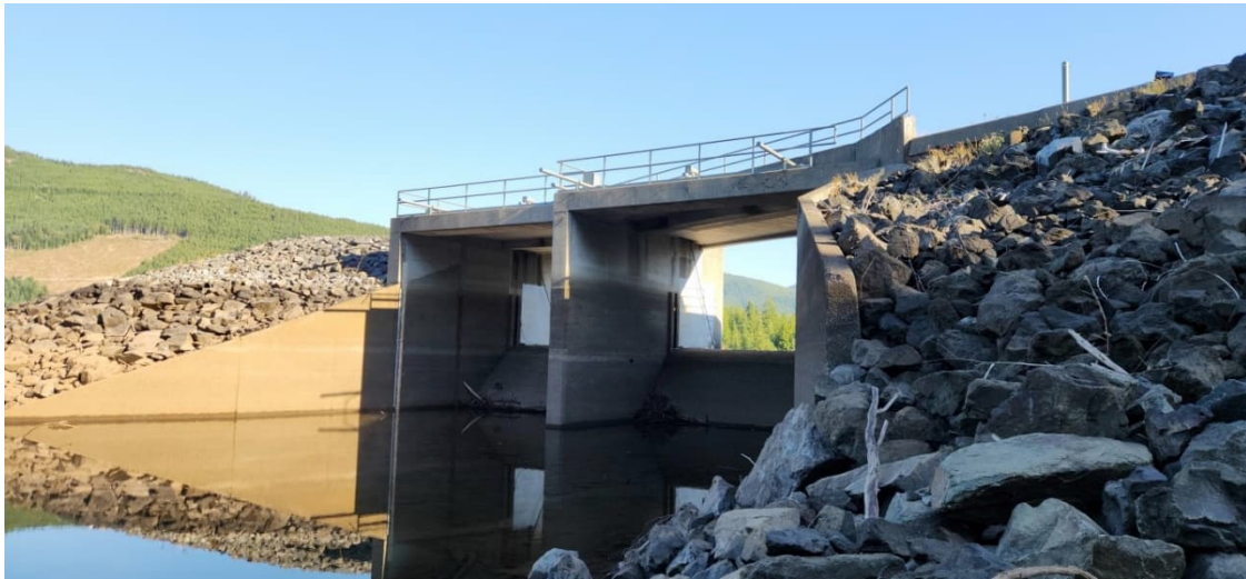
JCR 5: Upstream Side of Spillway Structure
