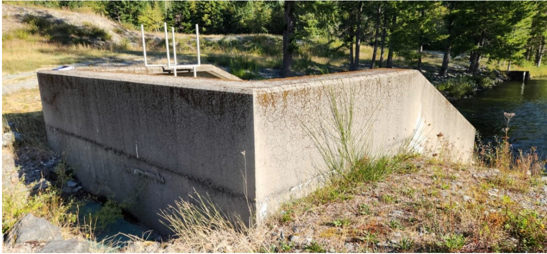
JCR 21: LLO Concrete Structure at Downstream Side (Right Wingwall)
