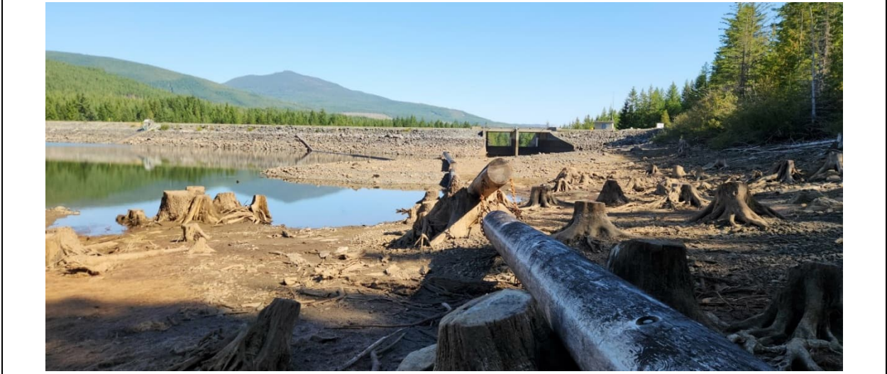
JCR 16: Upstream Face of Dam with Log Boom
