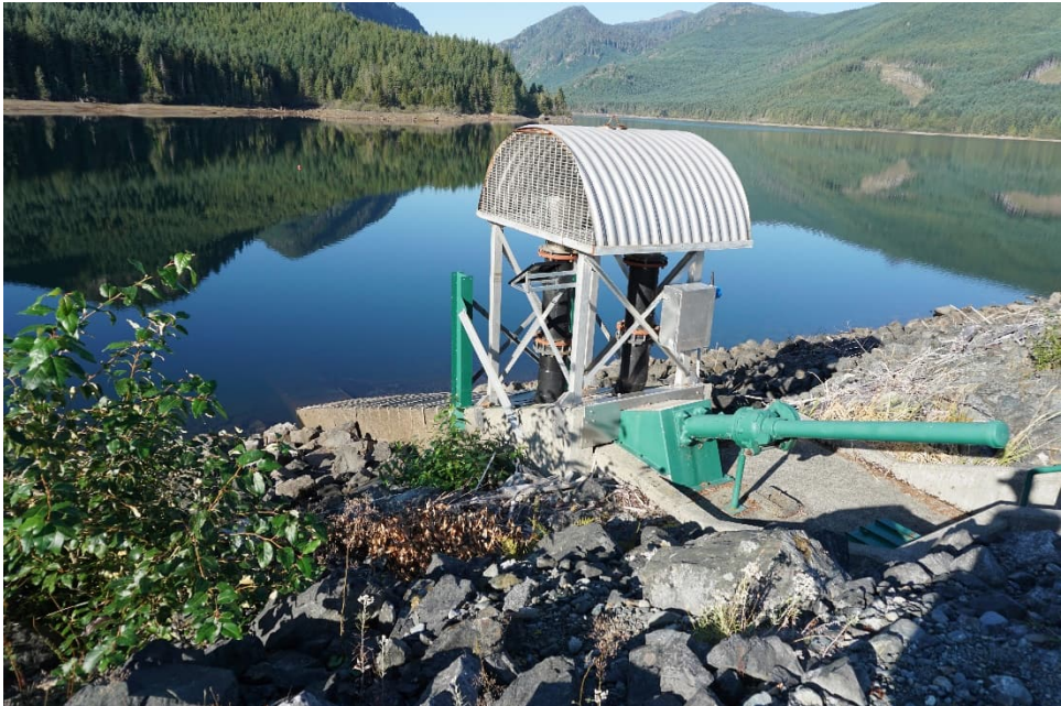
JCR 18: LLO Intake at the Upstream Face of the Dam
