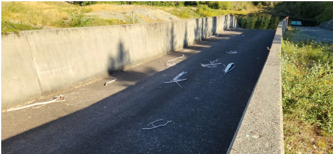
JCR 12: Spillway Structure Chute (looking Downstream)
