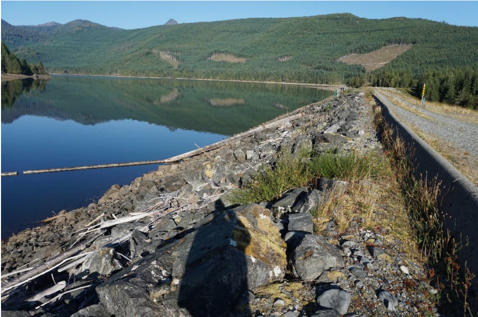
JCR 17: Dam Crest (Looking towards the Left Abutment)
