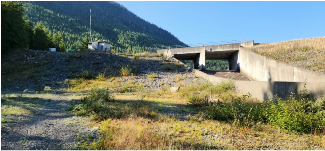
JCR 31: Downstream Right Abutment
