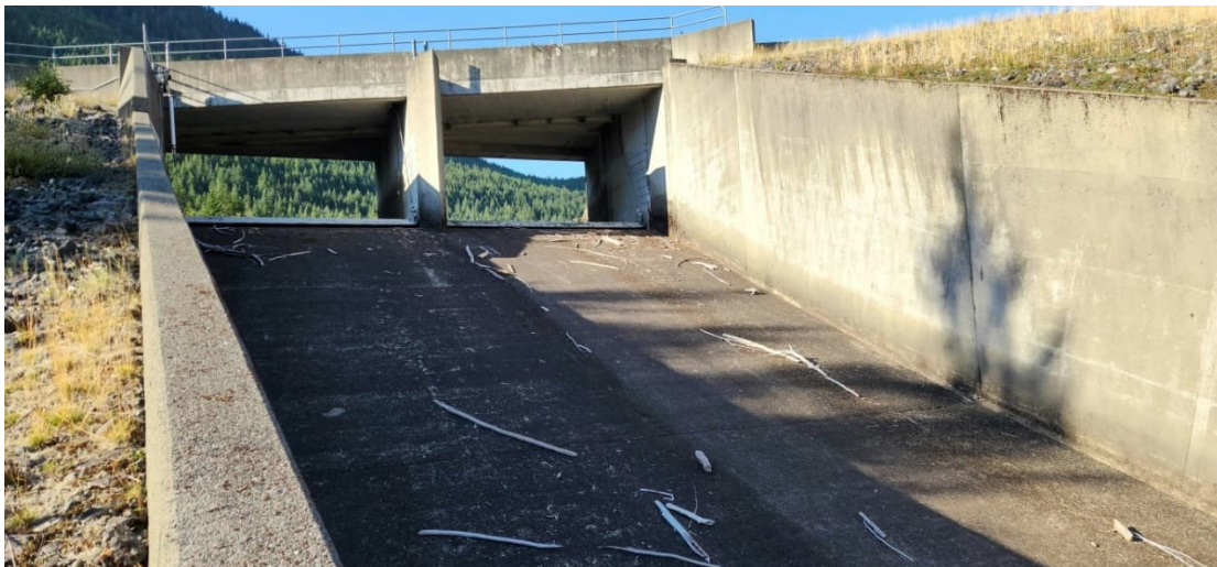
JCR 4: Downstream Side of Spillway Concrete Structure
