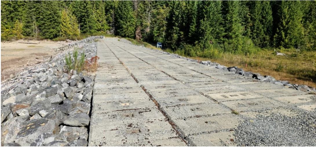
JCR 39: Auxiliary Crest Concrete Block
