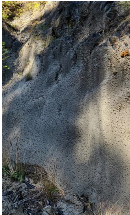
SFK 11: Headwall Shotcrete Condition (Downstream)
