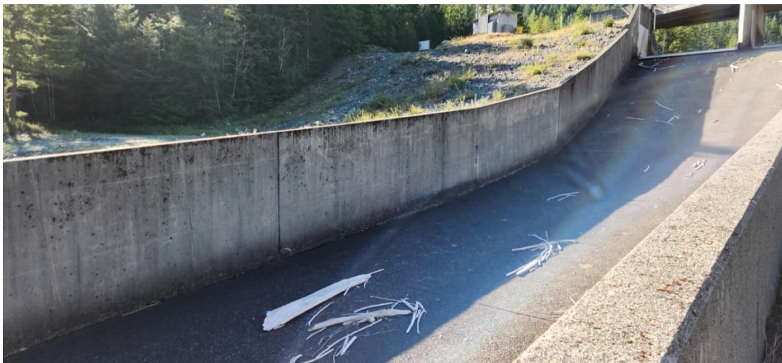
JCR 14: Construction Joints in Spillway Structure Chute
