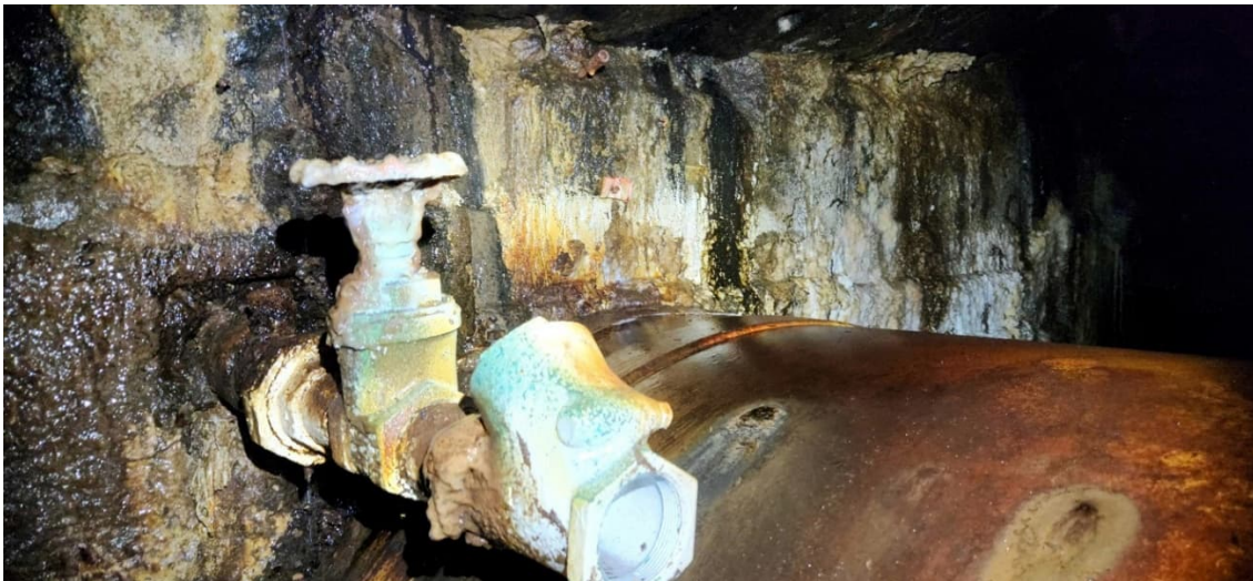
SFK 8: Upstream Face of Intake Tunnel
