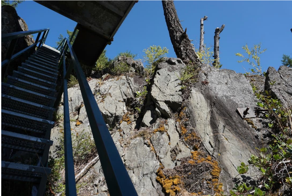
SFK 13: Exposed Bedrock Upstream of Left Abutment
