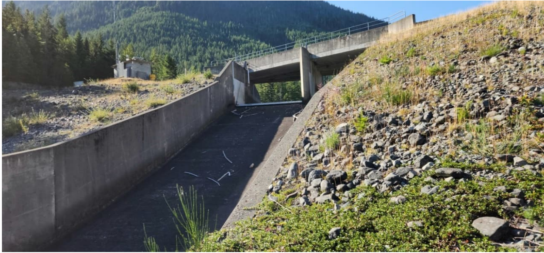
JCR 9: Spillway Chute (looking Upstream)
