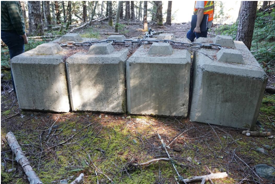
JCR 2: Log Boom at Right Anchors
