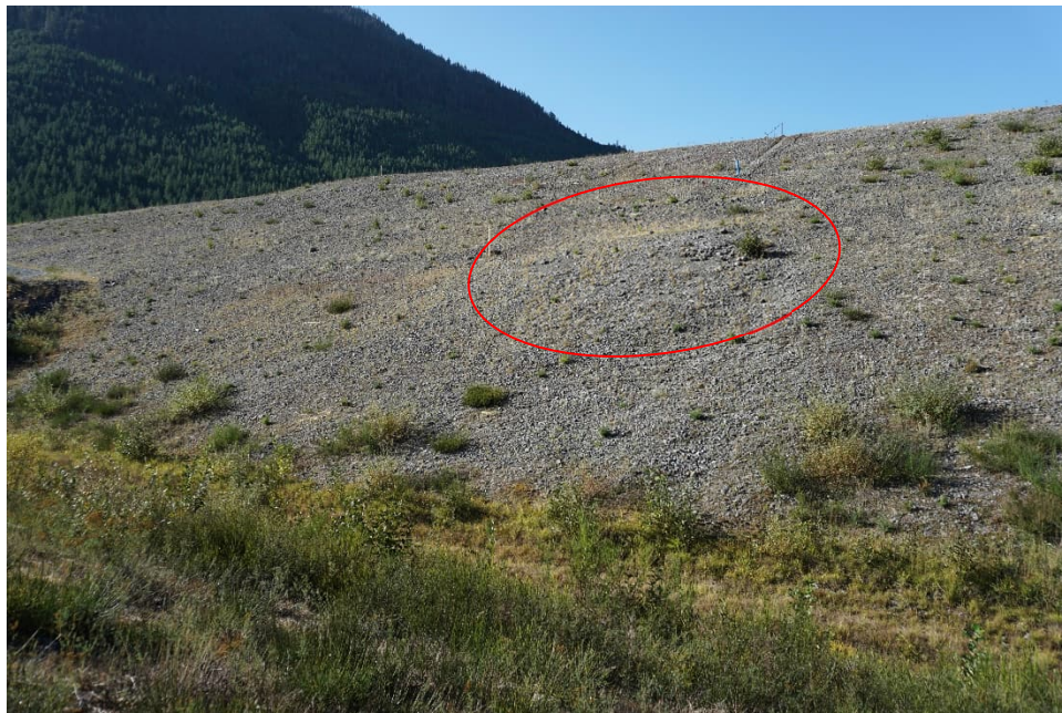
JCR 32: Bulge on Downstream Face (Looking from Downstream Toe)
