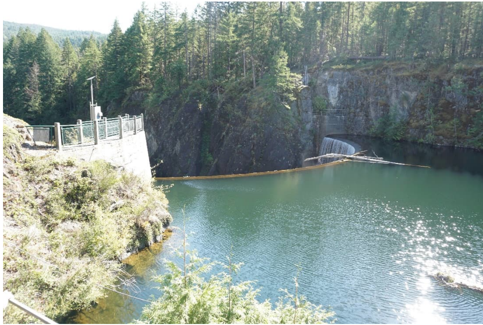
SFK 5: Right Abutment Rockface
