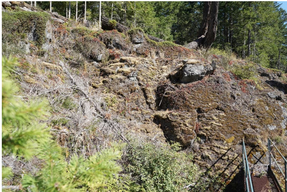
SFK 14: Upstream of Left Abutment
