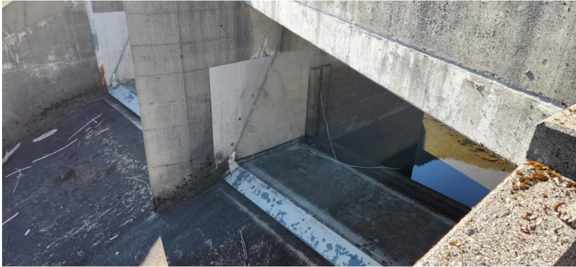
JCR 11: Open Spillway gates
