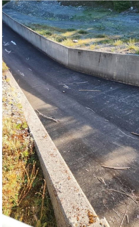
JCR 13: Small Debris Inside Spillway Structure Chute (Looking Downstream)
