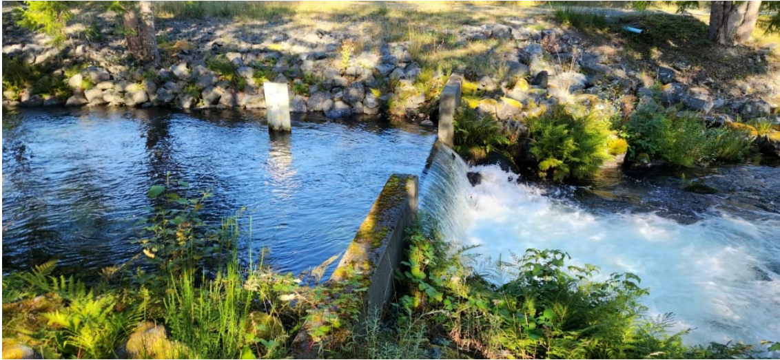
JCR 23: LLO Channel and Downstream Concrete Weir
