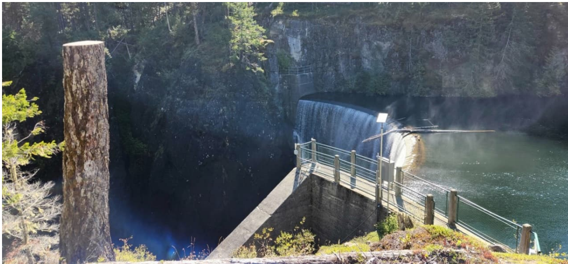
SFK 2: South Fork Dam (looking from Left Abutment)
