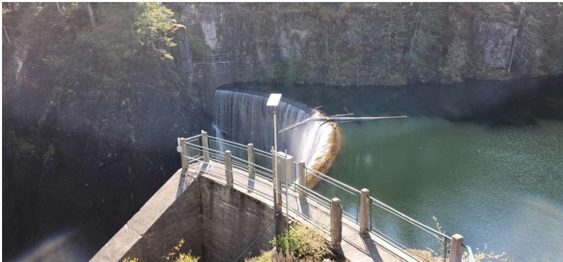
SFK 6: Left and Right Concrete Abutments
