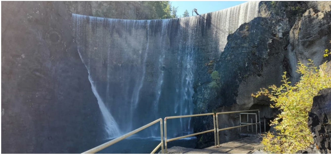
SFK 7: Downstream Face of Dam
