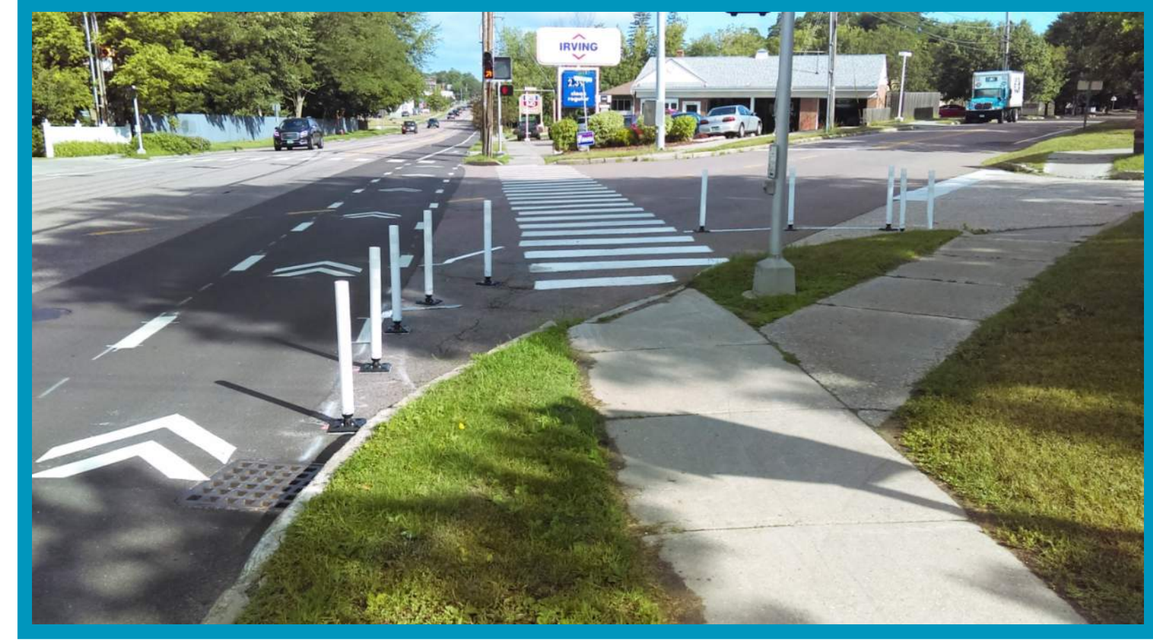
FLEXIBLE POSTS TO REDUCE CROSSING DISTANCE
