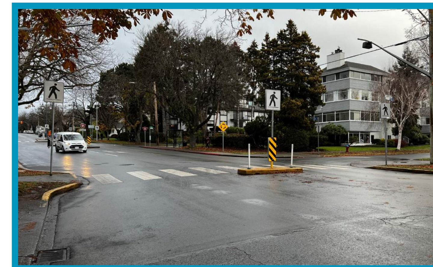
PEDESTRIAN CROSSING WITH PRE-CAST CONCRETE MEDIANS AND SIGNAGE
