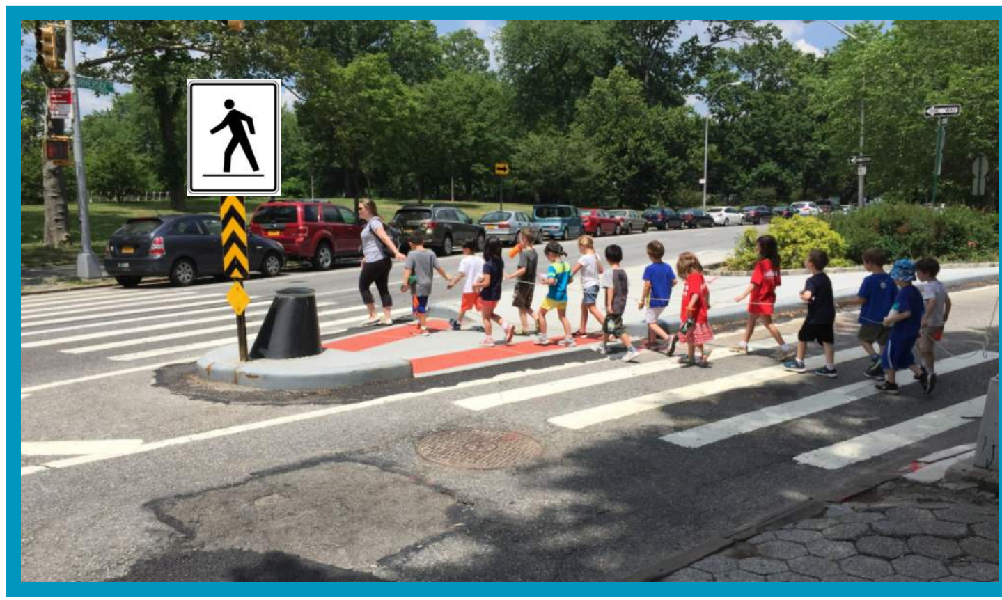
PEDESTRIAN CROSSING WITH CONCRETE MEDIAN/REFUGE ISLAND
