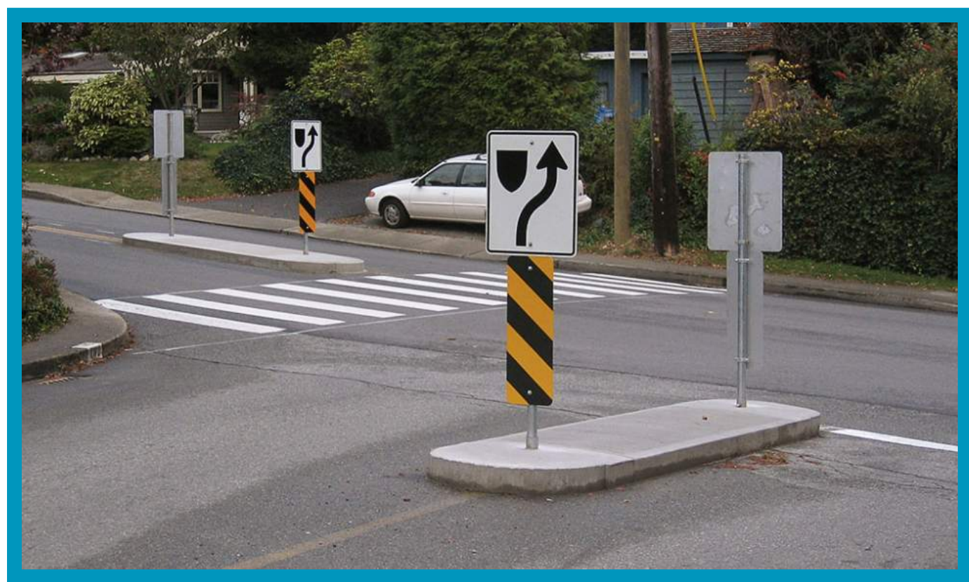
CONCRETE MEDIANS FOR TRAFFIC CALMING
