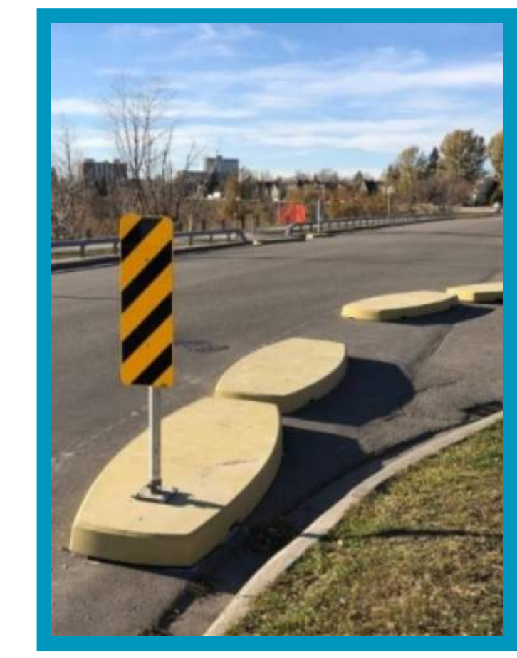
PRE-CAST MEDIAN WITH HAZARD SIGNAGE FOR TRAFFIC CALMING
