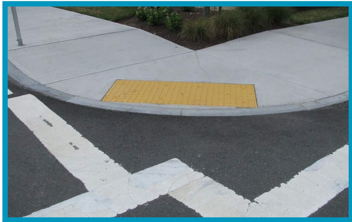
TACTILE WALKING SURFACE INDICATOR FOR VISUALLY IMPAIRED PEDESTRIANS
