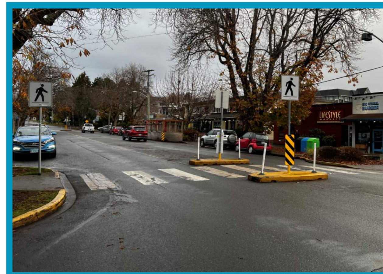
PEDESTRIAN CROSSING WITH PRE-CAST CONCRETE MEDIANS AND SIGNAGE
