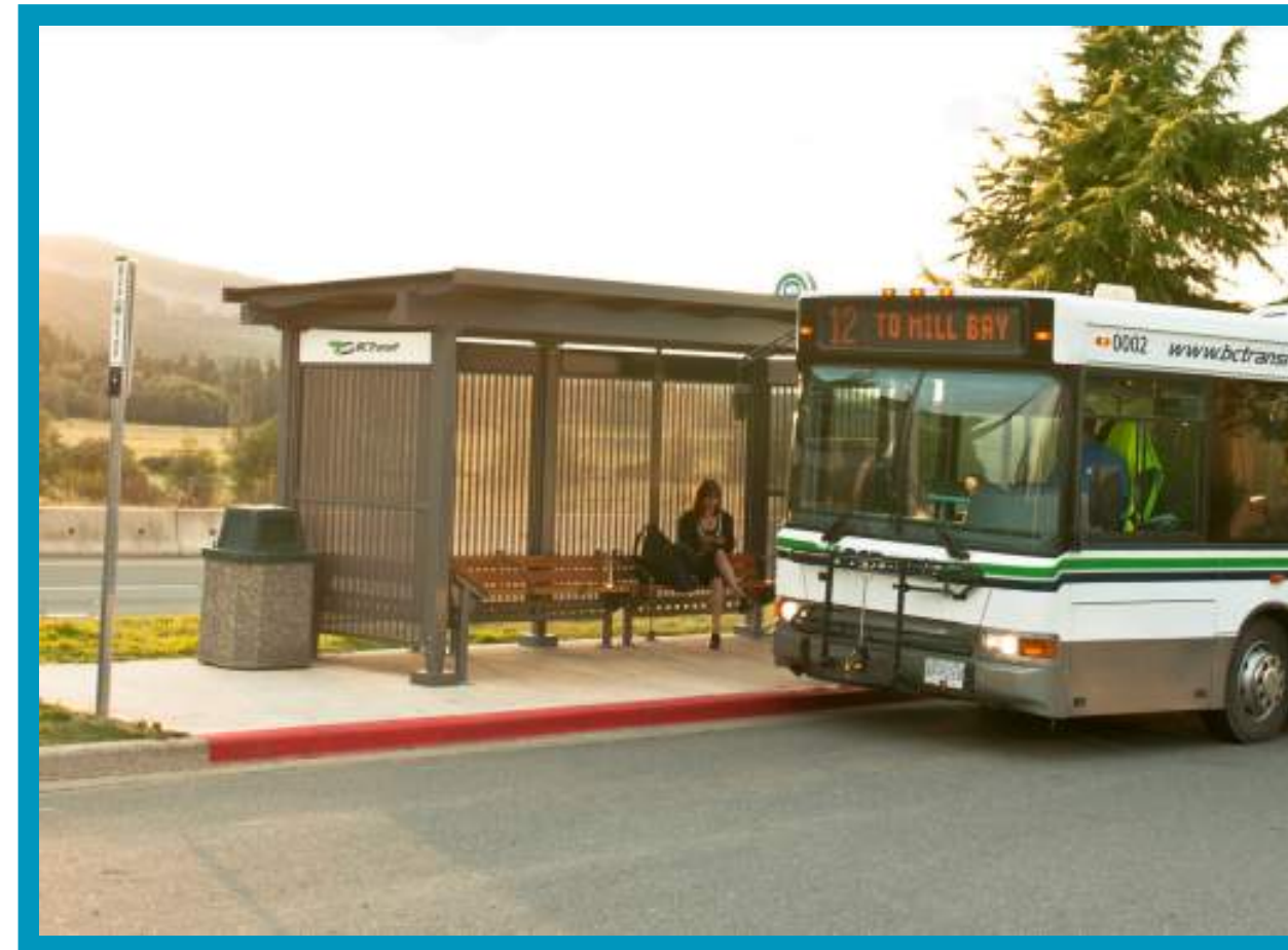
CONCRETE BUS STOP PAD
