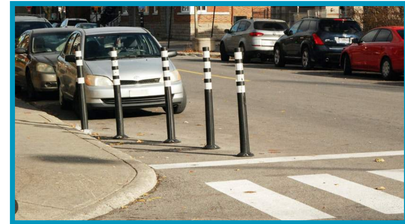
FLEXIBLE POSTS TO TIGHTEN CORNER RADIUS AND REDUCE PEDESTRIAN CROSSING DISTANCES
