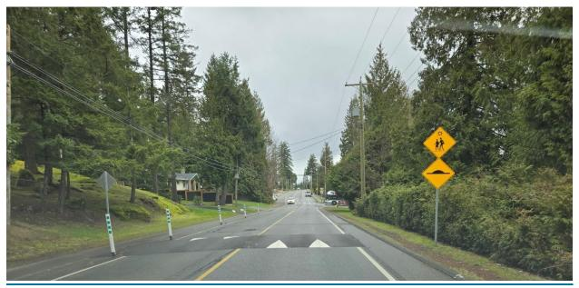
Figure 7 - Traffic Calming Infrastructure on Extension Road to the South of Cinnabar Drive, Including Signage, Speed Tables, Flexposts, Pavement Markings, and Rapid Flashing Beacons
