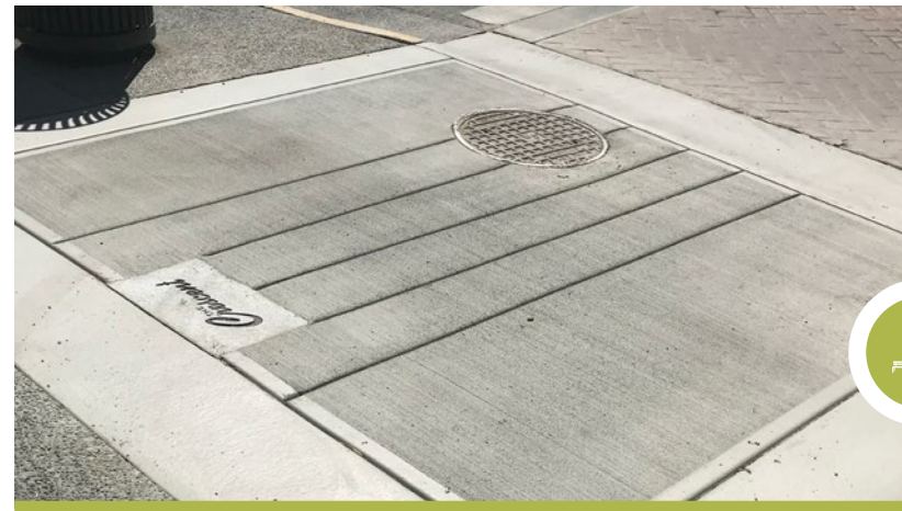
Victoria Crescent, Nanaimo. Broom-finished concrete with tooled joints and integrated wayfinding elements.
