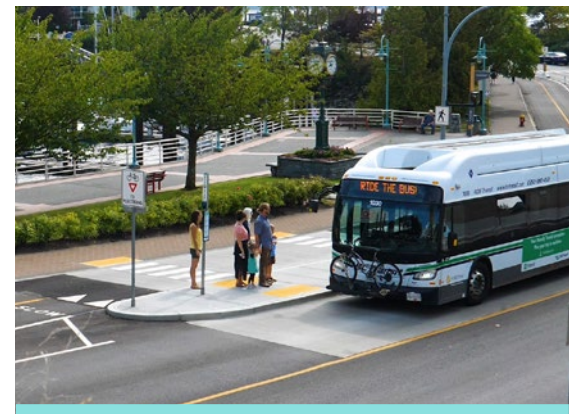
Front Street, Nanaimo. Continuous sidewalk transit stops extend the sidewalk material (concrete) through the cycling facility in addition to signage and road markings, strengthening the indication that cyclists must yield to pedestrians in this zone.
