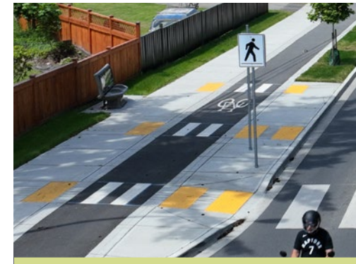
Metral Drive, Nanaimo. High contrast TWSIs indicate where pedestrians may cross the path of a motor vehicle or bicycle.
