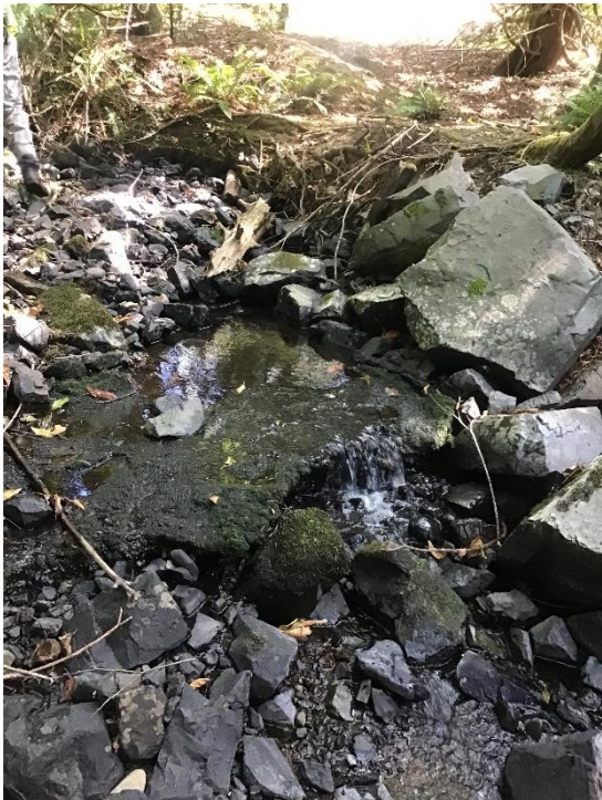
Figure 12. Boulders used for bank armoring in Reach 2 of Cottle Creek within Stephenson Point Park.
