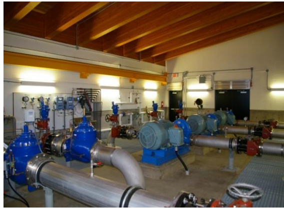
Inside the new Energy Recovery Facility - April 1, 2015
