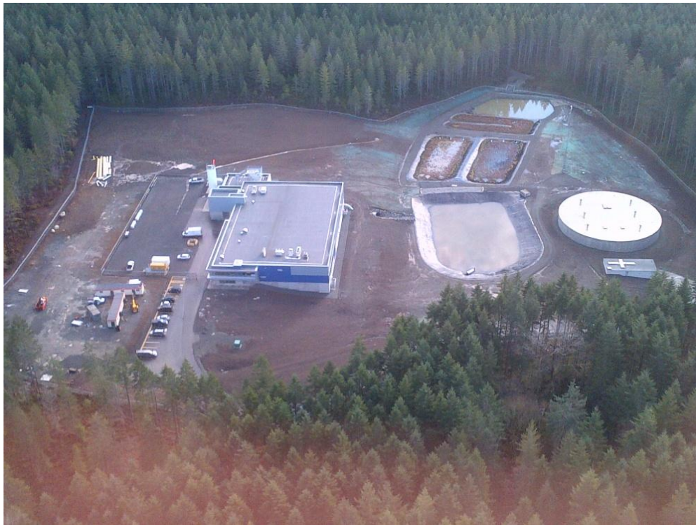
new Water Treatment Plant building, wetlands & clearwell tank – January 28, 2016
