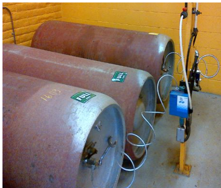
chlorine tanks at Water Process Centre
