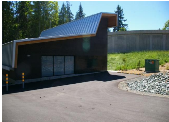
The new Energy Recovery Facility and drinking water storage tank - April 1, 2015
