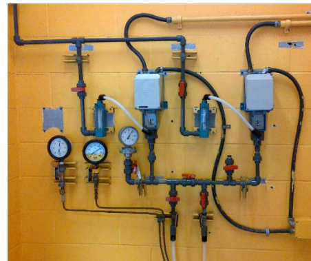
chlorine disinfection at Water Process Centre
