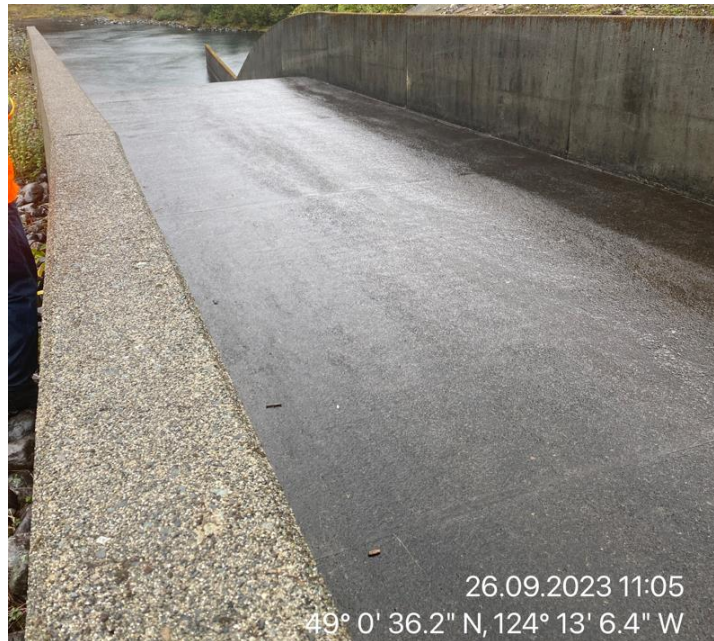
JCR 15: Spillway Structure Chute
