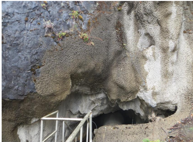
SFK 3: Shotcrete at the Entry to Water Supply Tunnel
