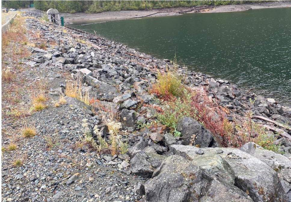
JCR 34: Good Condition Riprap with Average Interlock Observed on Upstream Face of Dam (Looking towards the Right Abutment)
