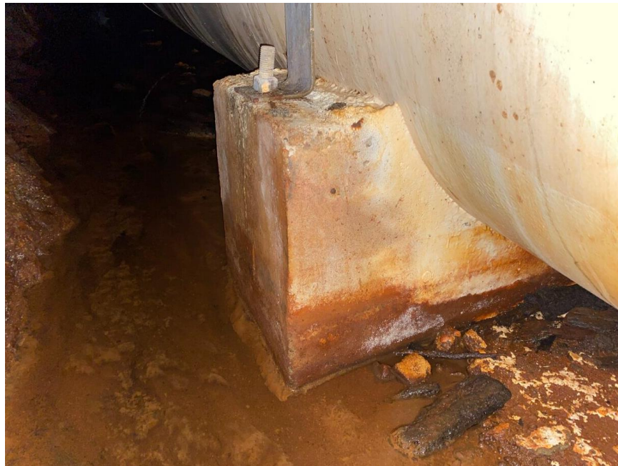
SFK 9: Water Supply Pipe Anchor and Foundation Block
