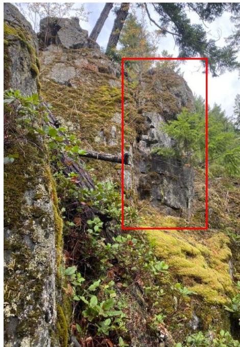
SFK 14: Potential Rock Block Instability Located Upstream of Left Abutment
