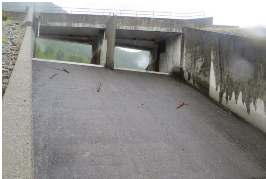
JCR 4: Downstream Side of Spillway Concrete Structure
