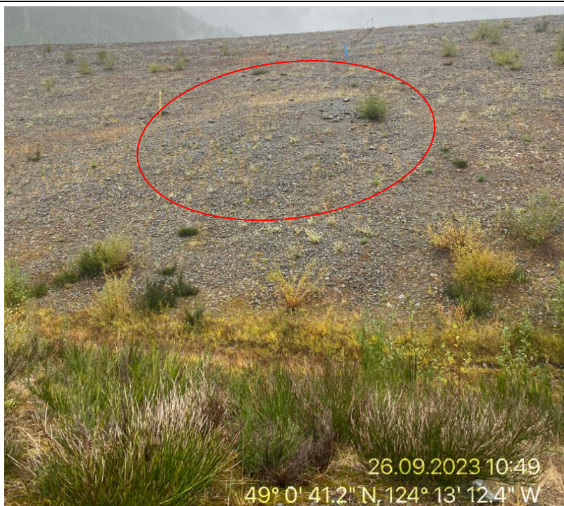
JCR 37: Bulge on Downstream Face (Looking from Downstream Toe)
