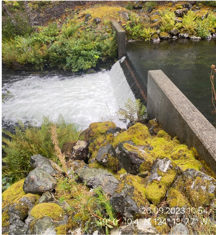
JCR 23: LLO Channel and Downstream Concrete Weir
