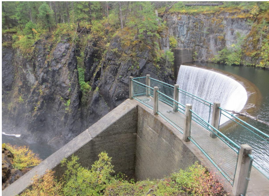
SFK 6: Left and Right Concrete Abutments
