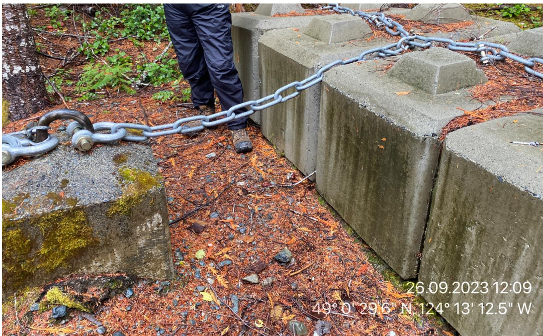
JCR 2: Log Boom at Right Anchors
