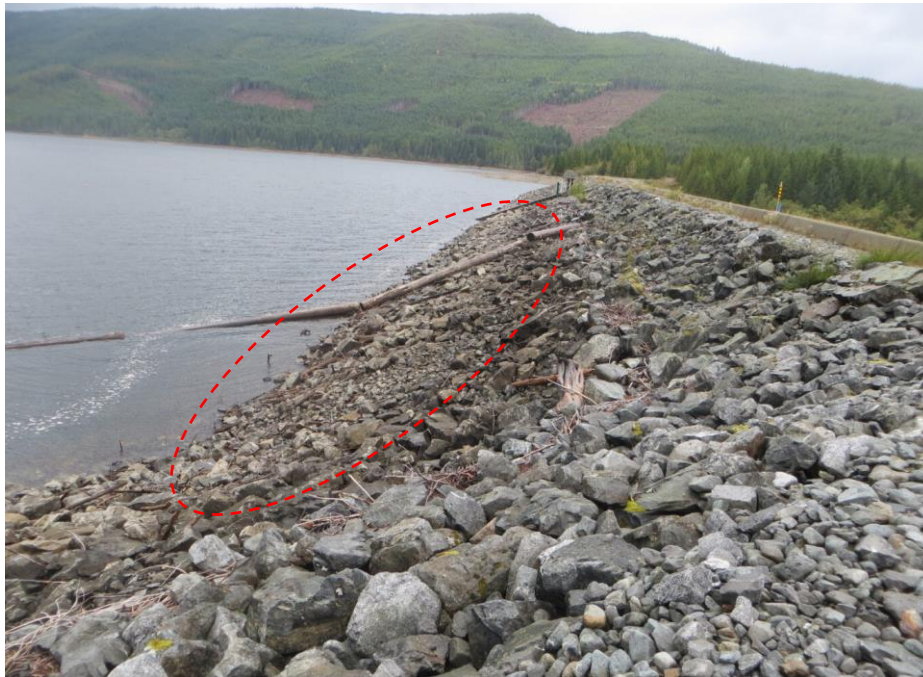
JCR 1: Upstream Face of the Dam, with Smaller Size Rock Particles along the Reservoir
