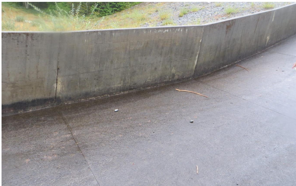
JCR 14: Construction Joints in Spillway Structure Chute
