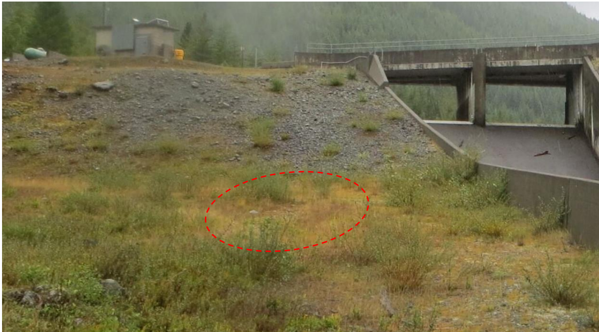
JCR 32: Sign of Seepage on Downstream Face Near the Right Abutment
