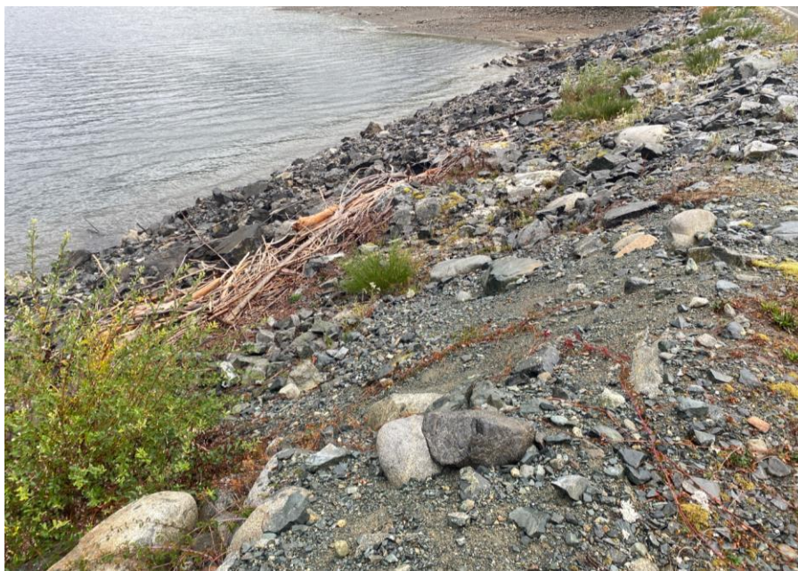
JCR 35: Poor Quality Riprap Left of Piezometer SP12
