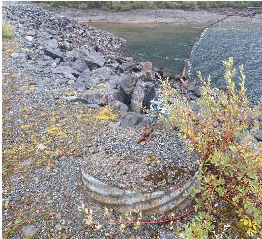
JCR 3: Log Boom Left Anchor
