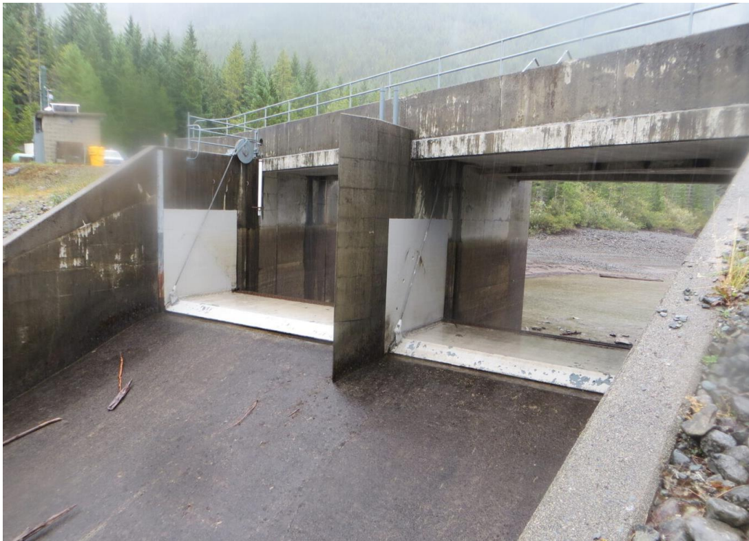
JCR 11: Open Spillway gates
