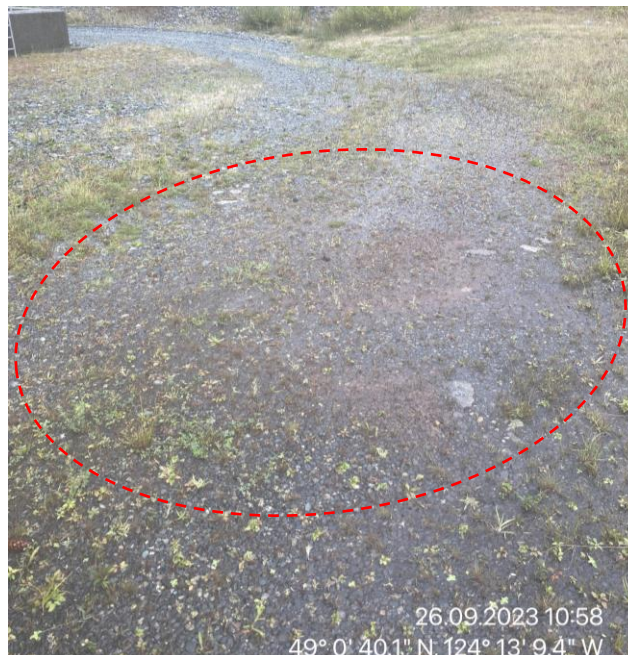
JCR 33: Previously Observed Wet Spot on the Lower Access Road Upstream of Weir E
