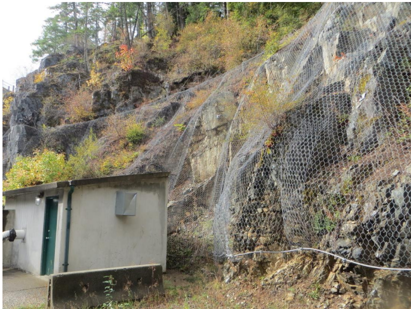
SFK 12: Rock Slope with Rock Bolts and Mesh Installed Behind Building
