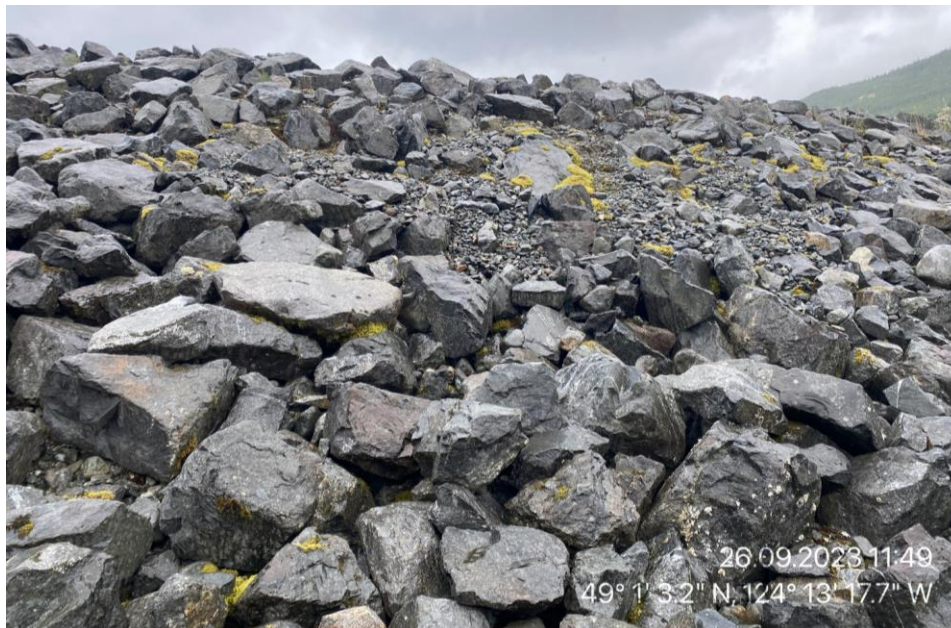
JCR 43: Auxiliary Spillway and Downstream Face of Dam, zone with sparse riprap
