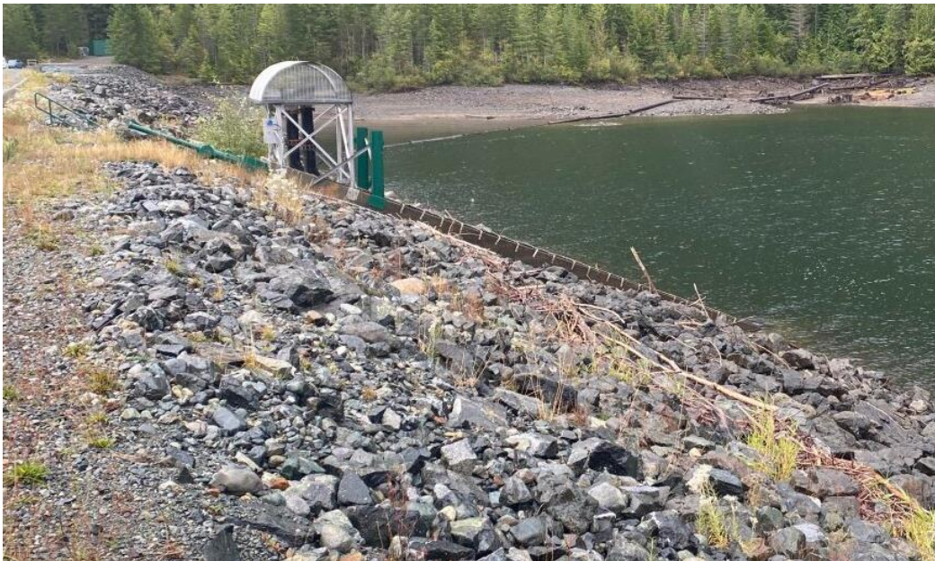
JCR 18: LLO Intake at the Upstream Face of the Dam
