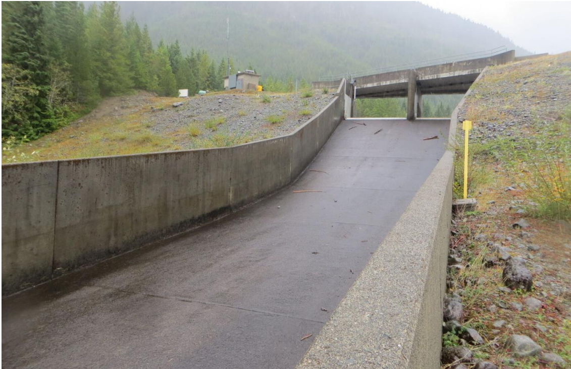
JCR 9: Spillway Chute (looking Upstream)
