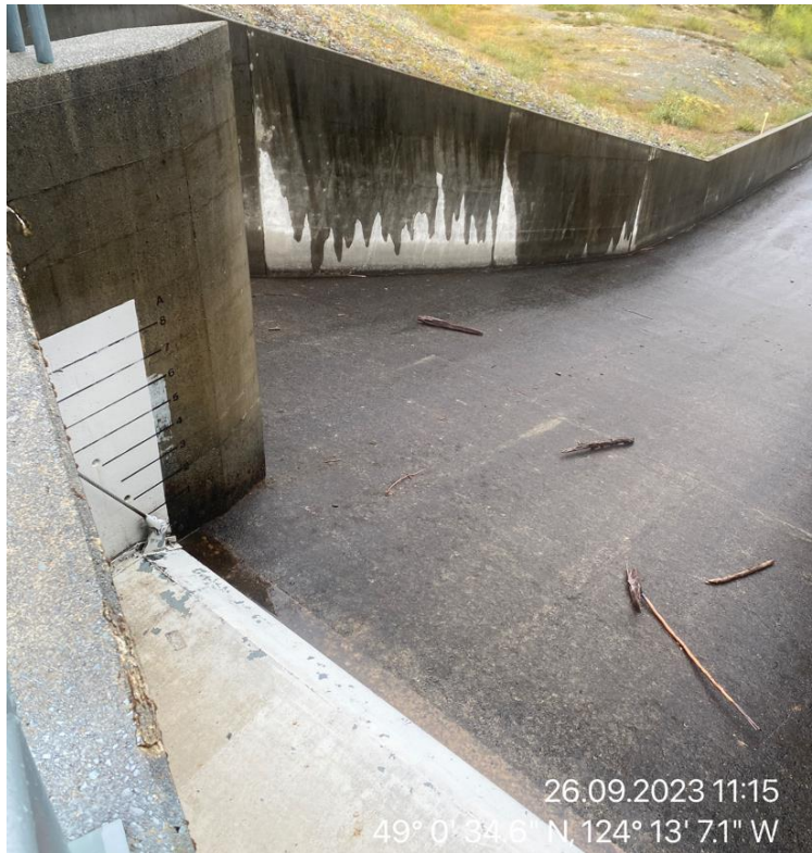
JCR 13: Small Debris Inside Spillway Structure Chute (Looking Downstream)
