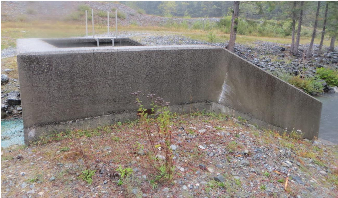
JCR 21: LLO Concrete Structure at Downstream Side (Right Wingwall)
