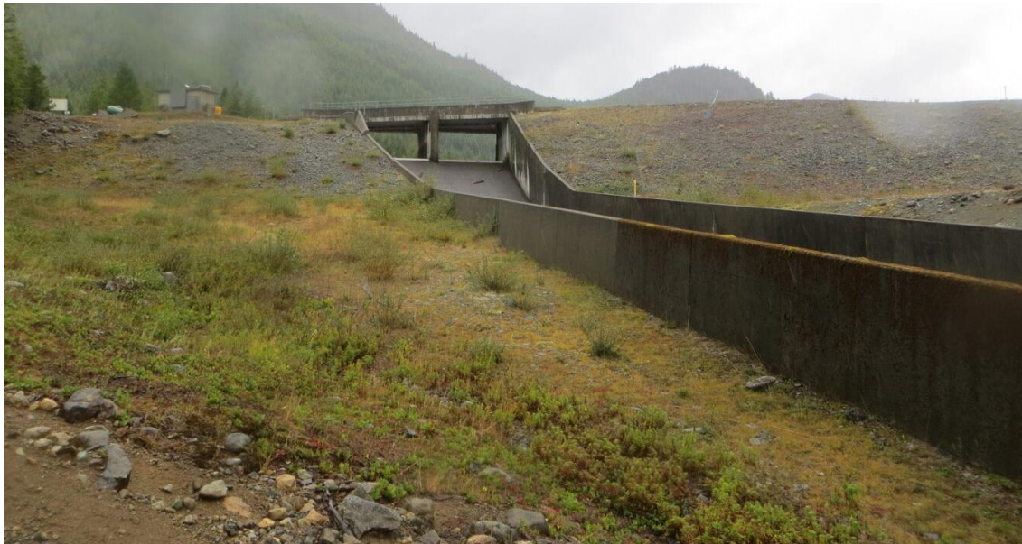
JCR 10: Vegetation near to Right Wall of Spillway Chute
