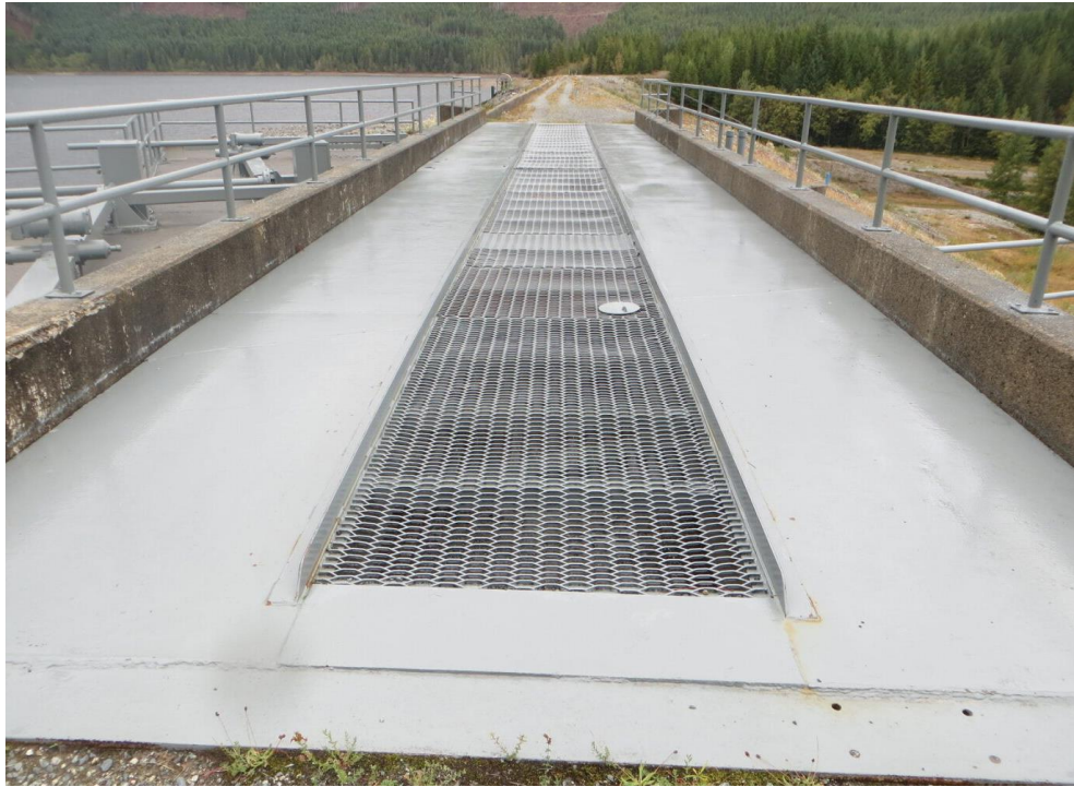
JCR 7: Steel Grating and Angles on Spillway Deck to Prevent Wheel Loading on Grating
