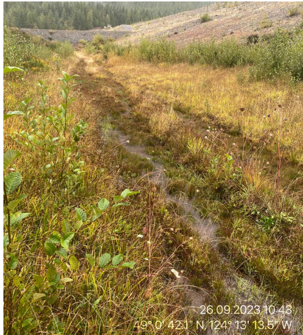
JCR 38: Downstream Toe with Ruts and Seepage
