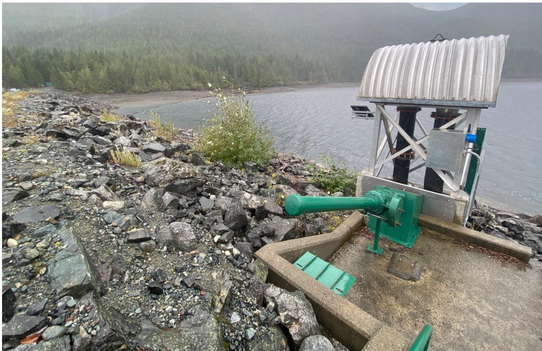
JCR 6: LLO Intake Gate at Upstream Face
