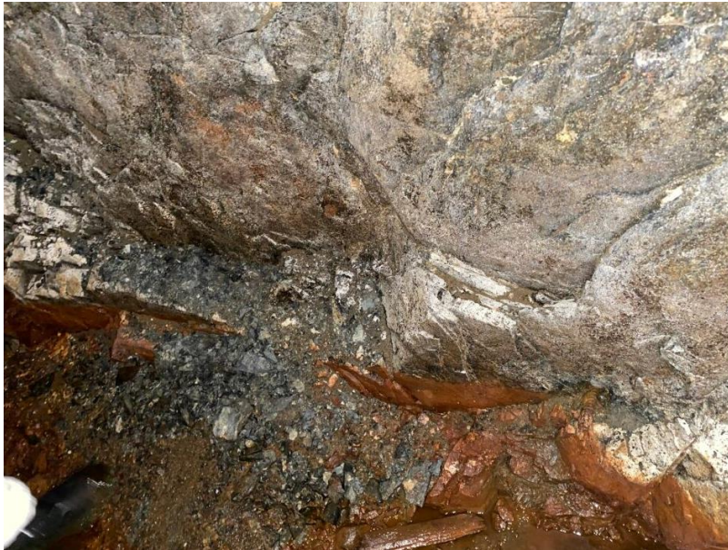
SFK 15: Loose Rocks Observed at the Toe of the Left Wall of the Supply Tunnel, where Local Shear Clay-filled Discontinuity is Found
