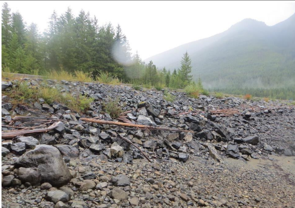
JCR 39: Over-steepened Section in the Upstream Riprap at the left Abutment
