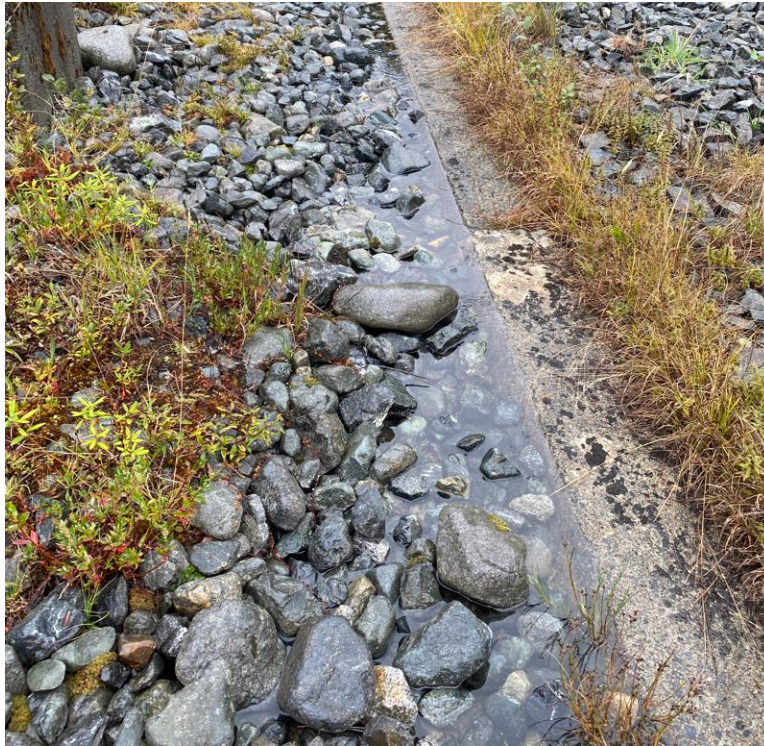
JCR 44: Seepage at Downstream Toe of Auxiliary Spillway
