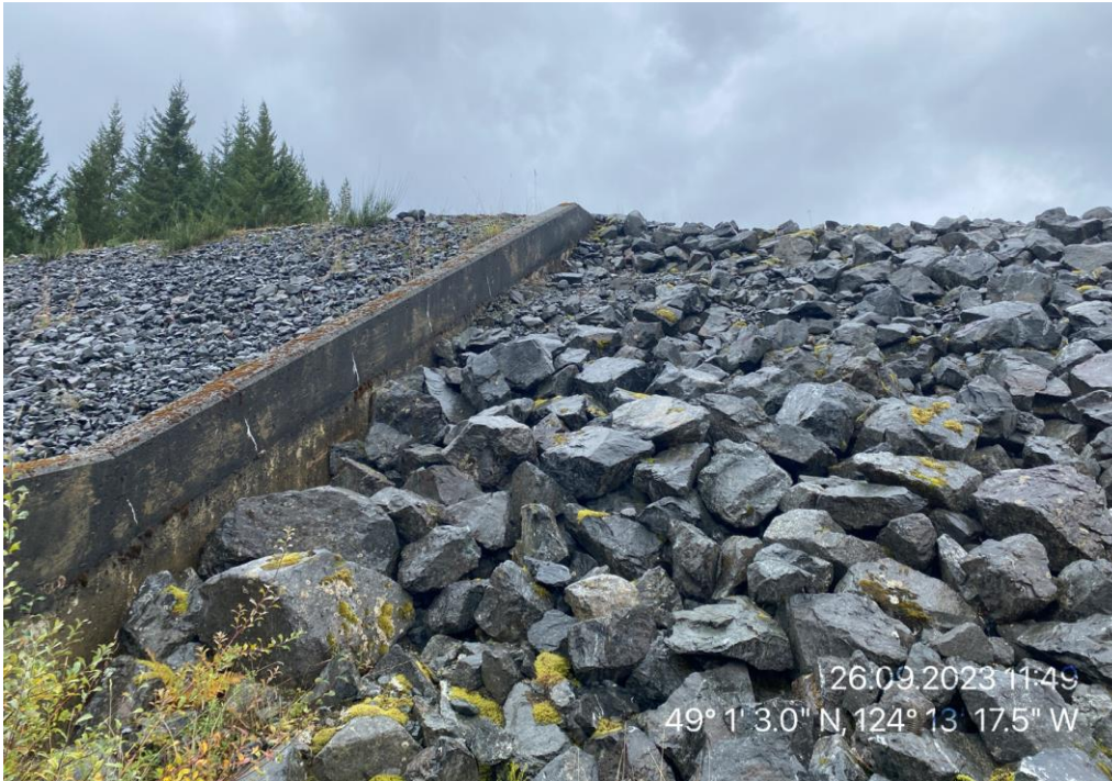
JCR 42: Auxiliary Spillway and Downstream Face of Dam, zone with sparse riprap
