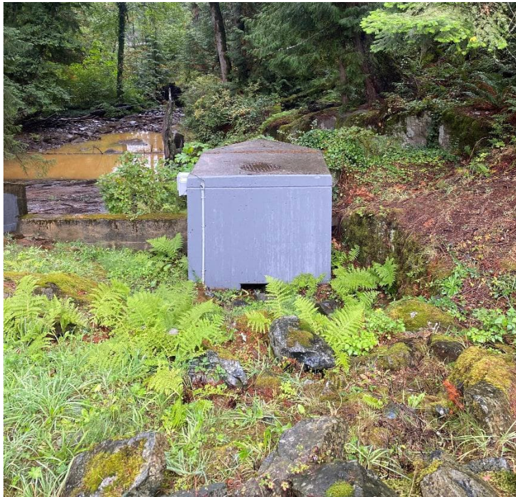
MCR 13: 'V' Notch Weir Housing at Downstream Toe
