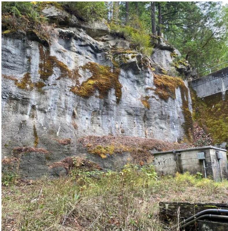
R01 7: Right Abutment Wall Downstream of the Dam (Bedrock, Partially Covered in Shotcrete)
