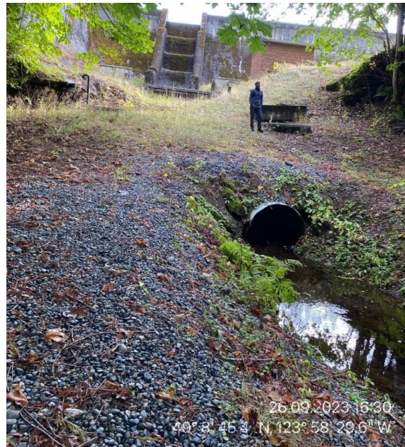
R01 9: Drainage Pipe Downstream of Dam
