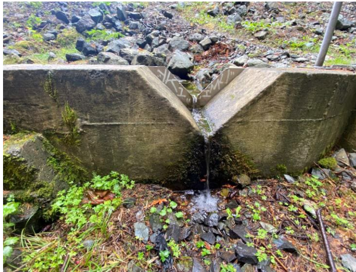
WWL 9: Downstream Seepage Monitoring Weir
