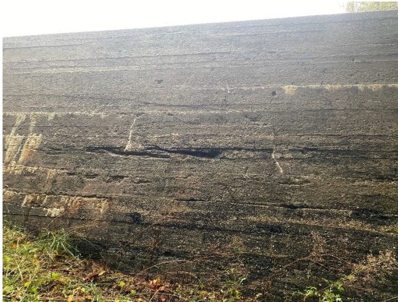
HAW 8: Concrete Deterioration at Downstream Face of the Dam
