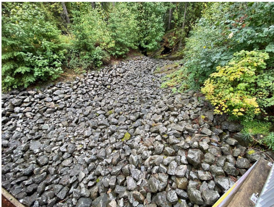
LCR 22: Well-Interlocked Riprap Downstream of Auxiliary Spillway Looking Downstream
