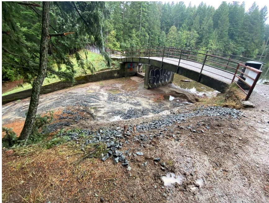
MCR 16: No Fence/Handrail and presence of Cobble cover at Left Side of Spillway
