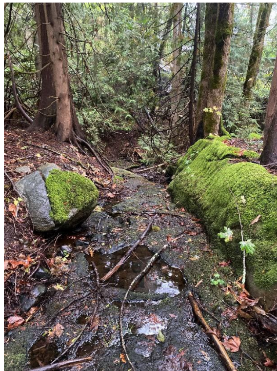
HAW 11: Channel Downstream of Spillway with Minimal Riprap Protection
