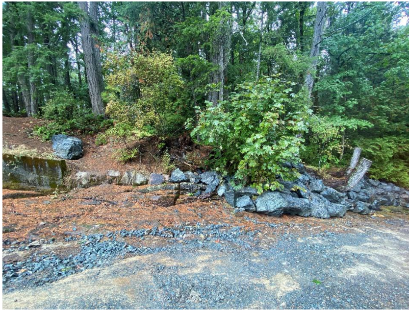
MCR 15: Newly Placed Riprap at the Left Embankment Beyond the Wing Wall
