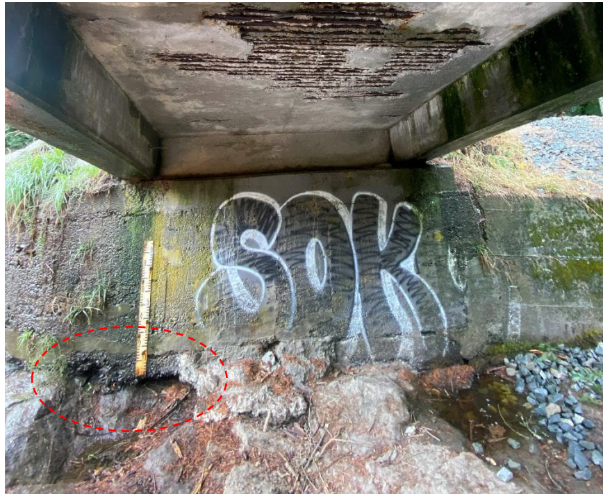
MCR 5: Concrete Erosion at Contact with Rock at Left Abutment of the Spillway Bridge Deck (Left Bay)
