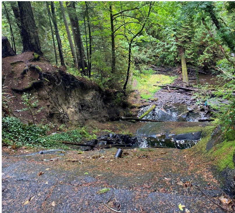
LCR 12: Scoured Rock Channel filled with Debris Downstream of Main Spillway Chute Slab
