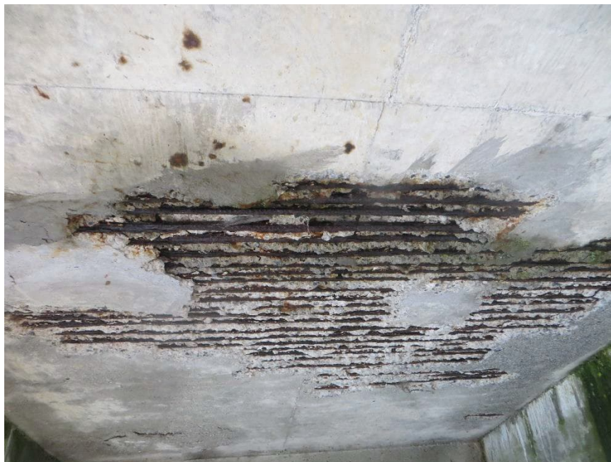
MCR 4: Concrete Deterioration with Exposed Reinforcing Bars Underside of the Spillway Bridge Deck (Left Bay)
