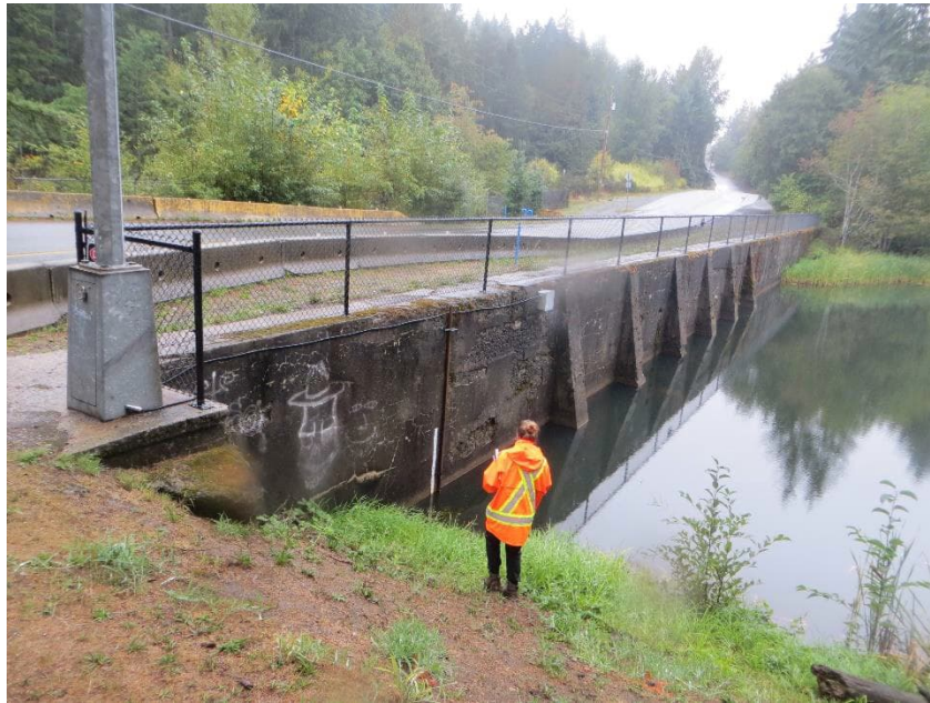
UCR 1: Buttressed Retaining Wall at Upstream Face of the Dam (Looking South)
