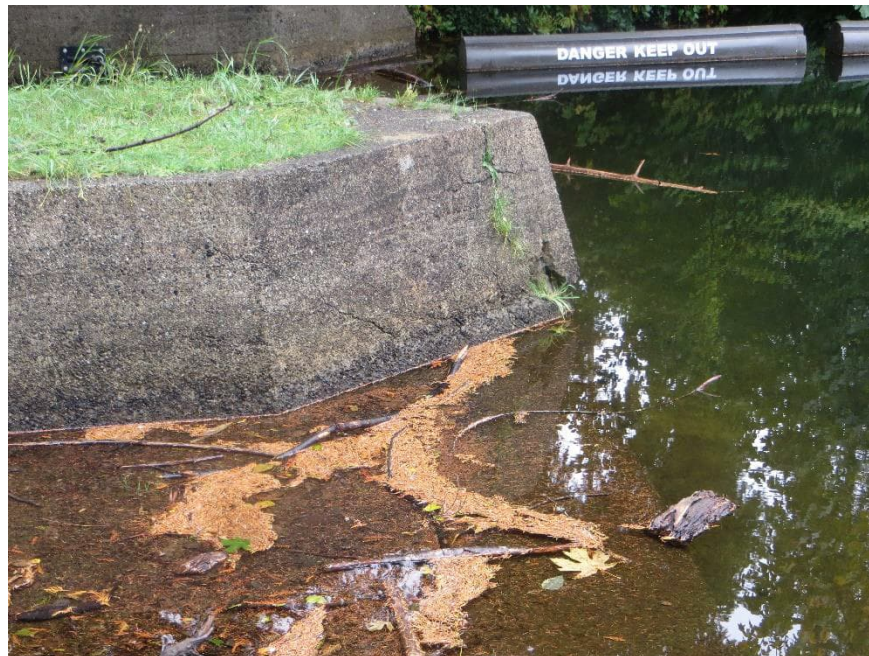
LCR 6: Spillway Centre Pier Nose with Exposed Reinforcing Bar
