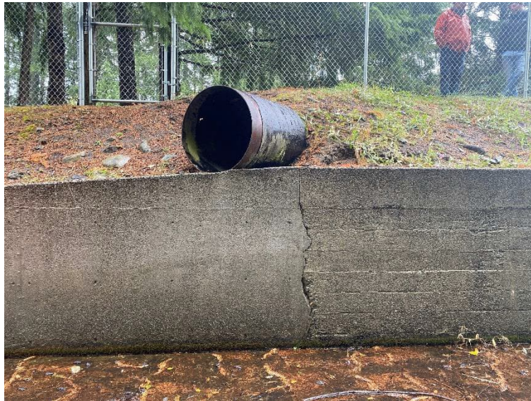
UCR 7: Right Spillway Chute Wall with Crack at Drainage Pipe
