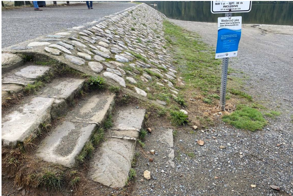
WWL 1: Reservoir, Crest of Main Dam and Upstream Stone Face of Main Dam
