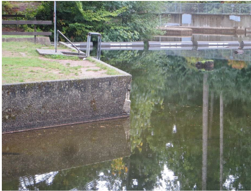
LCR 7: Upstream Retaining Wall for Reservoir Access with Spalling Visible
