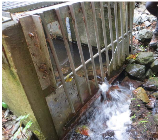
WWL 10: Seepage downstream of the monitoring weir
