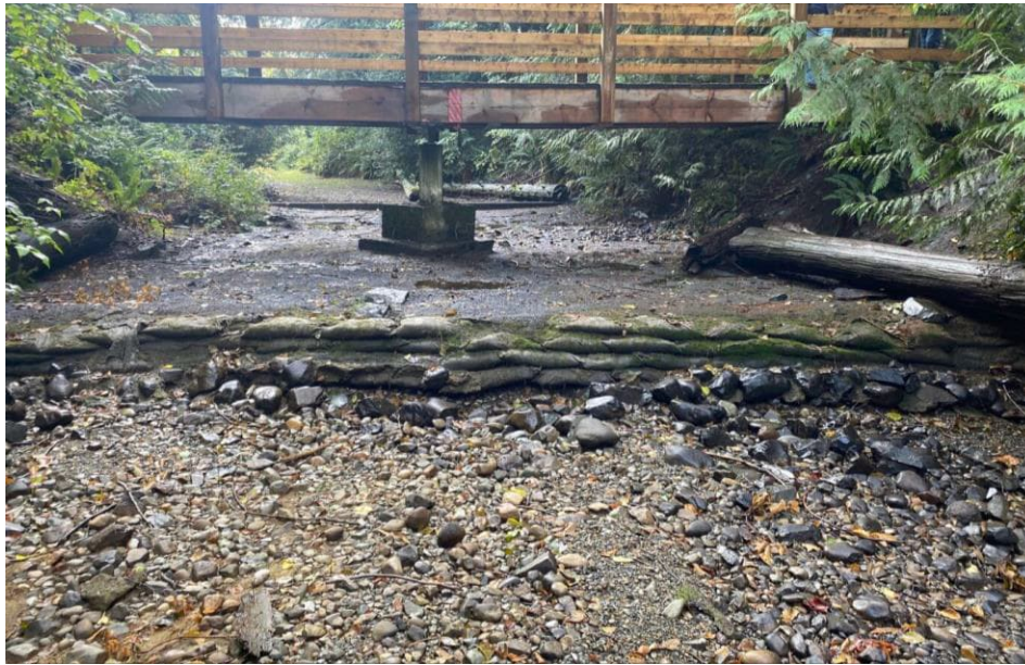
WWL 17: Undermining of the Dam Sacks and Dispersed Riprap at the Downstream Step in the Inlet Channel
