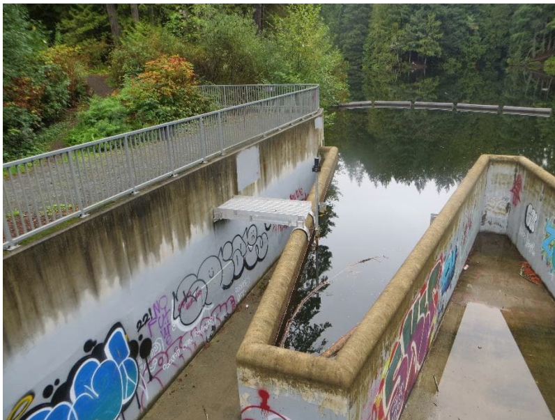
LCR 16: Upstream Side of Auxiliary Spillway Structure and Log Boom Beyond
