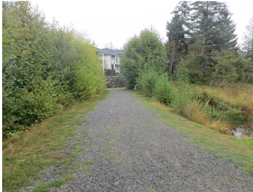
MGC 5: Vegetation on the Downstream and Upstream Face at Right Abutment
