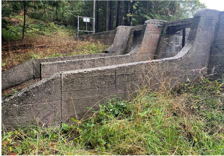
HAW 12: Gap in Joint at Top of Spillway Left Chute Wall
