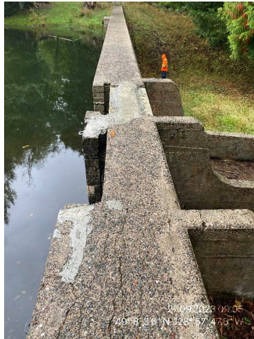
HAW 4: Concrete Deterioration of the Top of the Spillway Bridge
