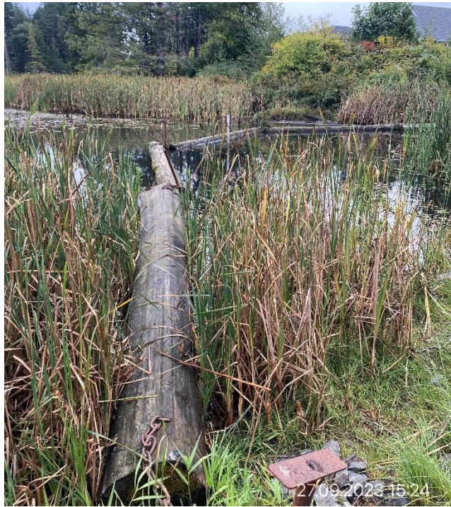
MGC 7: Log Boom at Upstream Side of Spillway Channel
