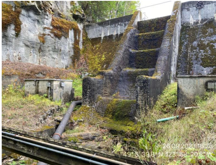
R01 4: Downstream Face and Spillway of the Dam
