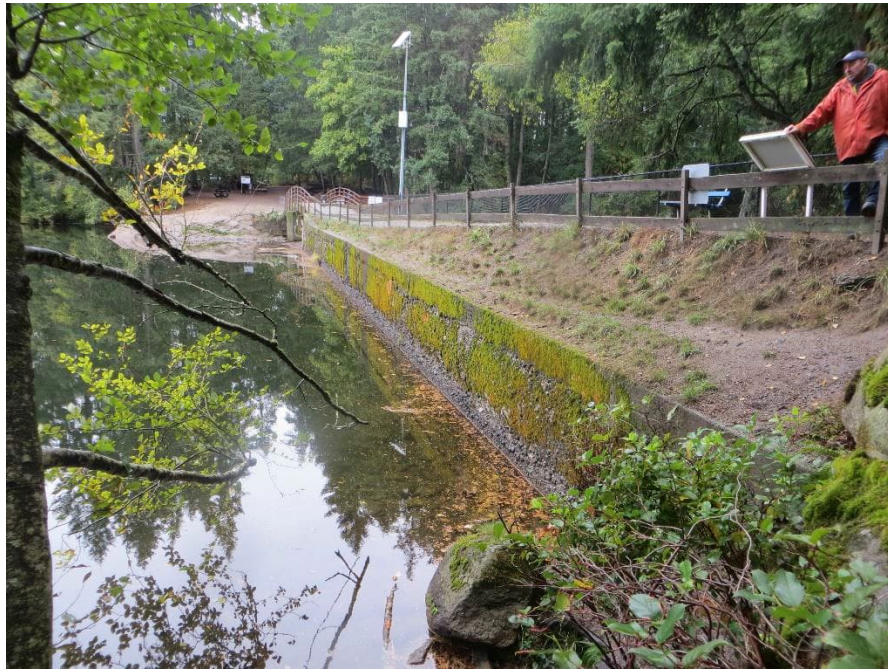
MCR 1: Upstream Wall of the Dam (from Right Abutment)
