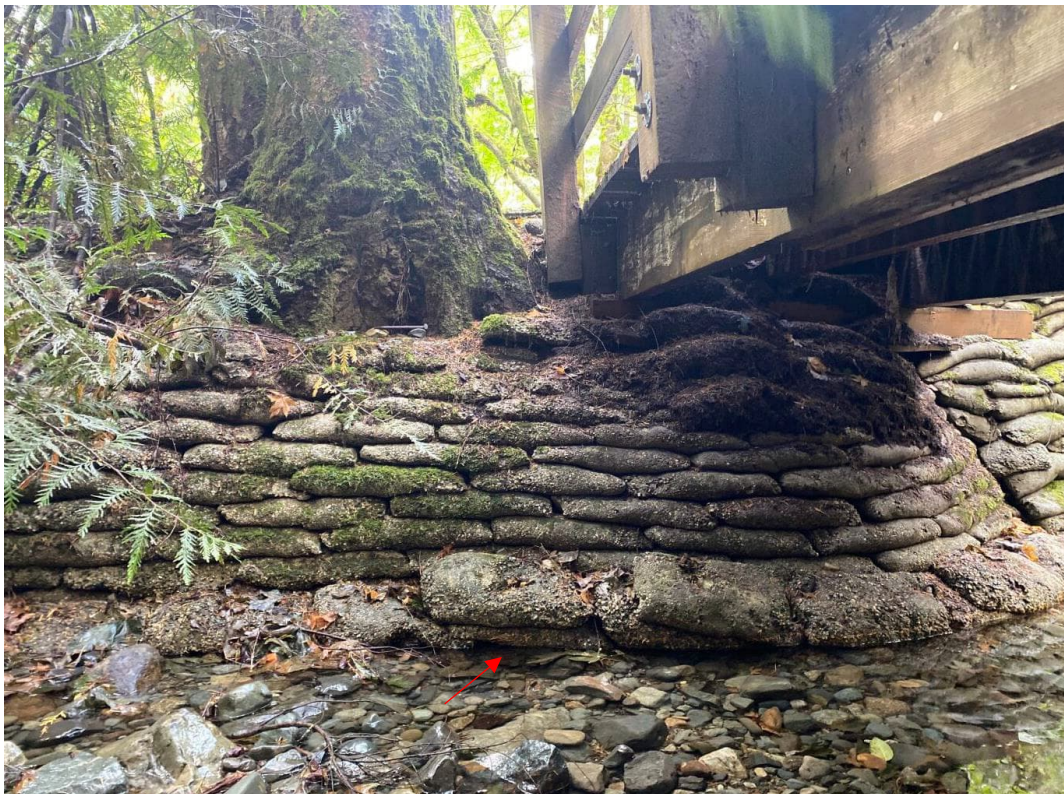
WWL 16: Erosion Damage on Downstream Right Abutment of Bridge (Inlet Channel)
