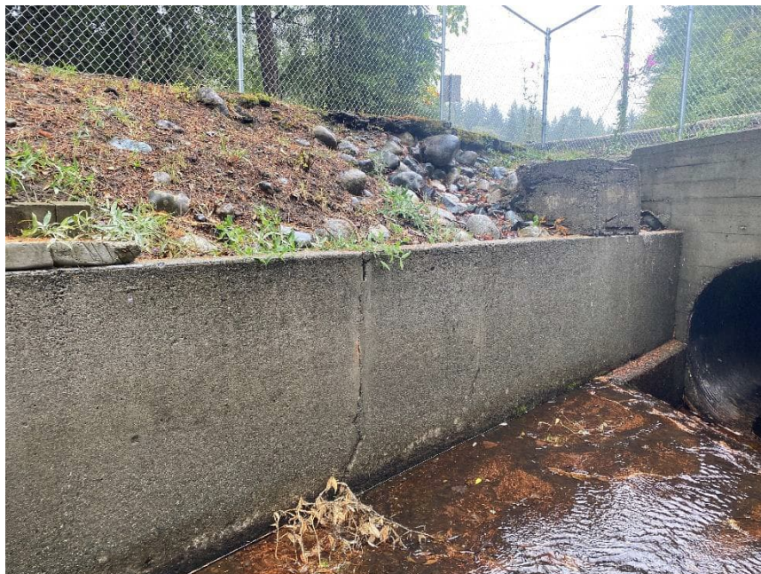
UCR 12: Surface Runoff Erosion Along Wingwall Slopes
