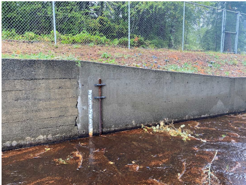
UCR 6: Left Spillway Chute Wall with Crack at Water Gauge
