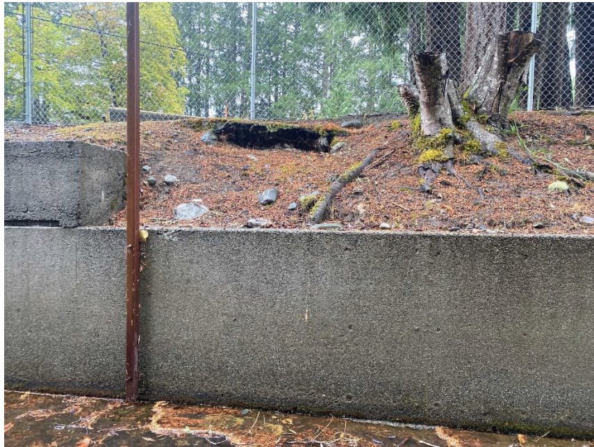
UCR 11: Surface Runoff Erosion Along Wingwall Slopes
