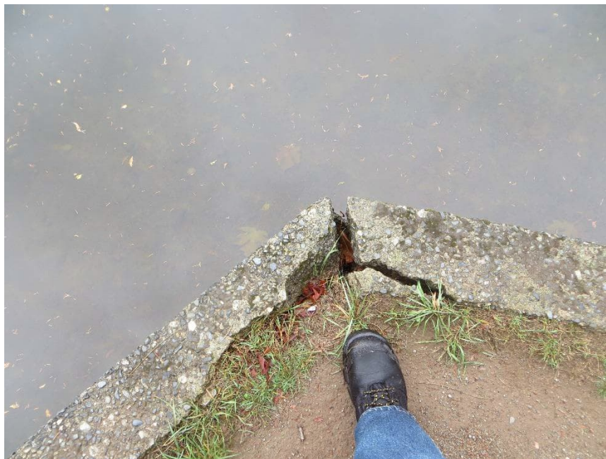
LCR 8: Cracks at Upstream Lower Wall Corner
