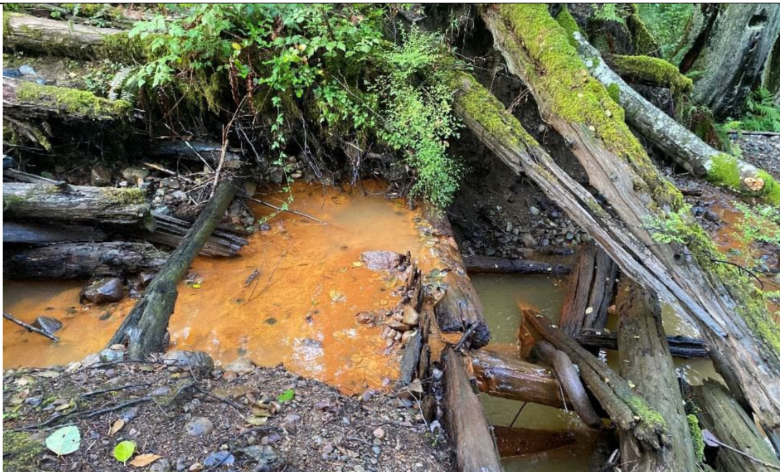
WCL 1: Left Abutment of Dam Showing High Degree of Deterioration
