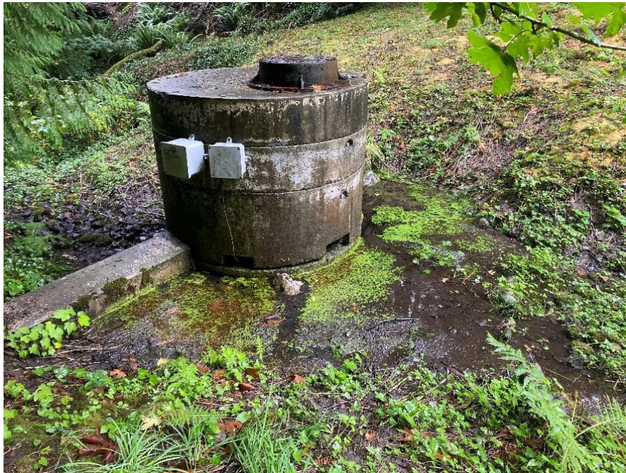
LCR 21: 'V' Notch Weir Housing at Downstream Toe
