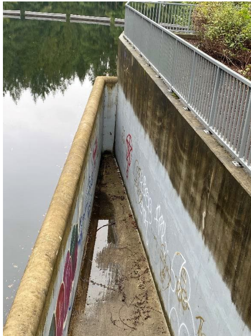
LCR 15: Downstream Face of Auxiliary Spillway (Wet Area at Corner)
