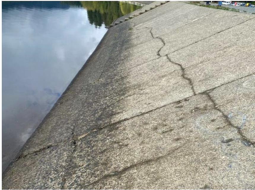
WWL 3: Upstream Concrete Face of Main Dam with Horizontal Cracking
