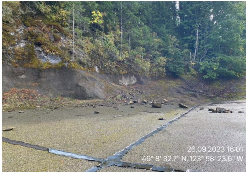
R01 12: Right South End of the Reservoir where Rockslide Debris was Observed
