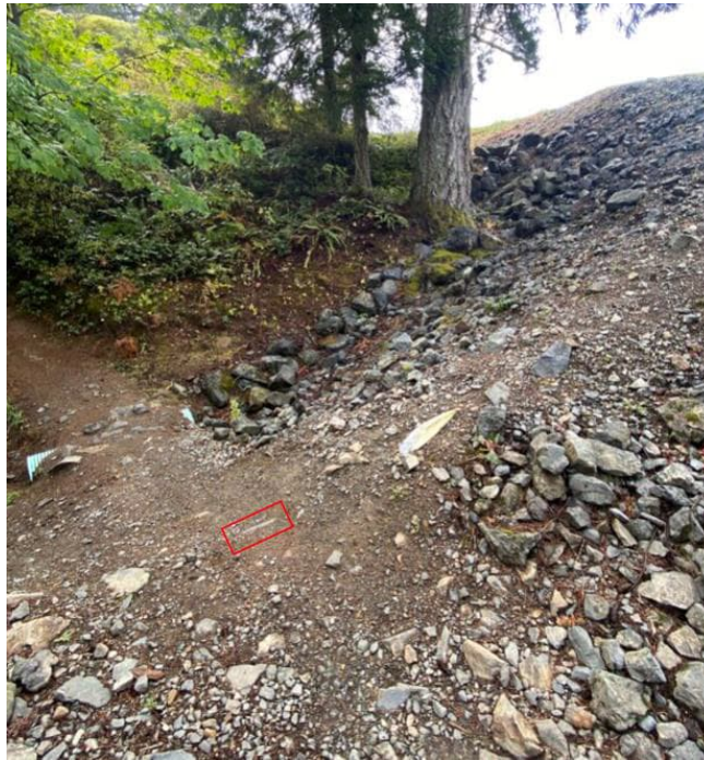
WWL 7: Downstream Face of Main Dam where Part of the Buried Department of Fisheries pipe is Exposed
