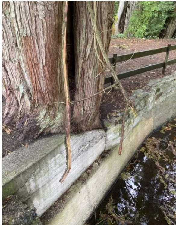
LCR 5: Large Tree Downstream of the spillway Bridge on the Left Abutment
