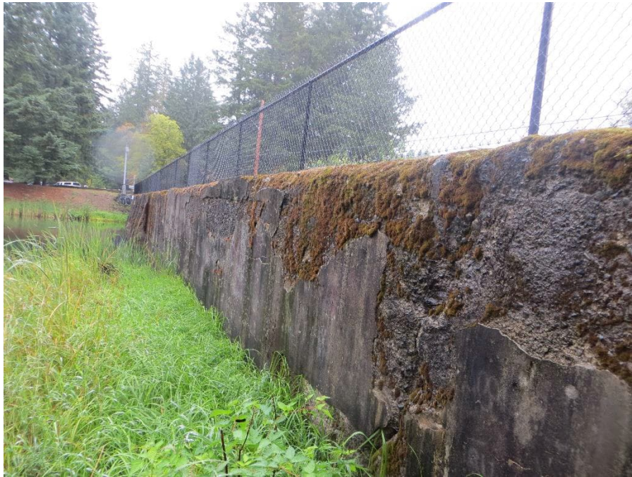
UCR 3: Concrete Deterioration at Right Side of Buttress Wall of the Dam
