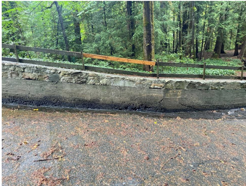
LCR 9: Erosion at the Base of the Spillway Chute Left Concrete Wall
