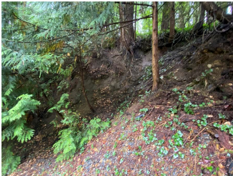
LCR 20: Steep Slope at Downstream Right Abutment with Vegetation, Seepage, and Wet Spots (from Downstream Face, Facing Towards Abutment and Downstream)
