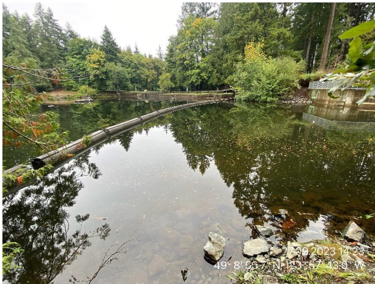
LCR 2: Safety Boom Upstream Side of Auxiliary Spillway
