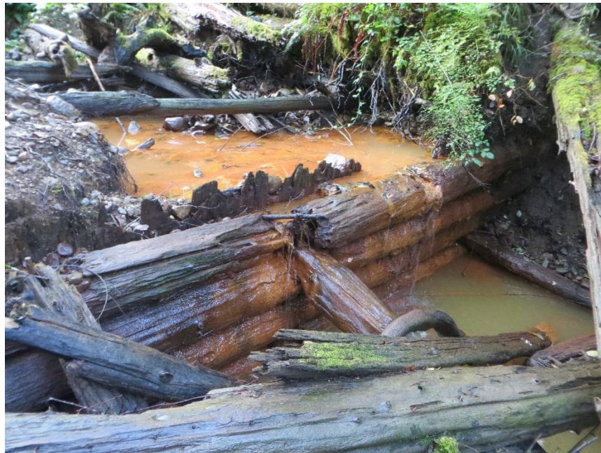
WCL 3: Dam Showing High Degree of Deterioration
