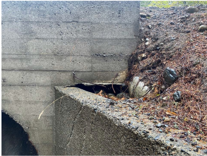
UCR 5: Undermining at the Base of Culvert Headwalls
