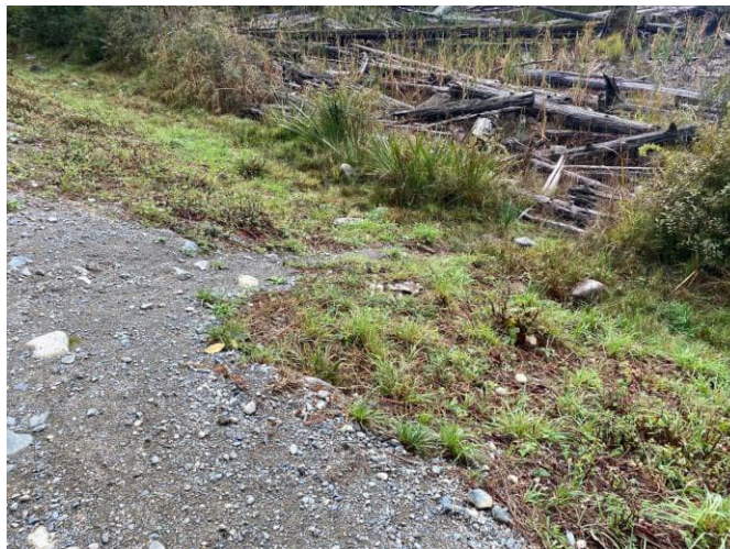
WWL 14: Debris Accumulated at Upstream Toe of Saddle Dam and Light Furrowing on the Upstream Slope
