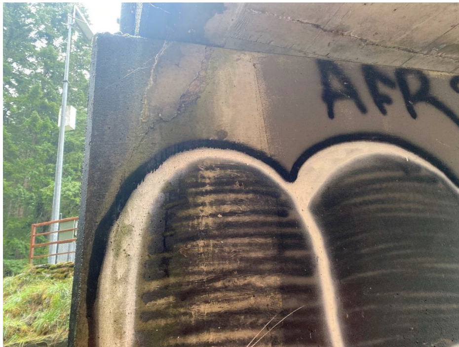
MCR 18: Concrete Crack at Top Corner of Centre Spillway Pier
