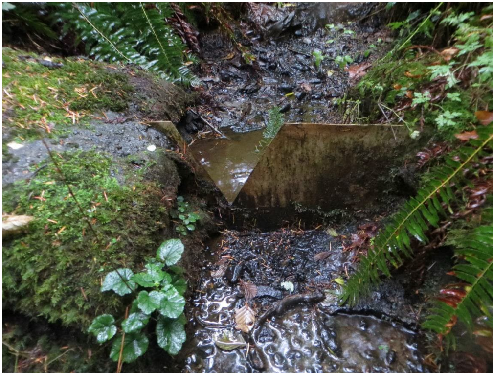
HAW 9: 'V' Notch Weir in Foreground, Stacked Rock Wall Beyond (Looking Upstream)
