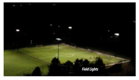
Field lights are typically designed to provide 500 Lux to the field surface as recommended by the Illuminating Engineering Society for tournament level lighting of events; however, if there are to be televised events, which is typical for a stadium, the levels have to be increased to 900 to 1,100 Lux. This higher level can also be achieved using temporary rental lights. This also depends on the level of play (recreational, semi-professional or professional).
