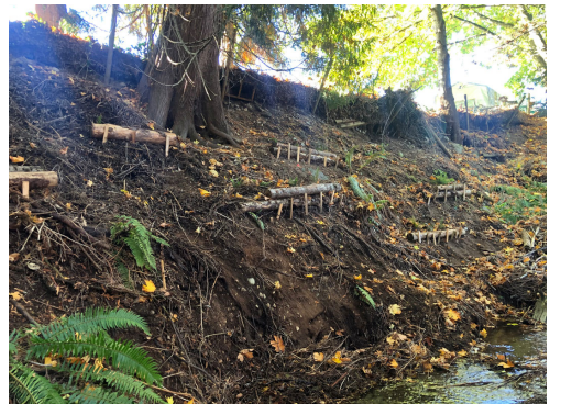
Bank stabilization along the Walley Creek corridor in Morningside Park.
