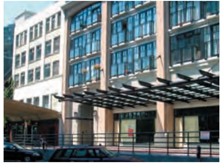
Canopies must be part of the architecture, not an afterthought. They should provide weather protection and not be used as an opportunity for large format signage.
