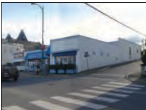
B. SOUTHWEST AT CHAPEL & FRONT
