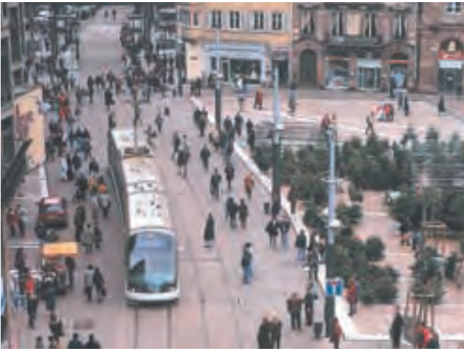
PLACE KLEBER, STRASBOURG Example of a 'shared' right-of-way (Woonerf)
