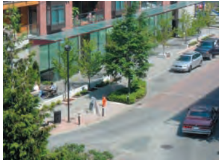
Textured pavement contributes to a more 'livable street'.
