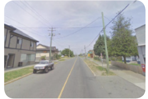
Existing conditions along Haliburton Street.
