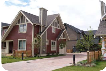
Shared driveways with permeable surfaces.
