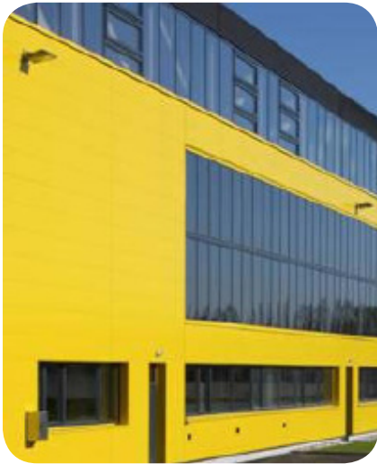
Strategic use of cladding, colors and window and entrance placement can break down the scale of large facades increasing visual interest.
