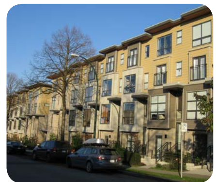
Multiple dwelling developments provide many “eyes on the street”.
