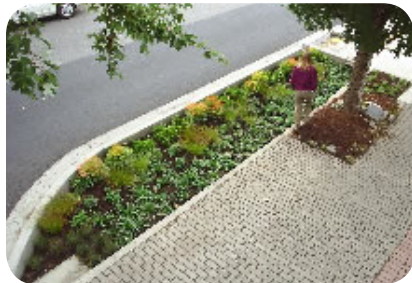
Corner bulges reduce crossing widths and provide opportunities for indigenous, drought tolerant plants and water infiltration.
