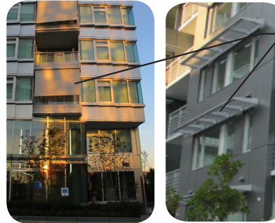
Incorporate shading devices into the building design.
