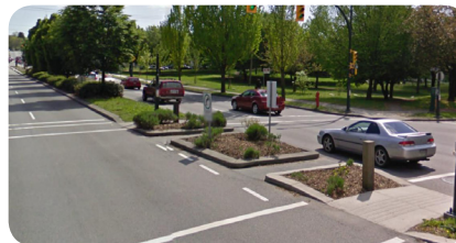
Pedestrian and cycle median crossings maintain traffic flow
