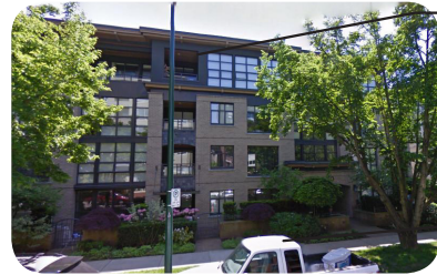
The 4th floor is expressed with darker materials, a floor level cornice line and a larger, divided glazing pattern. Individual gardens continue the pattern of green front setbacks.
