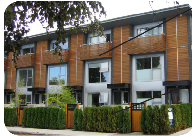
A simple combination of natural wood with industrial materials is recommended. Individual units are identifiable within the overall street elevation.
