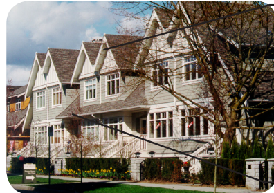
Extensive trim and detailing and large window proportions distinguish this new development.
