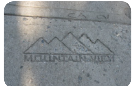
Stamped neighbourhood motifs can be integrated into any new concrete sidewalk surface.
