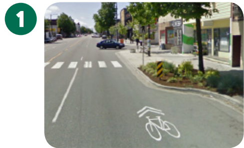
Pedestrian crossings and designated bicycle lanes
