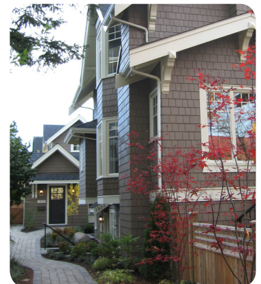
Coach houses can provide valuable living space with minimum impact on neighbour's privacy and private outdoor space.
