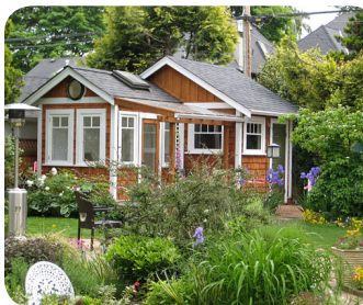
Gabled roofs, wood cladding, generous trim proportions, simple building forms and careful landscaping allow coach houses to fit into existing neighbourhoods and complement traditional and heritage style properties. Photo Credit: smallworks.ca.
