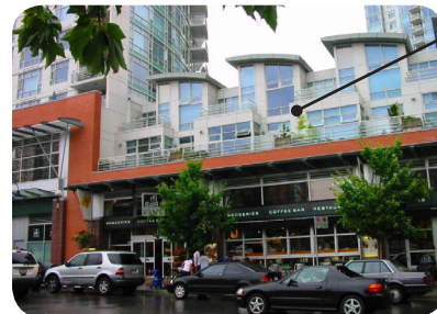
Low rise forms with varying roof heights and changes in plane contribute to the streetscape.
