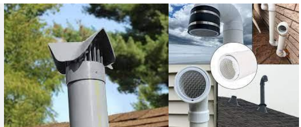
Illustration F Pipe termination protection
