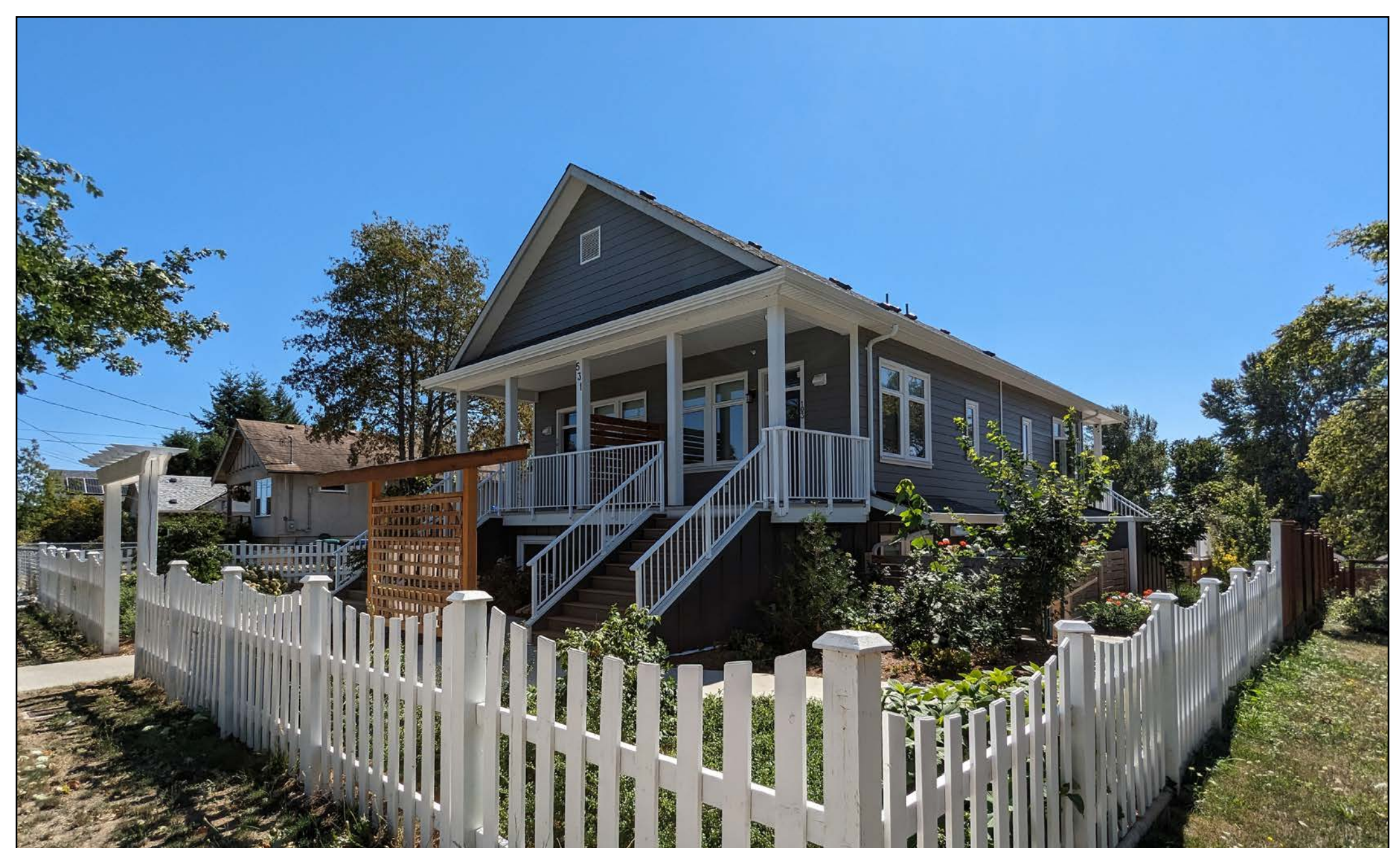
Image [above]: Fourplex home in Nanaimo.
