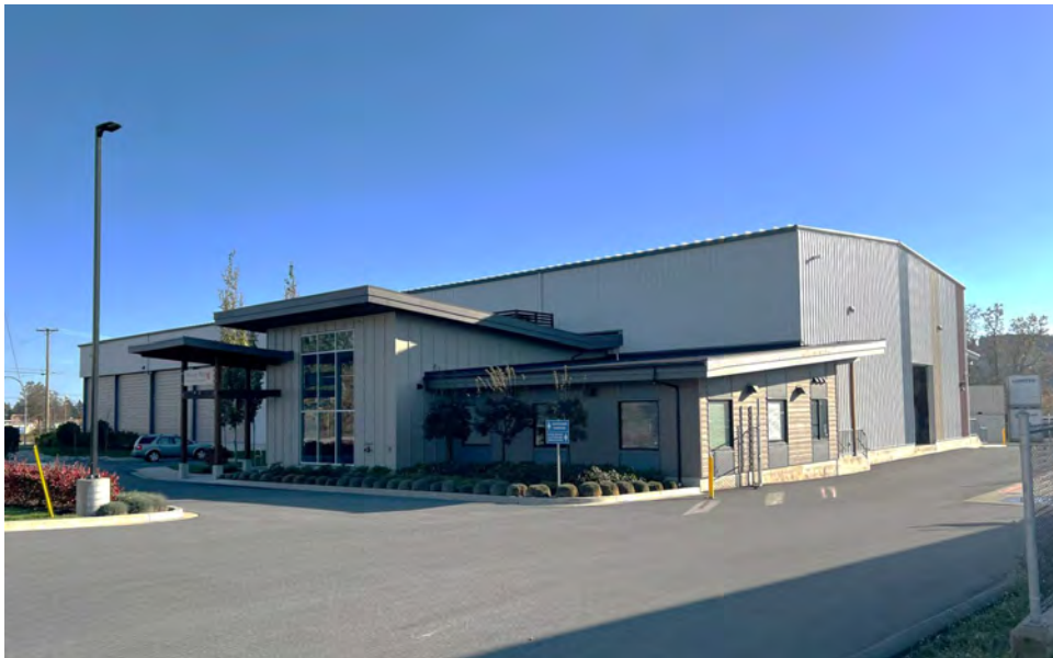
Example of Building in Area: Pre-engineered building with architectural storefront on street
