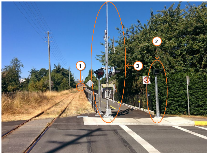
Figure 10: Components of a Grade Crossing Requiring Upgrades to Signals and Gates
