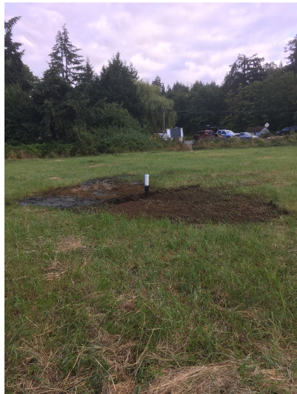
Photo 5. Completed well installation.
