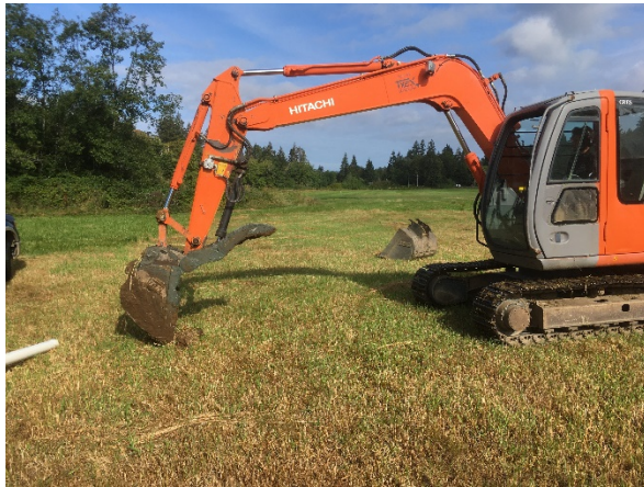
Photo 2. Stripping vegetation and surface organics during well installation.
