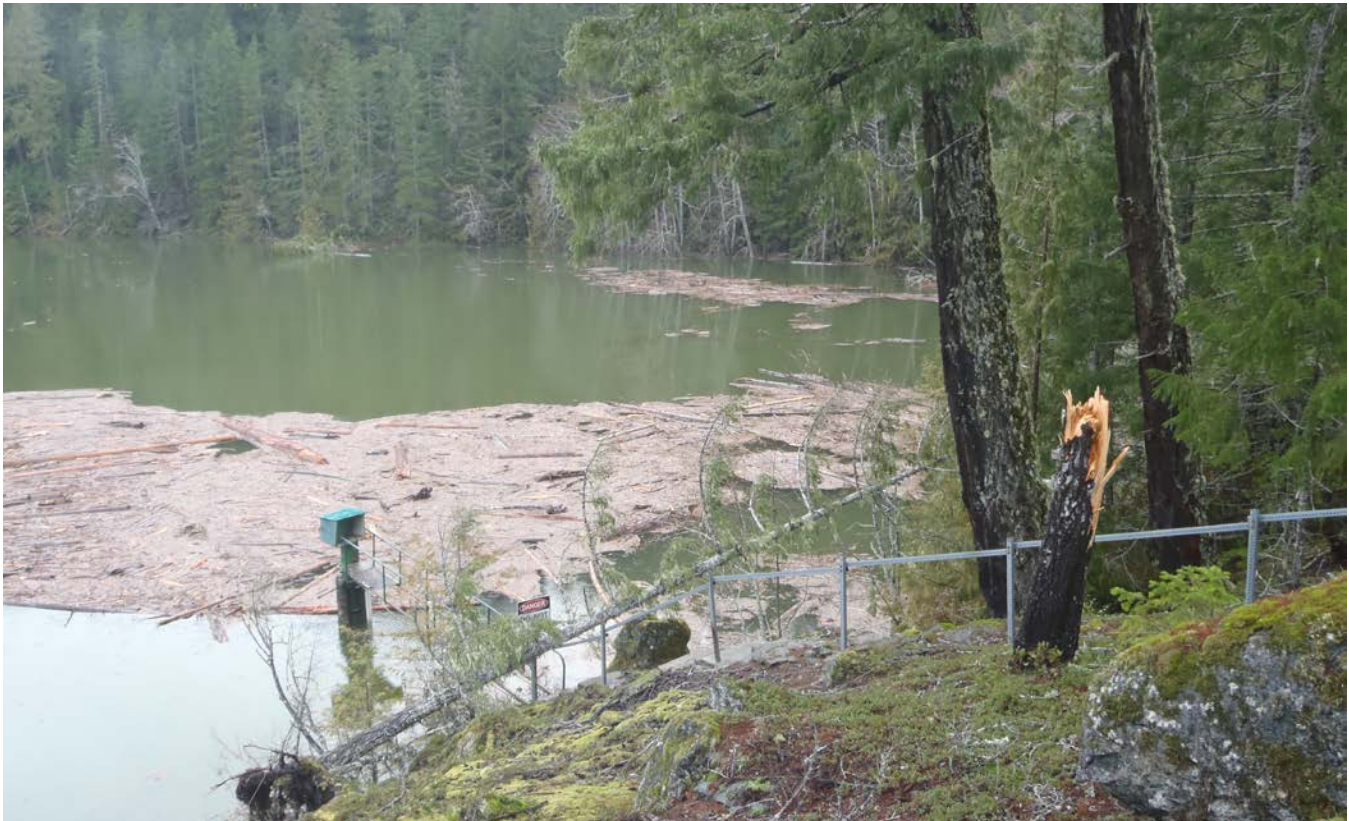
Figure 6-1: Example of multi-hazard interactions that threatened the water intake at South Fork Dam. Source: City of Nanaimo.
